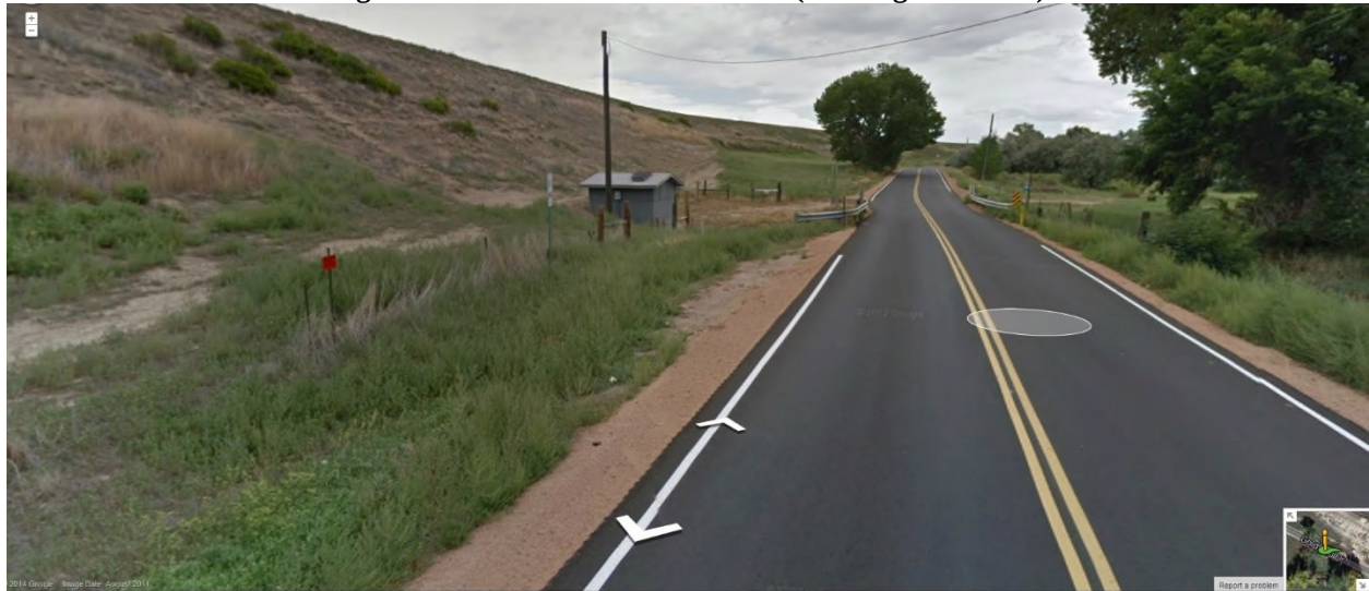
Figure 7-5 Big Johnson Reservoir Embankment (Looking Southeast)
