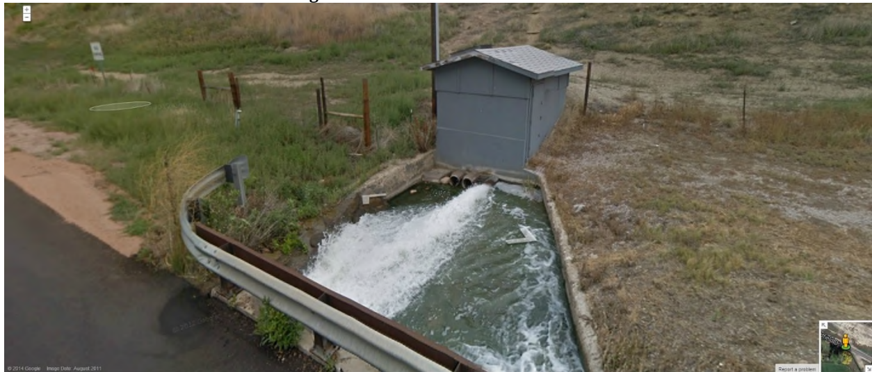
Figure 7-6 Big Johnson Reservoir Outlet Works
