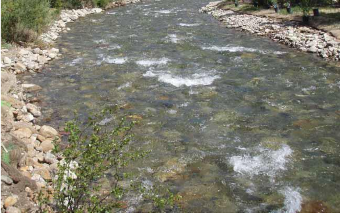
Figure 4: An example of an area where a pool was constructed but had filled in after erosion and deposition occurred during the 2014 flood
