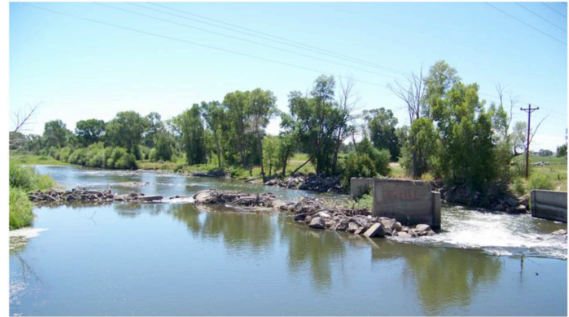
Figure 4. McDonald Ditch Diversion (Looking Downstream)
