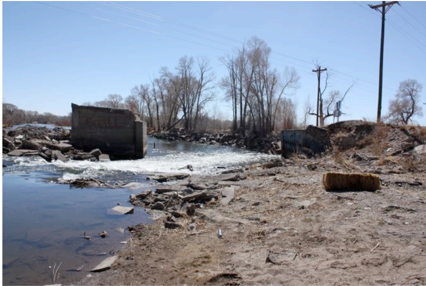
Figure 28. Power Poles Near the McDonald Ditch Diversion
