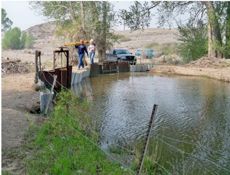
Figure 9. Silva Ditch Headgate (Right)
