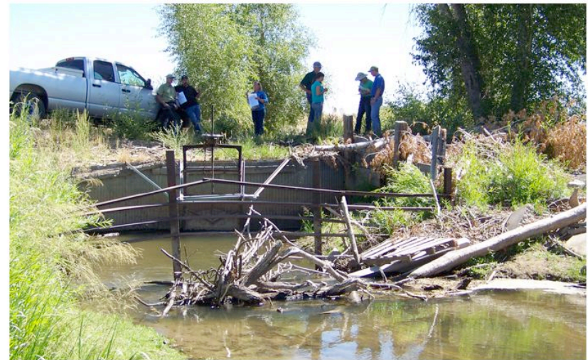
Figure 5. McDonald Ditch Headgate
