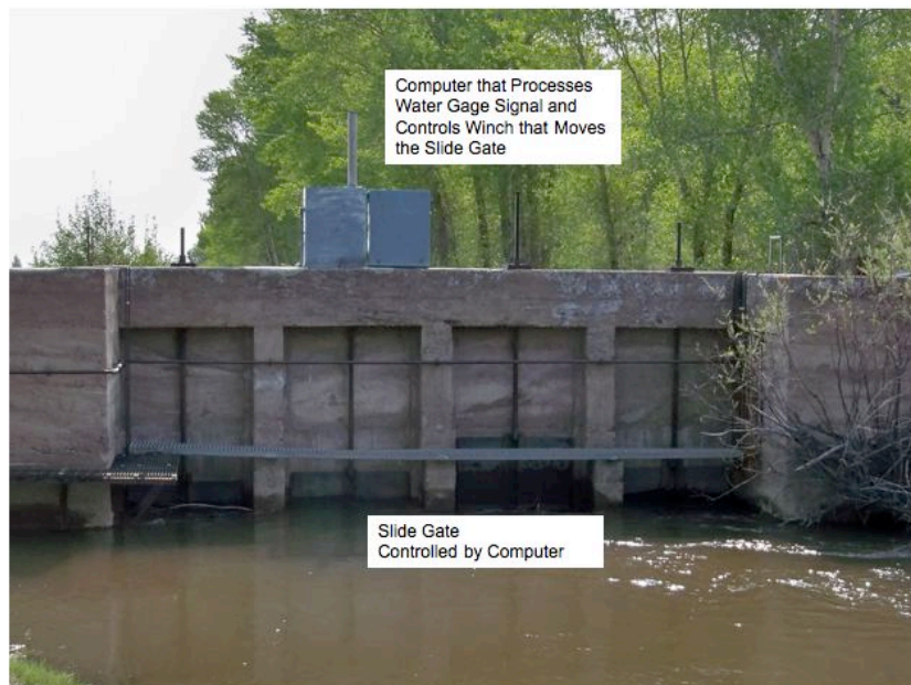
Figure 24. Automated Gate at the Prairie Ditch Headgate.
