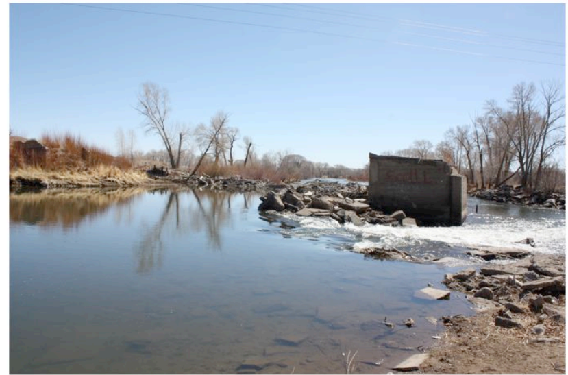
Figure 30. Old Sevenmile Plaza Bridge Pier; Currently Part of the McDonald Ditch Diversion
