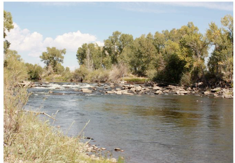
Figure 6. Prairie Ditch Diversion (Looking Upstream)
