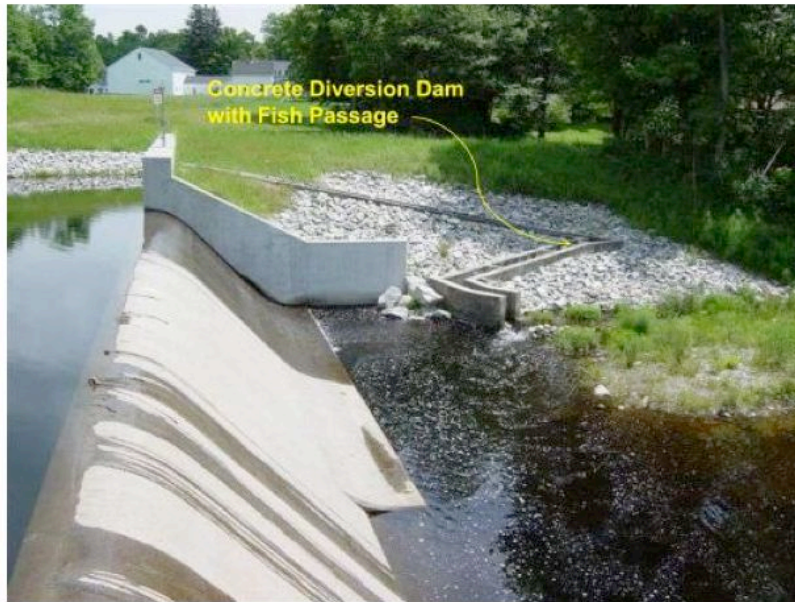
Figure 16. Example of Concrete Diversion Dam
