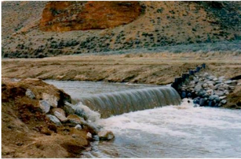
Figure 18. Example Grouted Rock Diversion Dam
