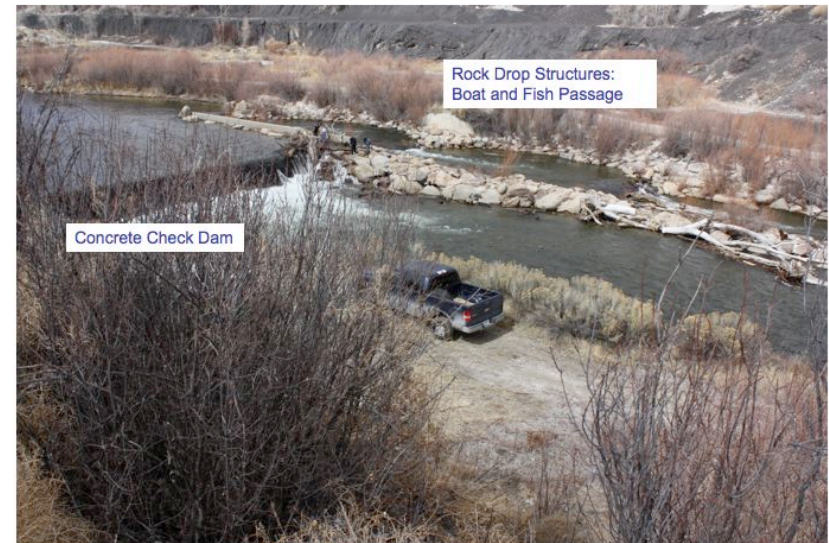
Figure 20. Example Hybrid Concrete and Grouted Rock Diversion Dam (Near Salida, CO on the Arkansas River)
