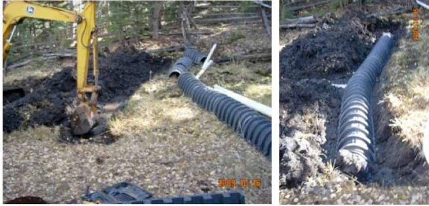
Figure 22. Example of Pipeline Installation
