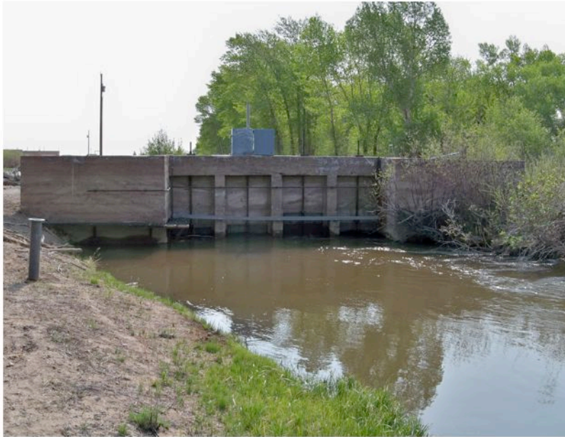
Figure 7. Prairie Ditch Headgate
