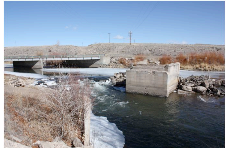
Figure 27. Sevenmile Plaza Bridge and McDonald Ditch Diversion
