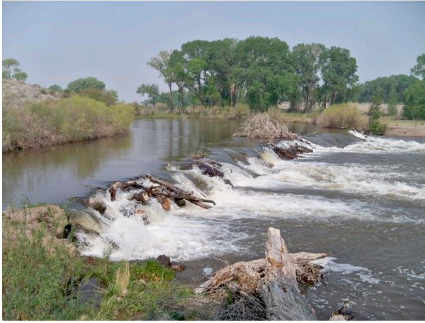
Figure 8. Silva and Atencio 2 Ditches Diversion
