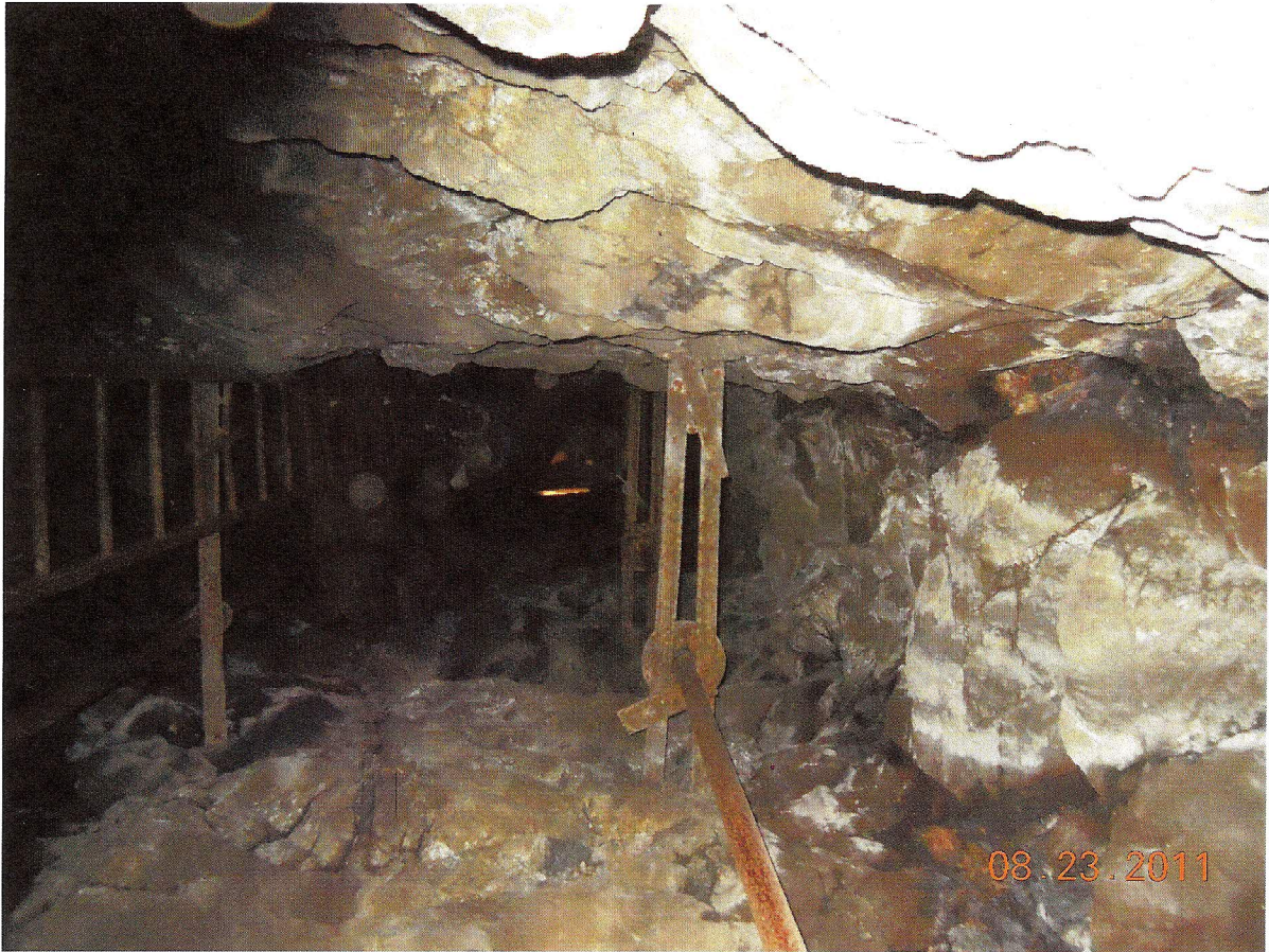
View looking upward into the vertical rockcut shaft for valve stems.
