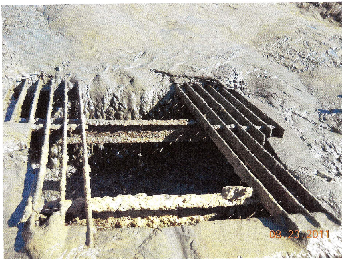
View of trashrack looking upstream from the upstream slope.
