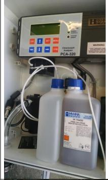
A Hanna Instruments Chlorine analyzer was installed to assist with monitoring.
