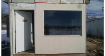
A new insulated window was installed in the south wall. Painting will be completed in the Spring, 2015.
