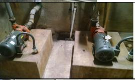
Existing pumps are designed to come on when pressure drops below to 24 psi and turns off at 39 psi.
