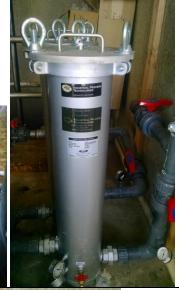
Graver Filter system installed with both a pre-filter (5MC3-30inch) and a final filter (5MC3-30-222-30inch). The filter cartridges were installed in early December. With the low turbidity in the water, they are expected to last longer than others. The filters can process 50 gpm into the pressure tank.
