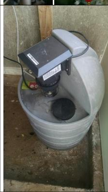
A Stenner pump and 30 gallon chlorine reservoir was installed to automate chlorination.
