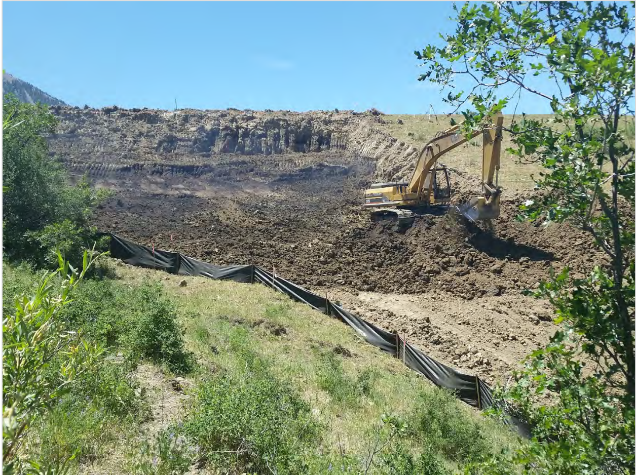
Photograph 9: excavated area at end of day July 2, showing silt fence and general progress of the excavation
