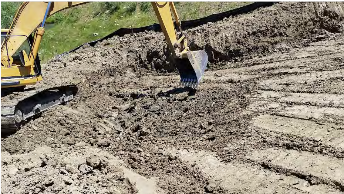
Photograph 13 showing excavation nearly complete at the toe of the dam
