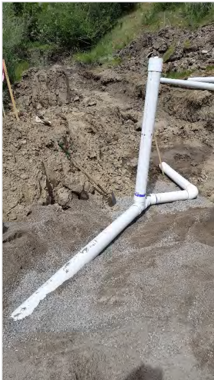
Photograph 17, left, showing the placement of the toe drain pipe at the northeast corner, note aggregate media under pipe.
