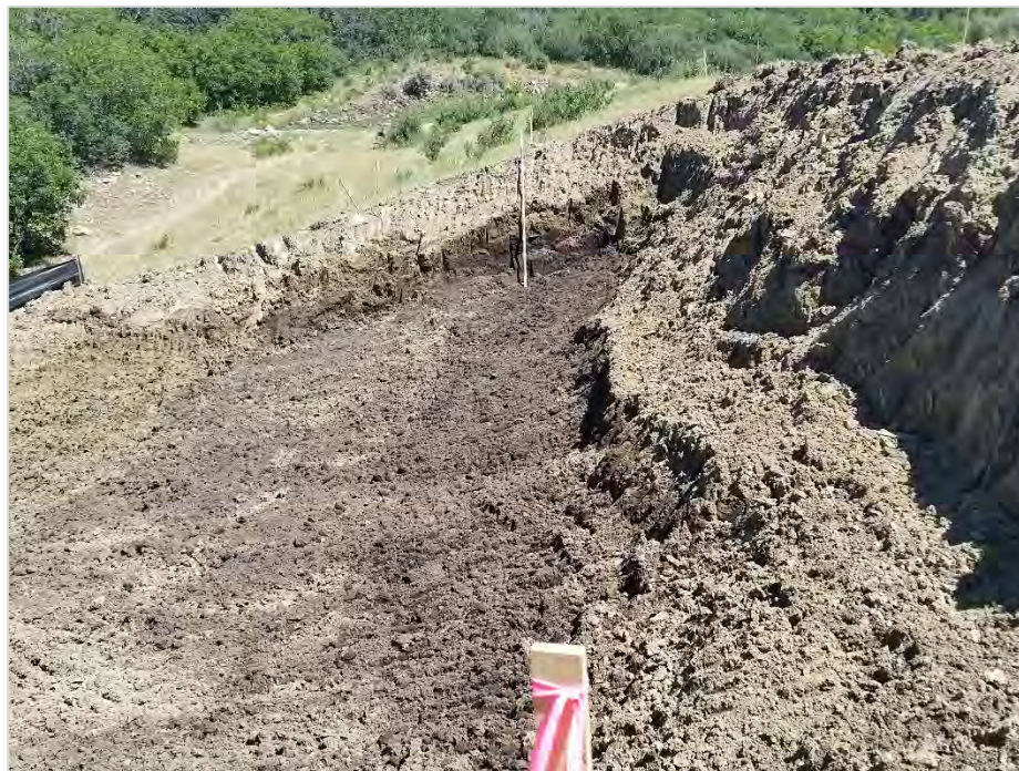
Photograph 6: Shows excavation looking south and the organic material at the base of the cut and the large organic mass extending beyond the planned excavation limits.
