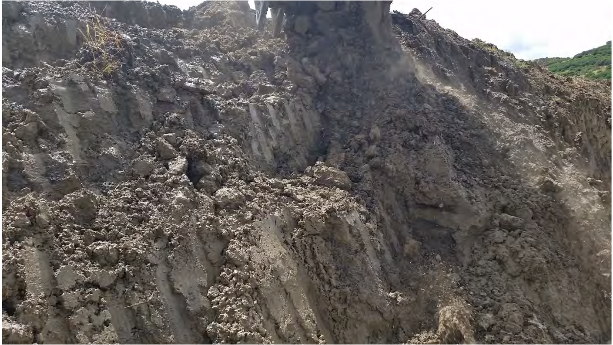
Photograph 27 showing excavation of 1 foot benches in the western face of the excavation.
