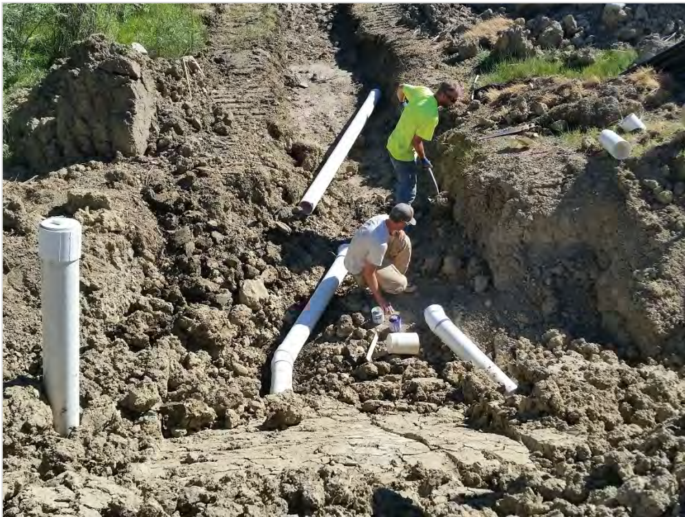
Photograph 22 shows the installment of the outfall portion of the toe drain.
