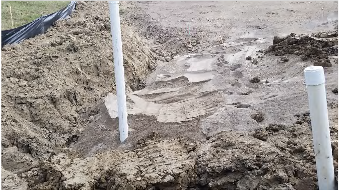
Photograph 19 showing the placement of the filter sand above the toe drain.
