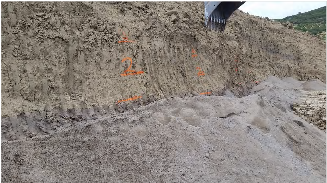
Photograph 24 showing the placement of the sand blanket which will extend to a height of two feet above the organic horizon. The desired height is marked with paint on the excavation wall.
