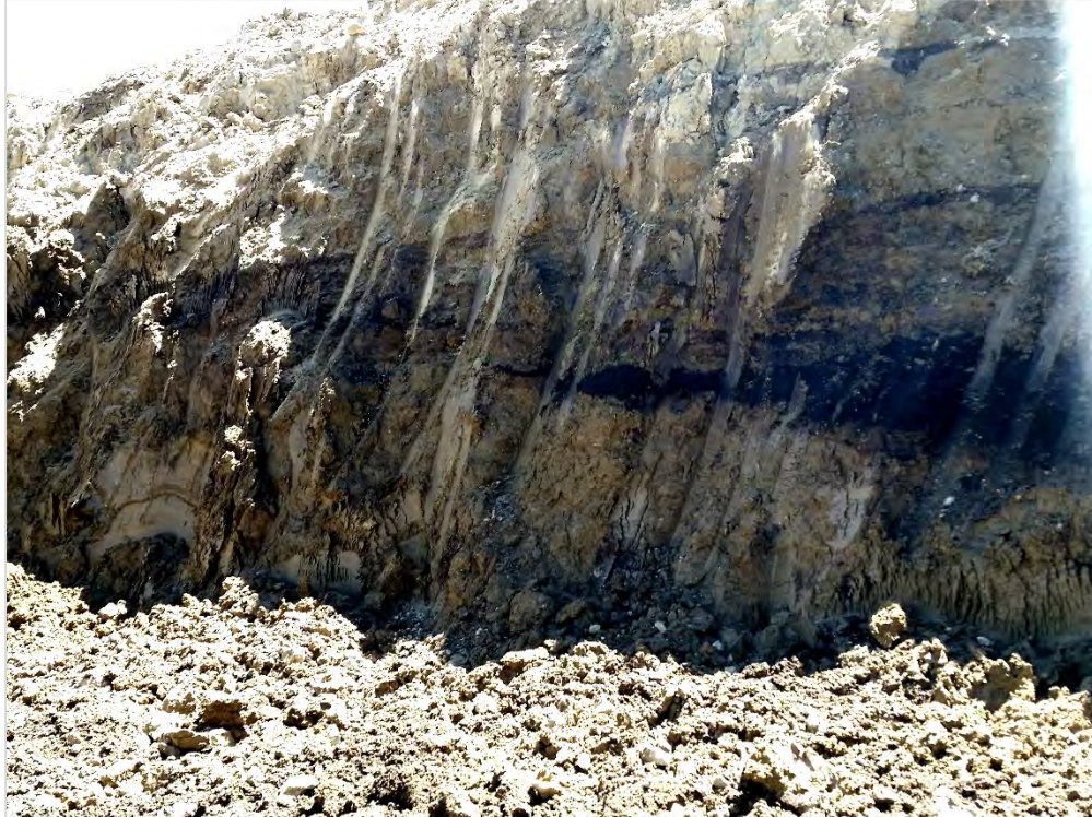
Photograph 3: Shows layered nature of the organic material in the side slopes of the excavated area
