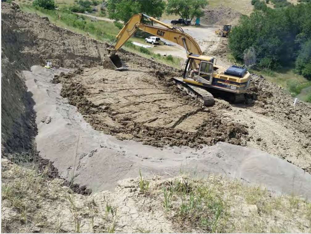
Photograph 21 showing the general methodology of filter sand placement and embankment soil.
