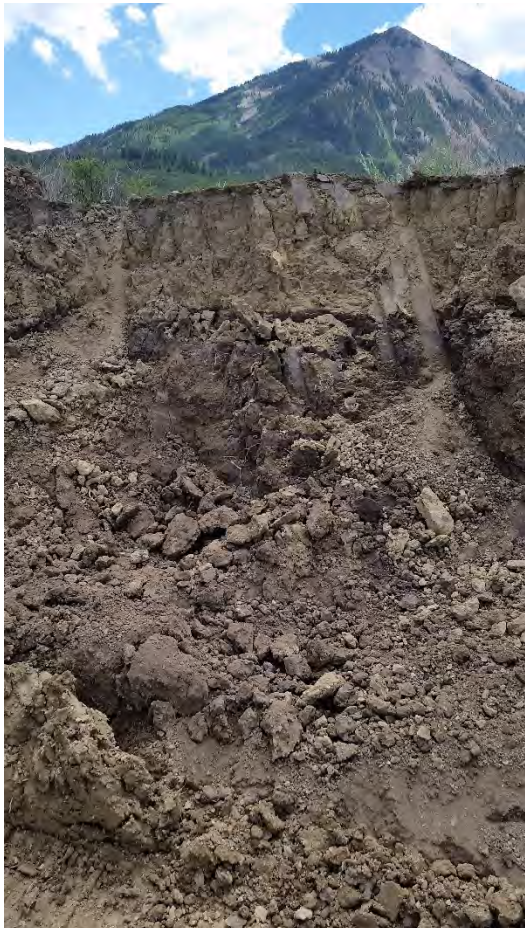
Photograph 27 showing excavation of 1 foot benches in the western face of the excavation.
