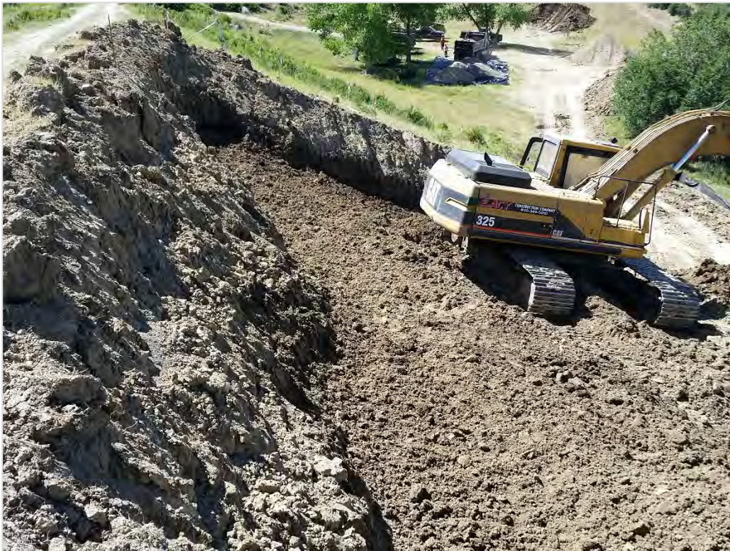
Photograph 3: Shows layered nature of the organic material in the side slopes of the excavated area
