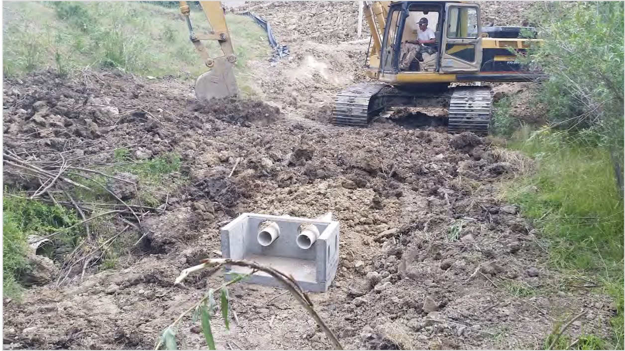
Photograph 23 shows the placement of the concrete outfall structure.
