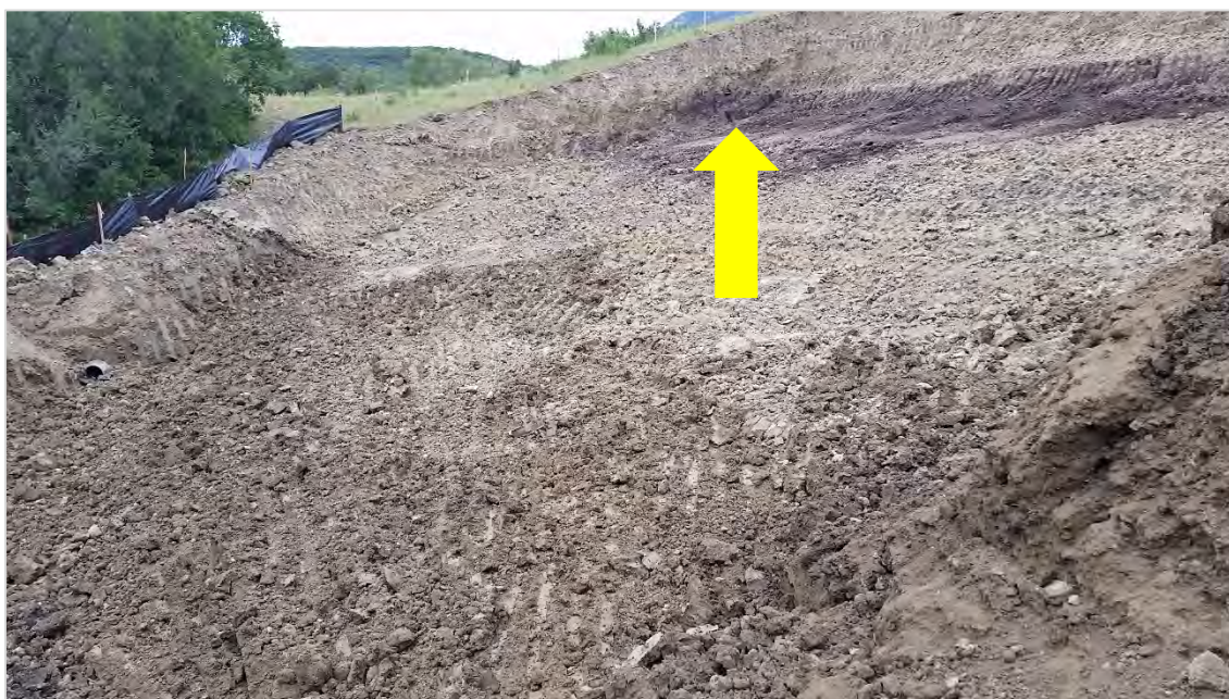
Photograph 15 showing the pocket of organics that extends west of the upper portion of the excavation (see arrow)
