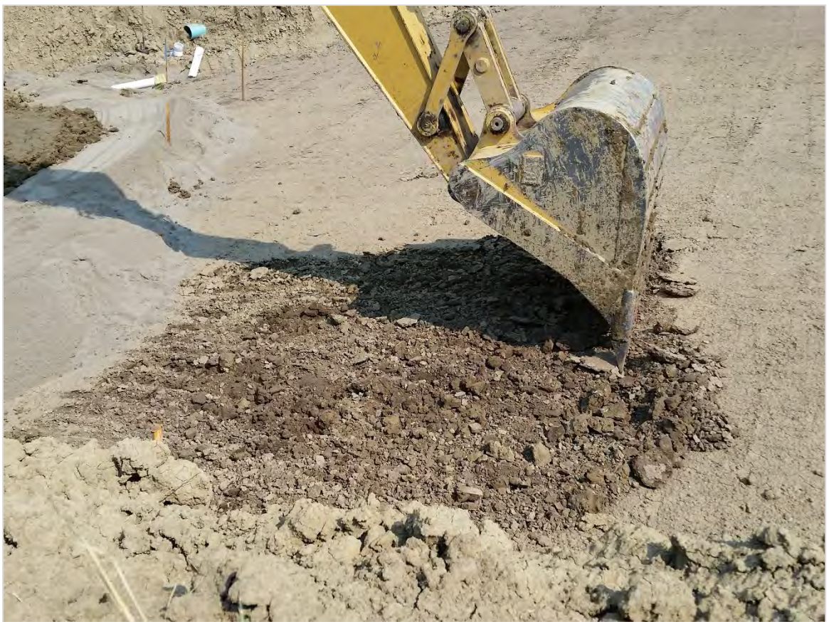
Photograph 20 shows scarification of the embankment with the bucket of the backhoe.
