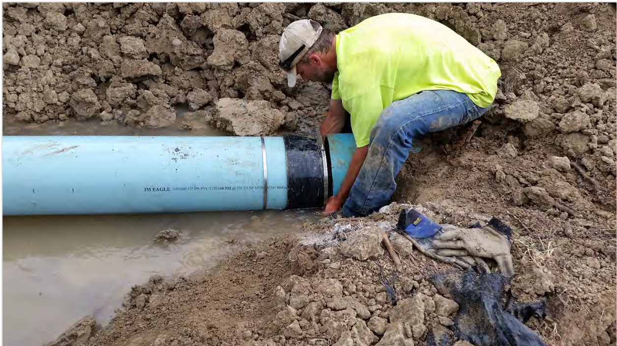
Photograph 26 showing the connection of the bypass line (left) to the existing pipe (right).
