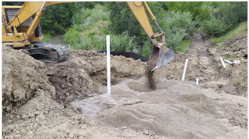
Photograph 18, below, showing placement of filter sand over the toe drain area.
