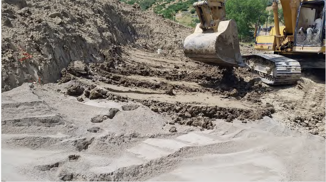
Photograph 25 showing the placement of a clay cap over the sand blanket.
