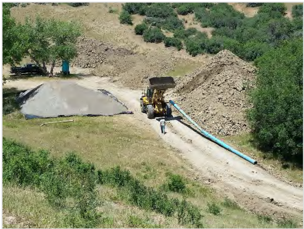
Photograph 10 (left): shows diversion pipe being exposed and Photograph 11 (right): show removal. Note the filter sand stockpile in the background.
