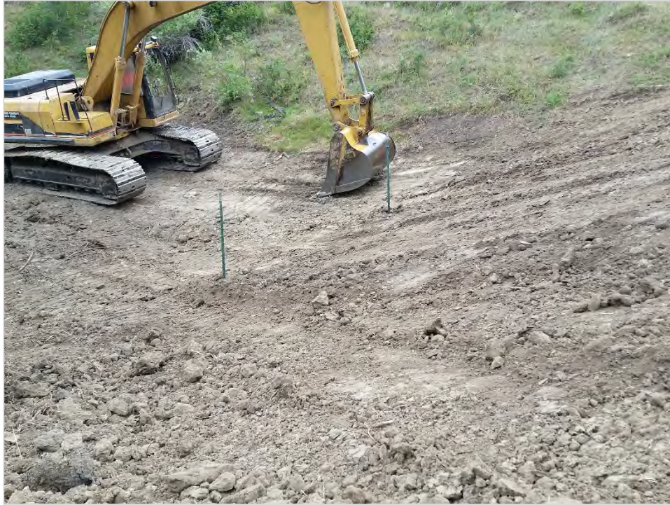
Photograph 29 showing the tracer wire attached to T-posts at each toe drain clean out/inspection port.
