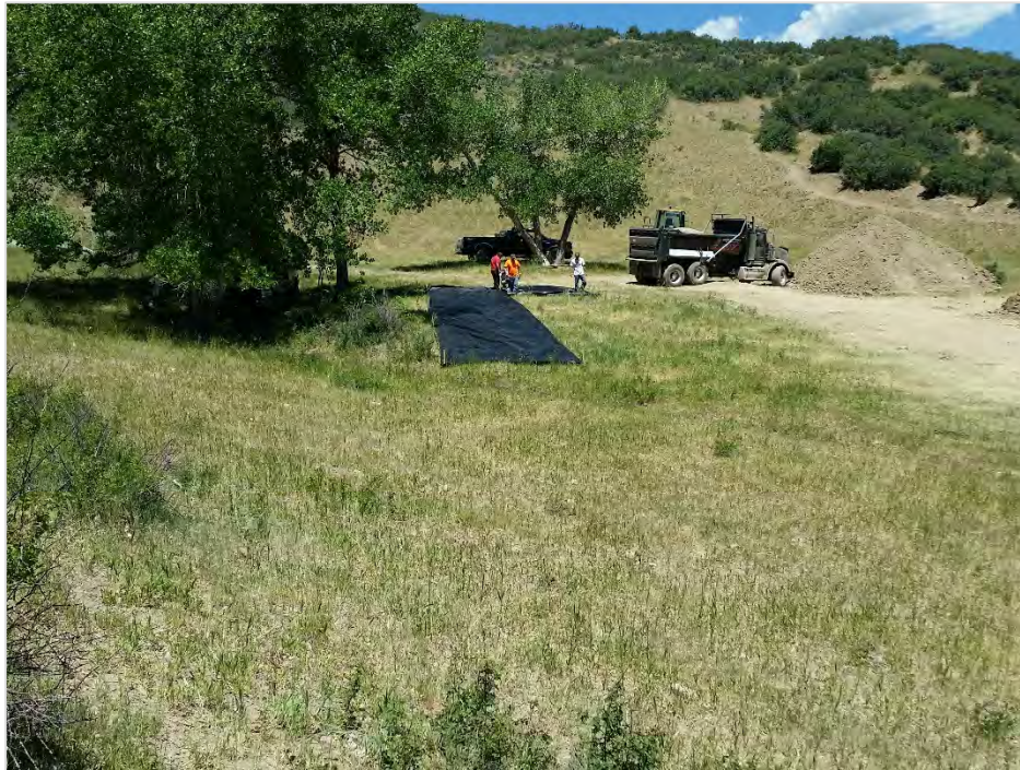
Photograph 5: Shows geotextile fabric being placed in area where filter sand will be stockpiled
