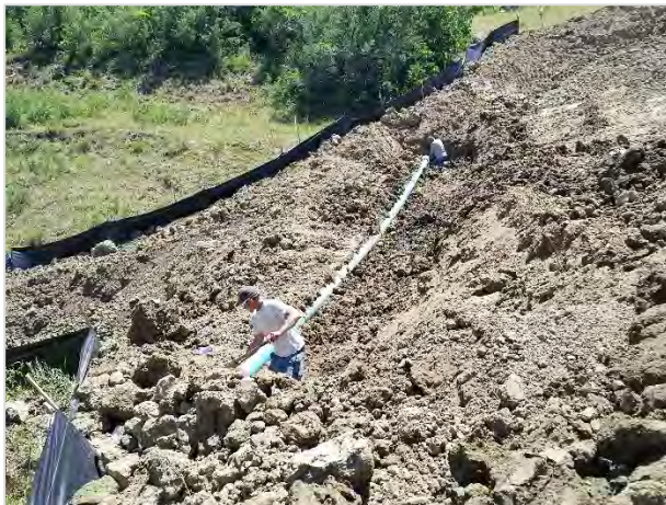
Photograph 10 (left): shows diversion pipe being exposed and Photograph 11 (right): show removal. Note the filter sand stockpile in the background.
