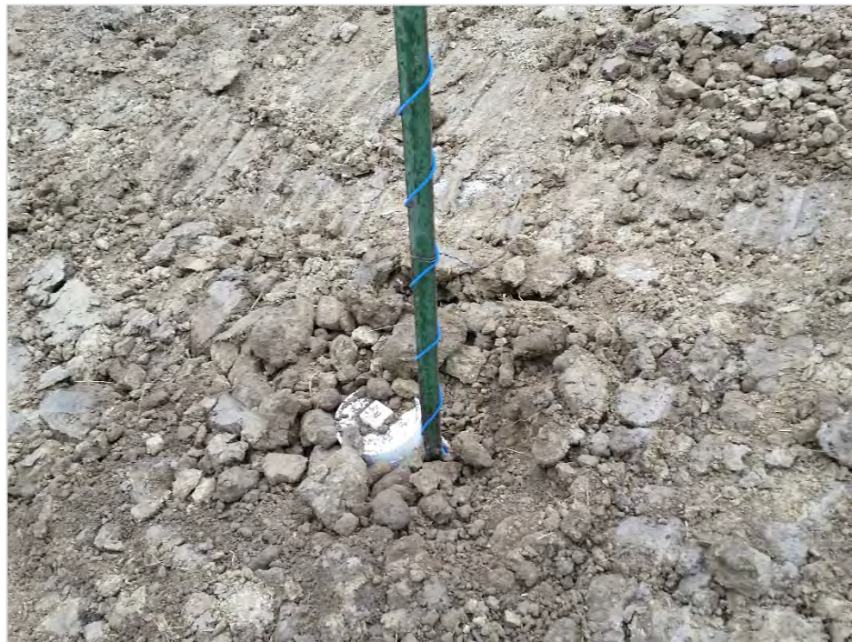
Photograph 30, detail of tracer wire secured to T-post at toe drain pipe clean out/inspection port.
