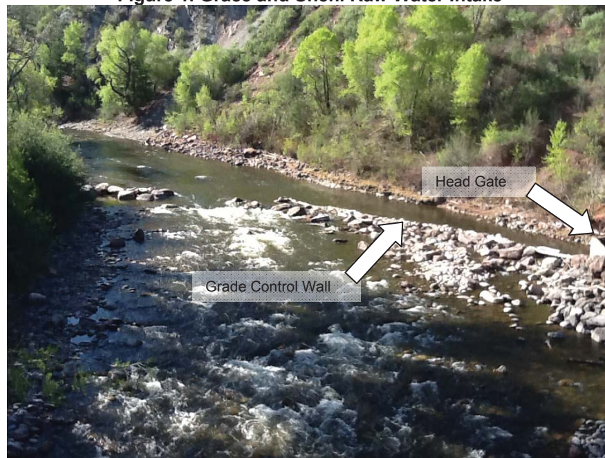
Figure 1. Grace and Shehi Raw Water Intake
