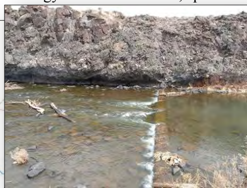
Existing Sanford Ditch Diversion
