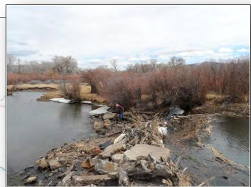
Existing Ephraim Ditch Diversion
