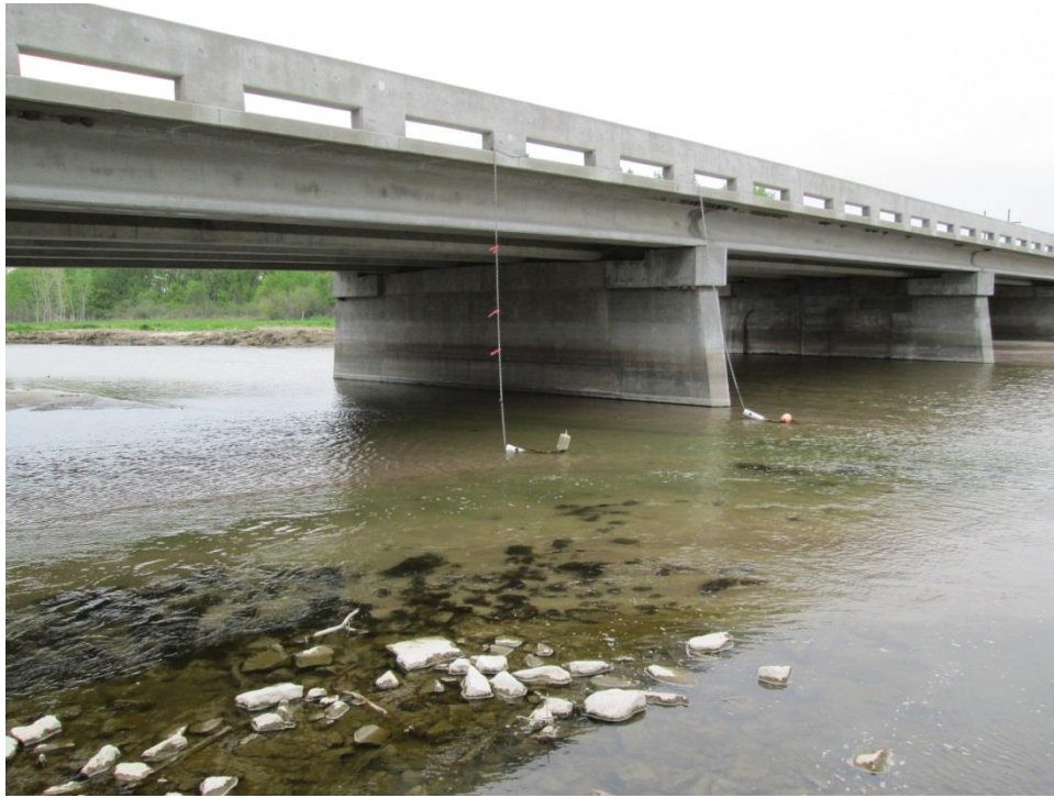
1. Manta 2 sonde deployment at Platte River at Elm Creek, NE (chain with flagging).
