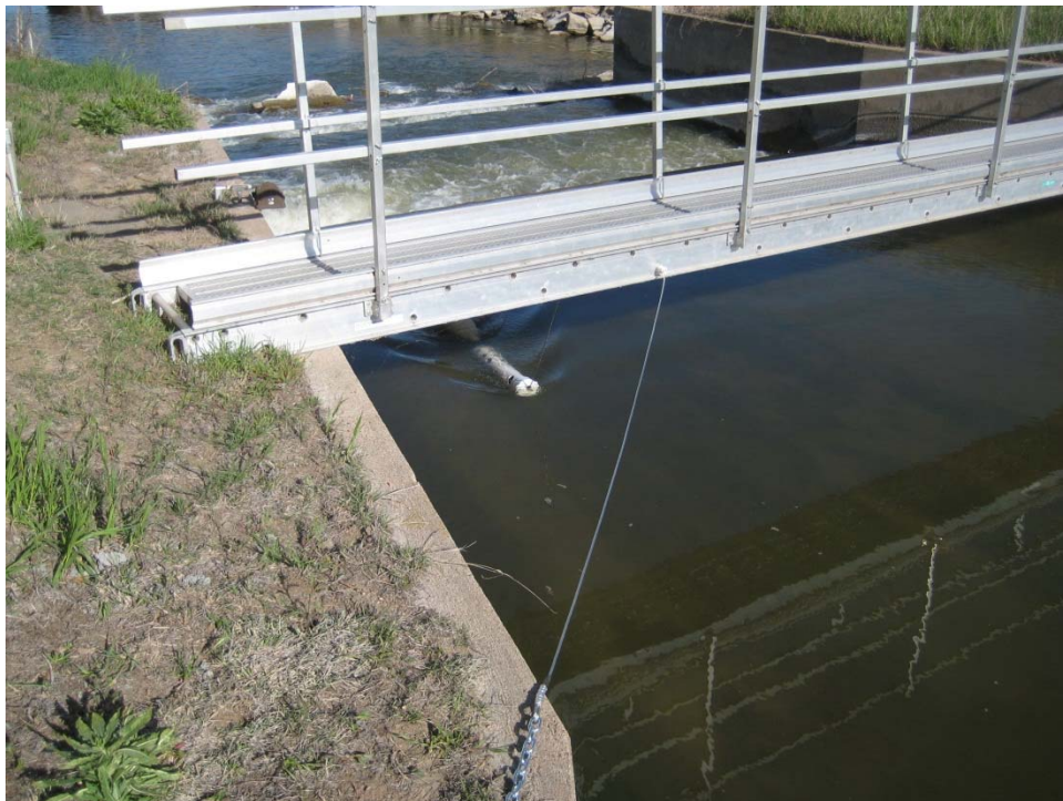
2. Manta 2 sampling location in the Kearney Canal downstream of the diversion near Elm Creek, NE.
