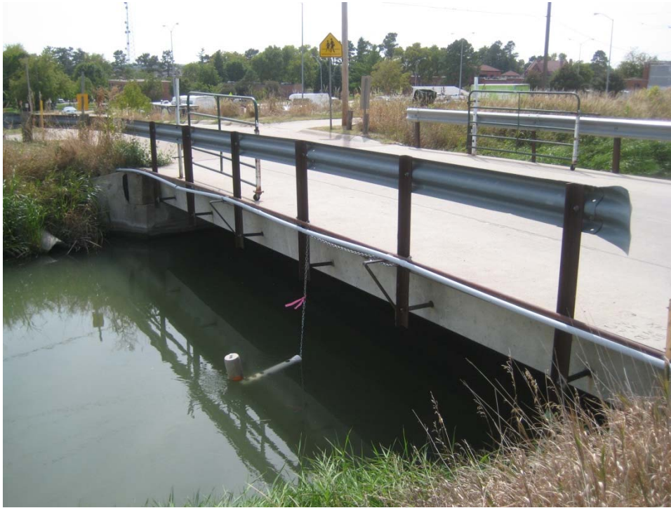
5. Manta 2 sonde deployment upstream of the Kearney Canal Hydro.
