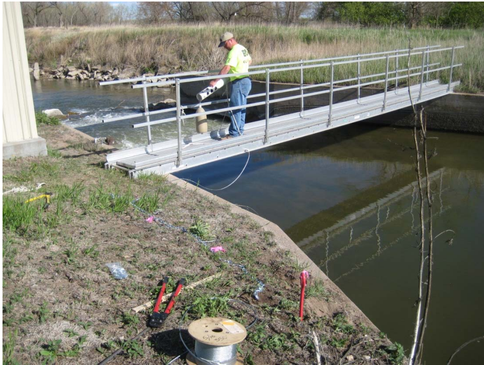
1. Manta 2 deployment into the Kearney Canal downstream of the diversion.
