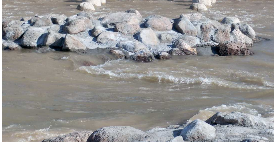
Figure 6 – Grouted Boulders
