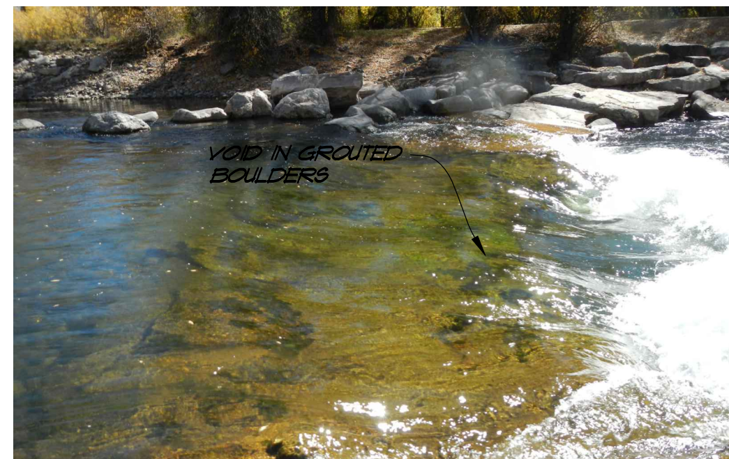
VOID IN GROUTED BOULDERS - BOAT CHUTE
