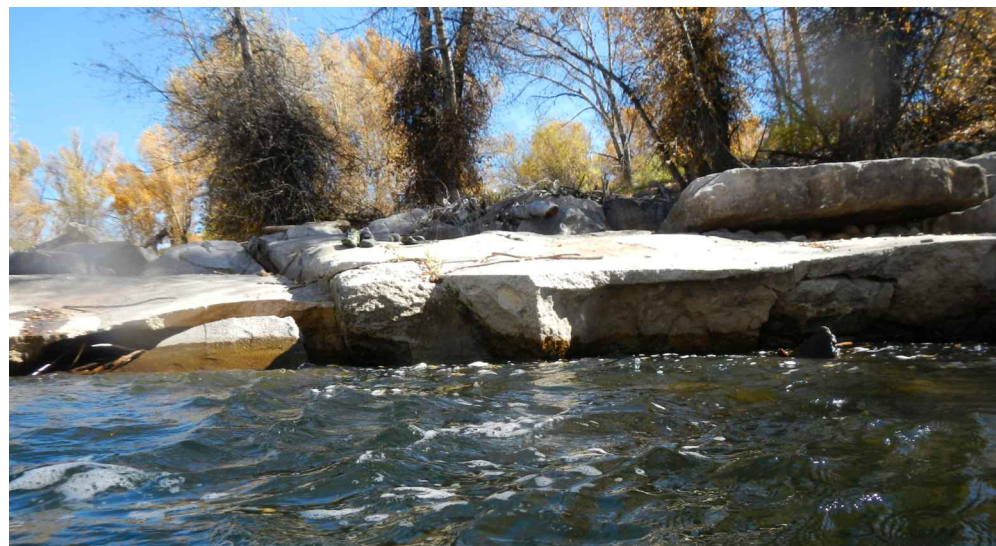
BOULDERS SEPARATED FROM STRUCTURE & UNDERCUTTING - RIVER LEFT SHOULDER
