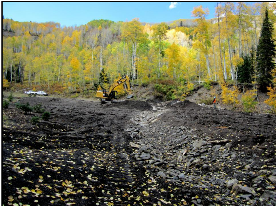
Figure 12. Area 2c alluvial fan during restoration.
