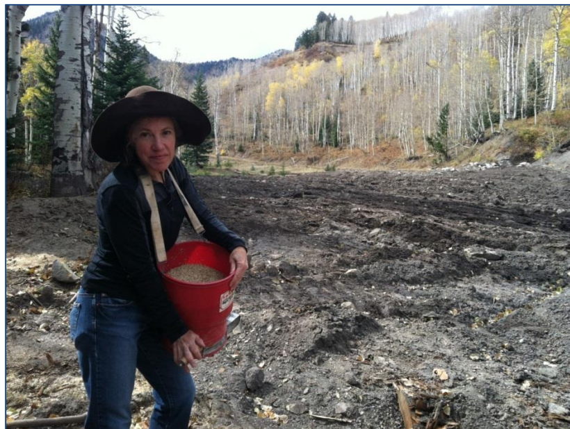
Figure 16. Reconstructed alluvial fan seeded with WRNF mountain brome, slender wheatgrass and blue wildrye.
