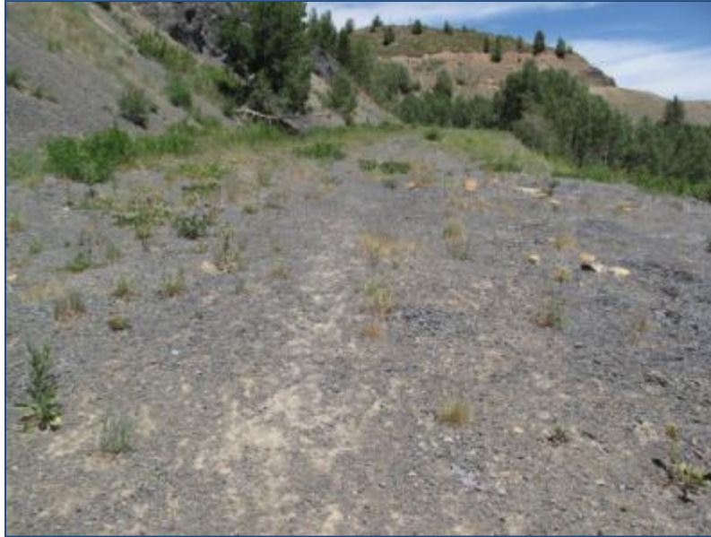
Figure 8. Road prism before treatment; road had minimal infiltration and excessive overland flow.
