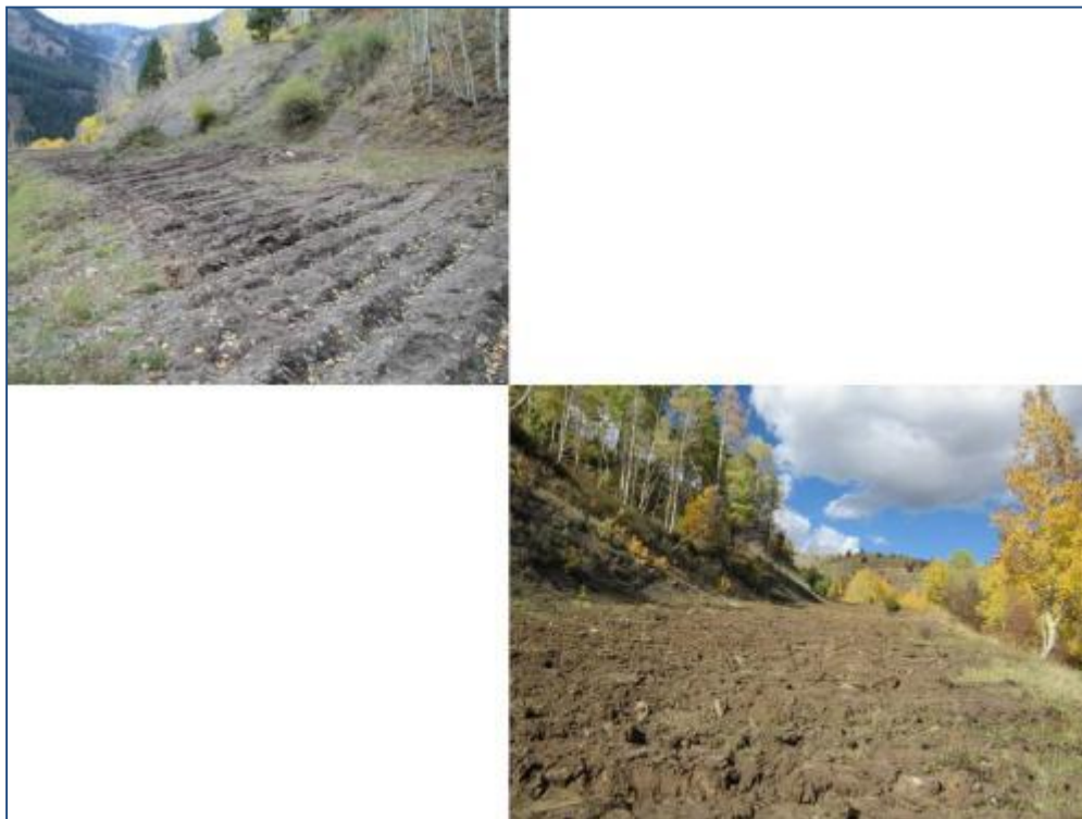
Figure 9. Cross-rippled road with compost/biochar soil amendment (above) and without soil amendment (below).
