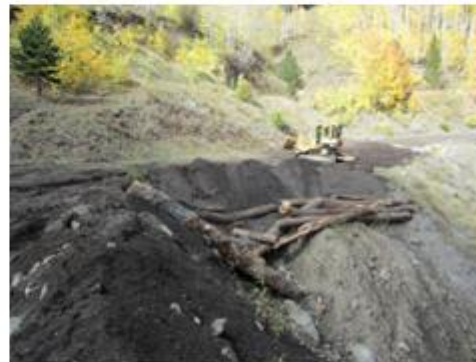
Figure 7. Area 2a during restoration.
