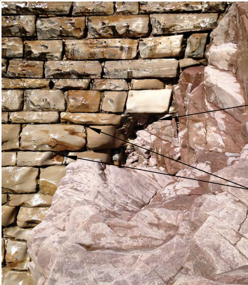
HOLE ON DOWNSTREAM LEFT ABUTMENT CONTACT APPROXIMATE 20FT BELOW CREST
