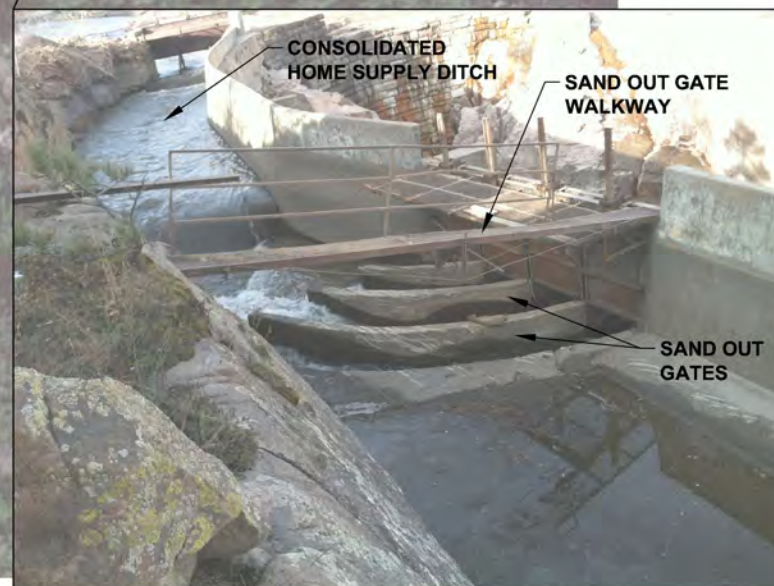
PHOTO C - SAND OUT & SLIDE GATES
