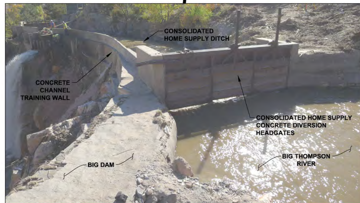
PHOTO A - CONSOLIDATED HOME SUPPLY CONCRETE DIVERSION STRUCTURE
