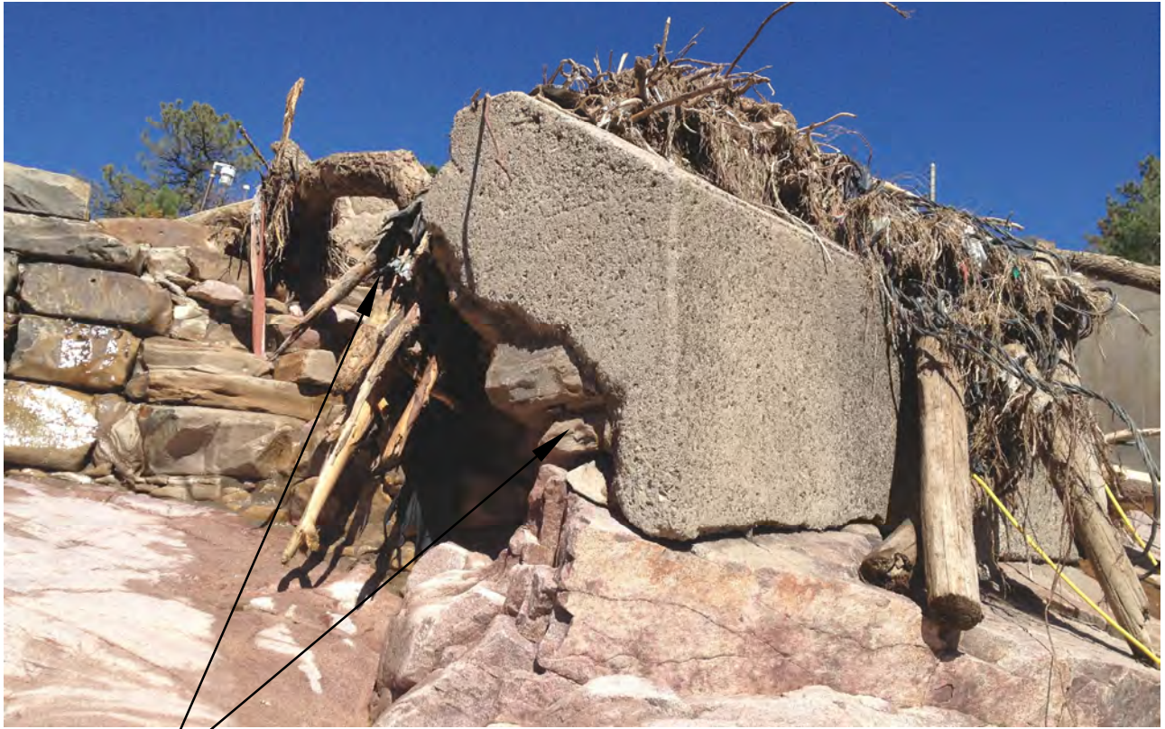
DAMAGED LEFT ABUTMENT BUTTRESS
