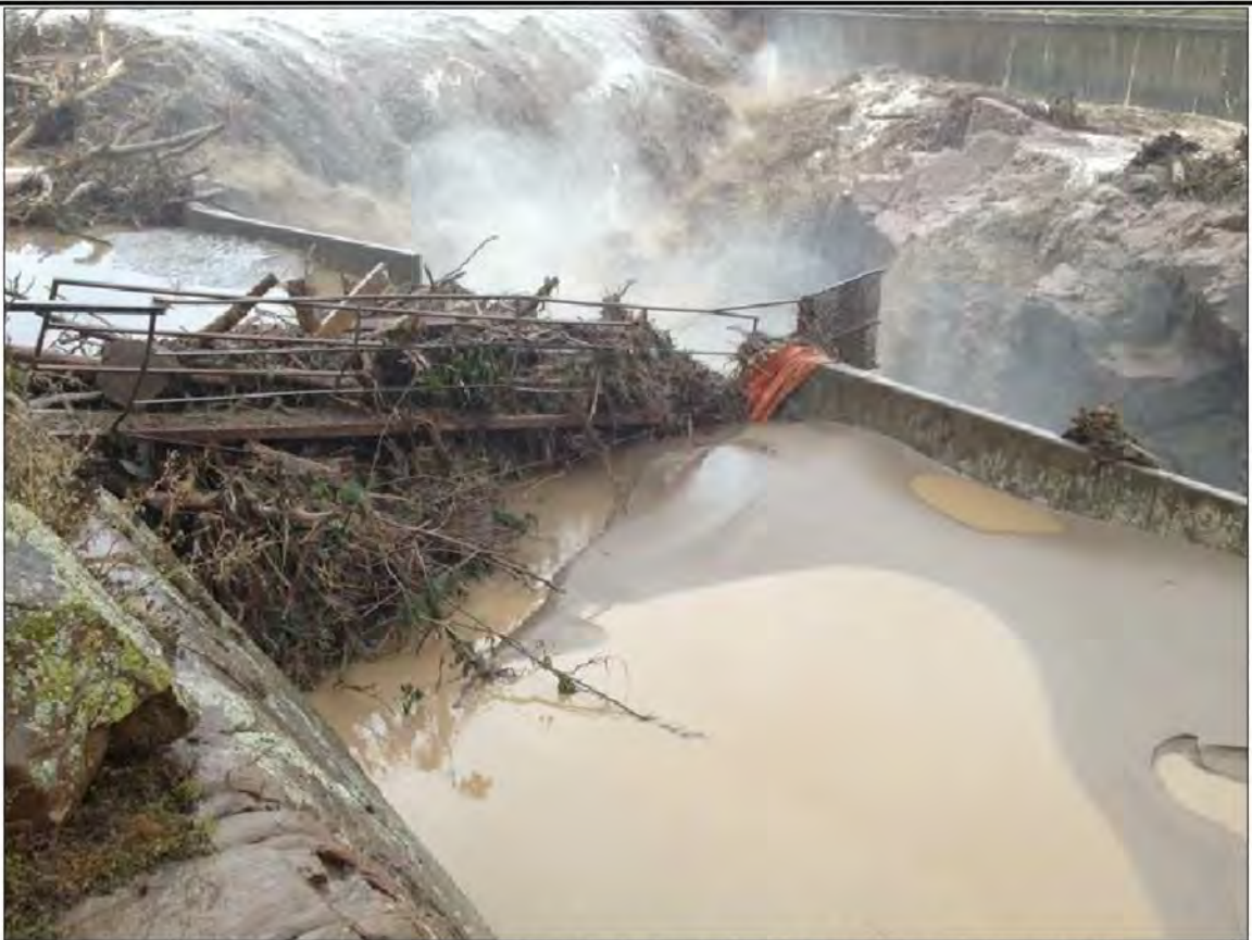
PHOTO 1 - DEBRIS AGAINST SAND OUT GATES ACCESS WALKWAY
