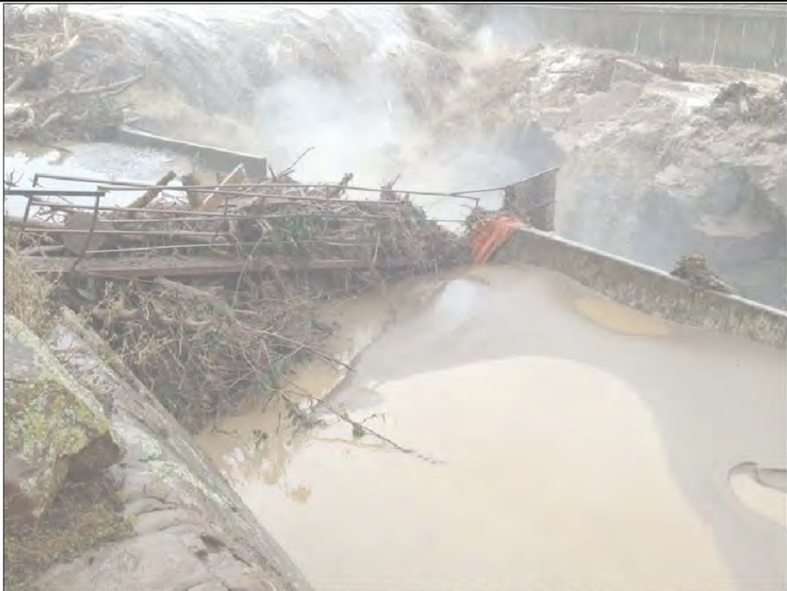
PHOTO 1 - DEBRIS AGAINST SAND OUT GATES ACCESS WALKWAY
