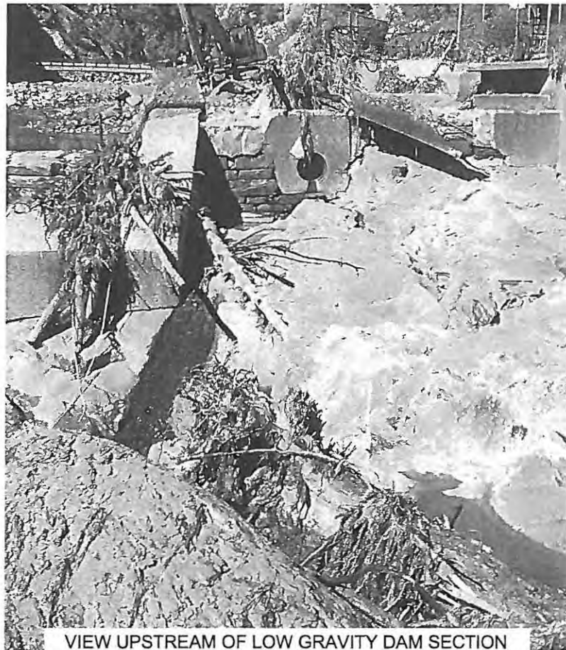
CREST WITH MASONRY RUBBLE
