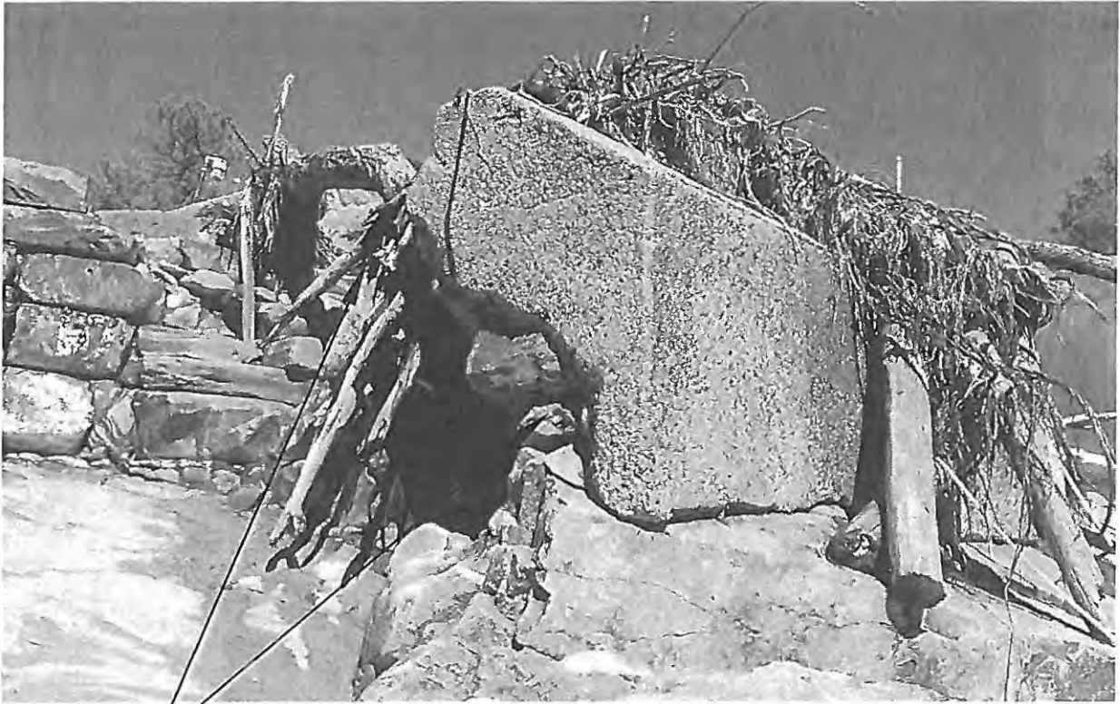
DAMAGED LEFT ABUTMENT BUTTRESS
