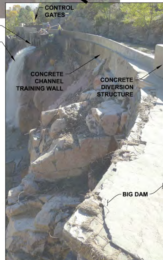
PHOTO B - SAND OUT & CONTROL GATES
