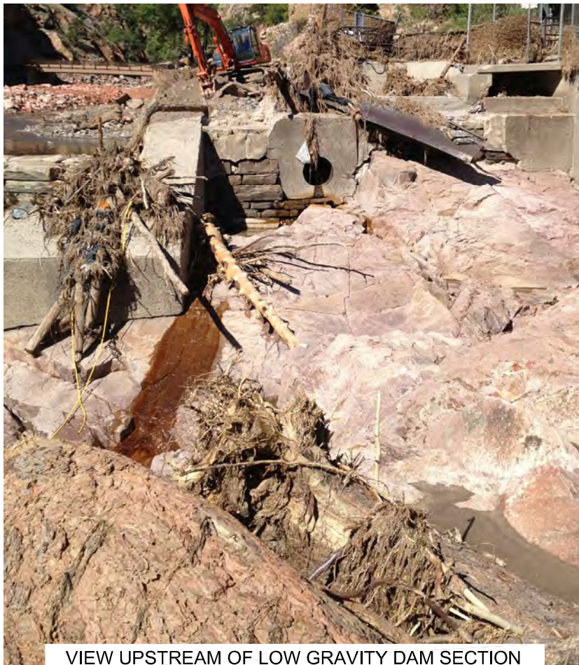
CREST WITH MASONRY RUBBLE
