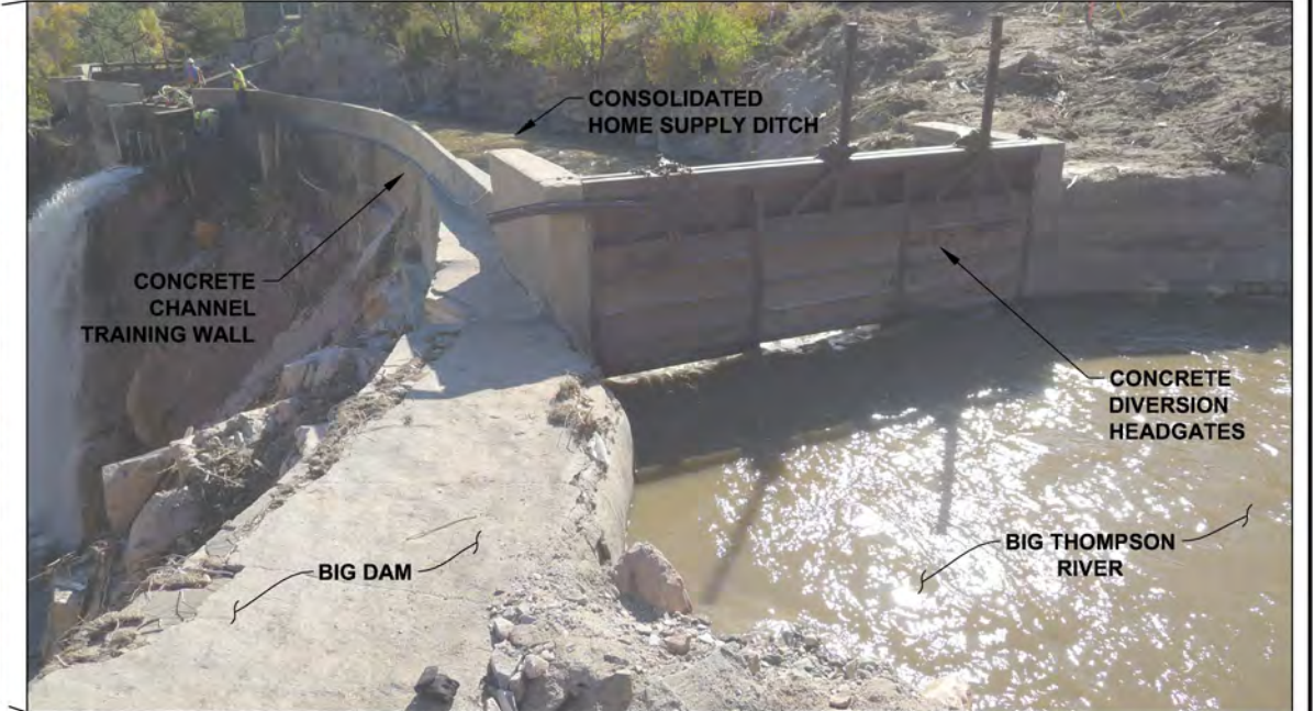
PHOTO A - CONCRETE DIVERSION STRUCTURE
