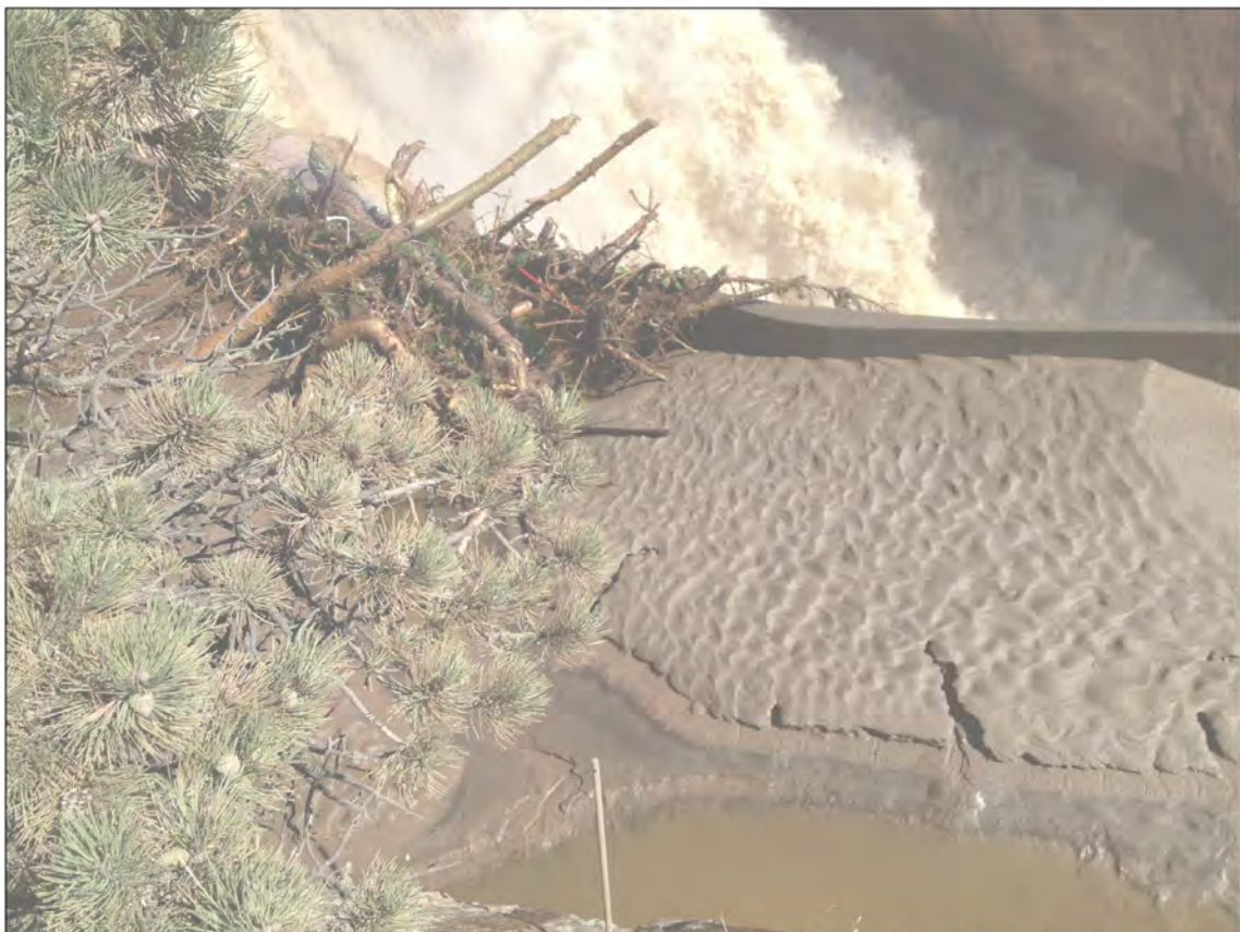
PHOTO 2 - SEDIMENT FILLED IRRIGATION CHANNEL UPSTREAM OF THE SAND OUT GATES
