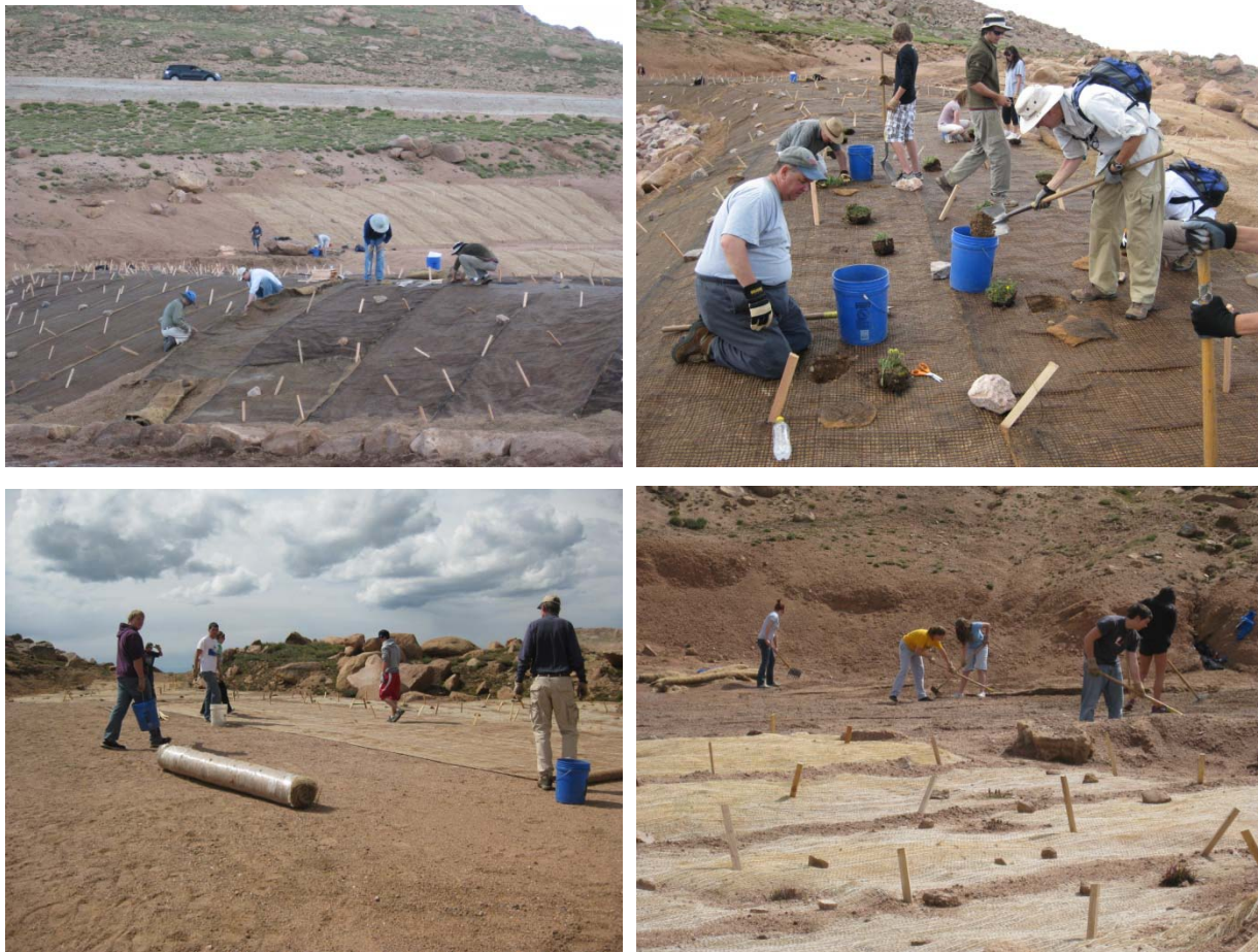
Figure 5-8. Volunteer crews completing bank stabilization.
