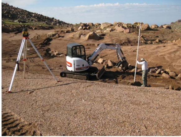
Figure 1 and 2. Installing cross-vanes and bank stabilization.
