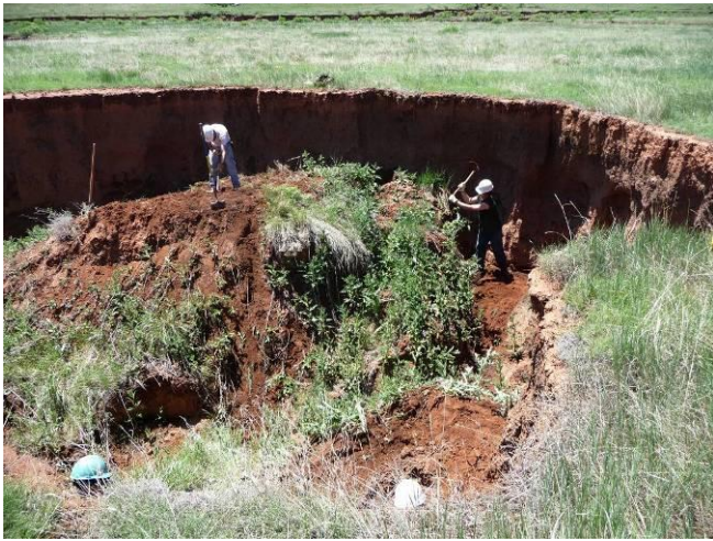
Regrading soil pillars by hand to reduce snow-based saturation points near headcuts and the base of valley walls. Additional grading was completed by excavator.
