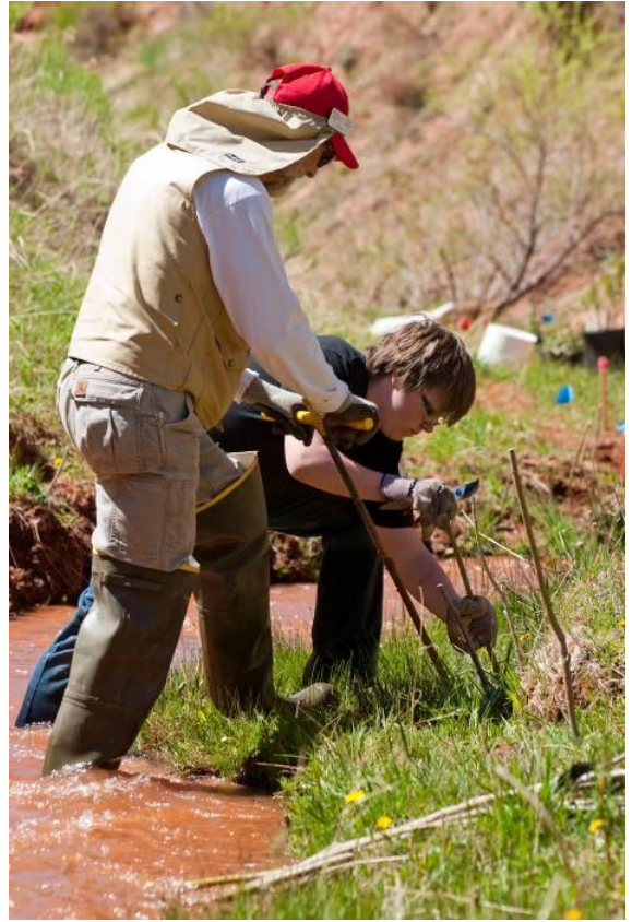
Installing willow cuttings with willow probes.
