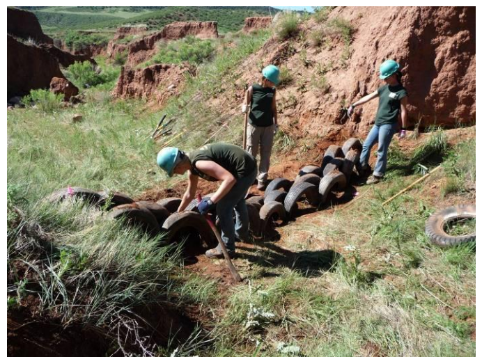
Vertical Tire Check Dam.
