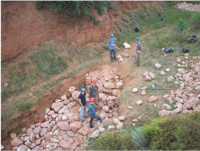
Construction of 4-step step pool with 6-foot headcut.
