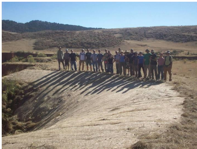
Finished erosion matting along regarded valley trench wall.
