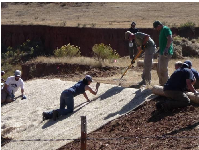
Odell Brewing staff spread seed and install erosion matting.
