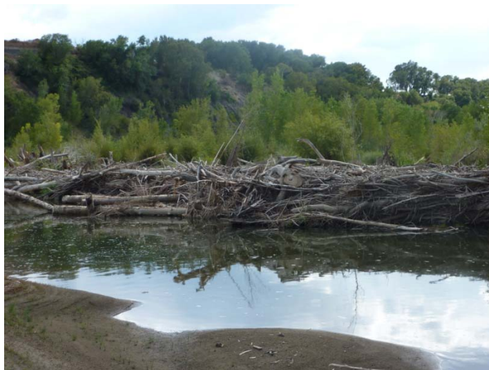
Avulsion channel blocked by woody debris caught in log structures
