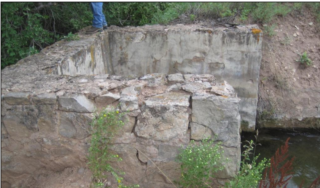
Photograph 18.—Silt Project Grass Valley Siphon 2 Outlet Structure.
