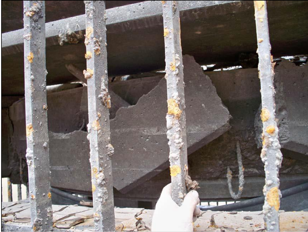
Photograph 12.—Paonia Dam Outlet Works Inlet and Bulkhead Damage.
