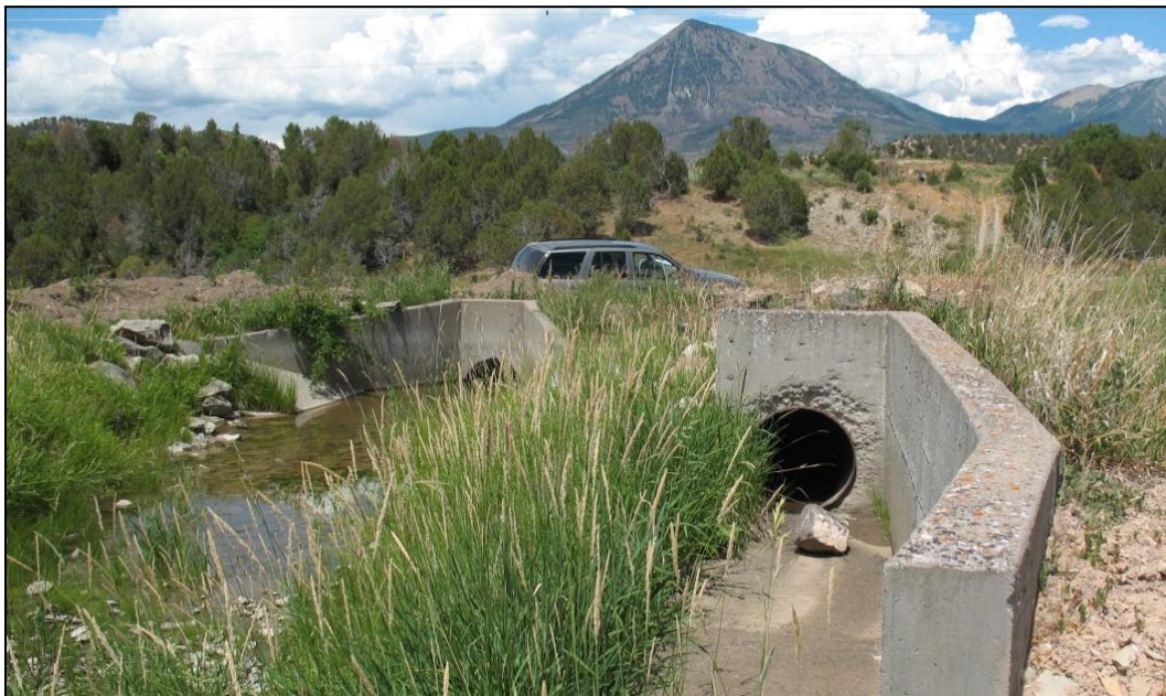
Photograph 23.—Smith Fork Project Feeder Canal Siphon Outlet.
