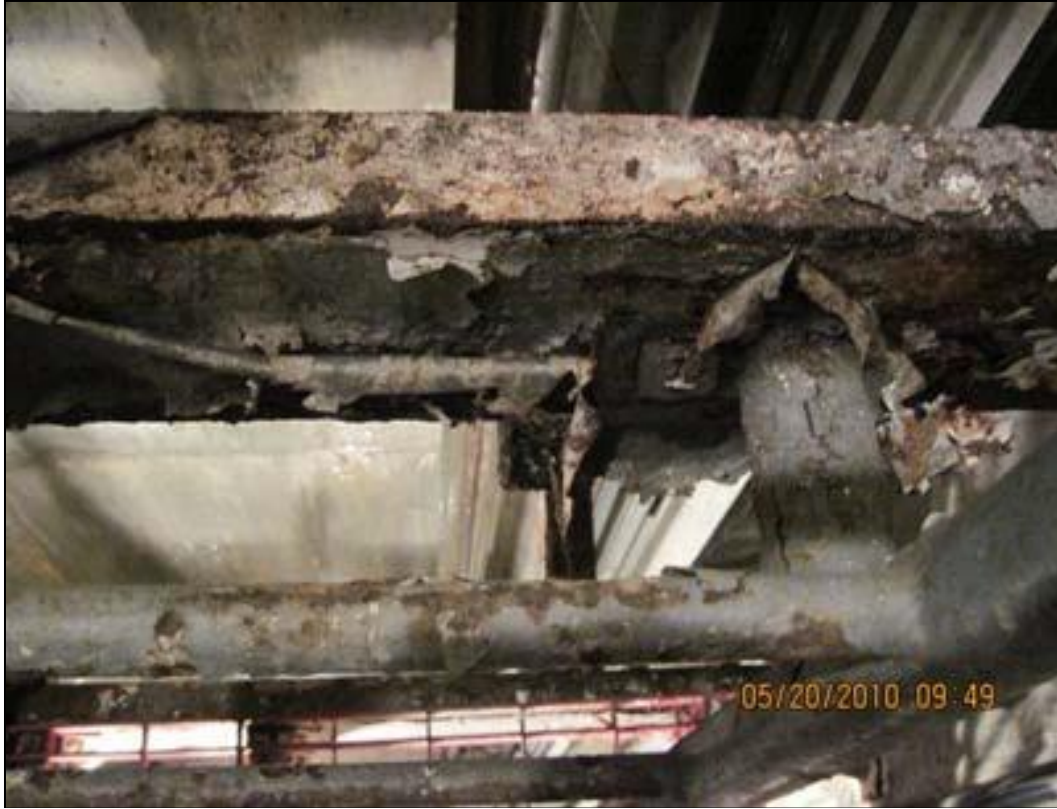
Photograph 11.—Paonia Dam Elevator Shaft Metal Corrosion.
