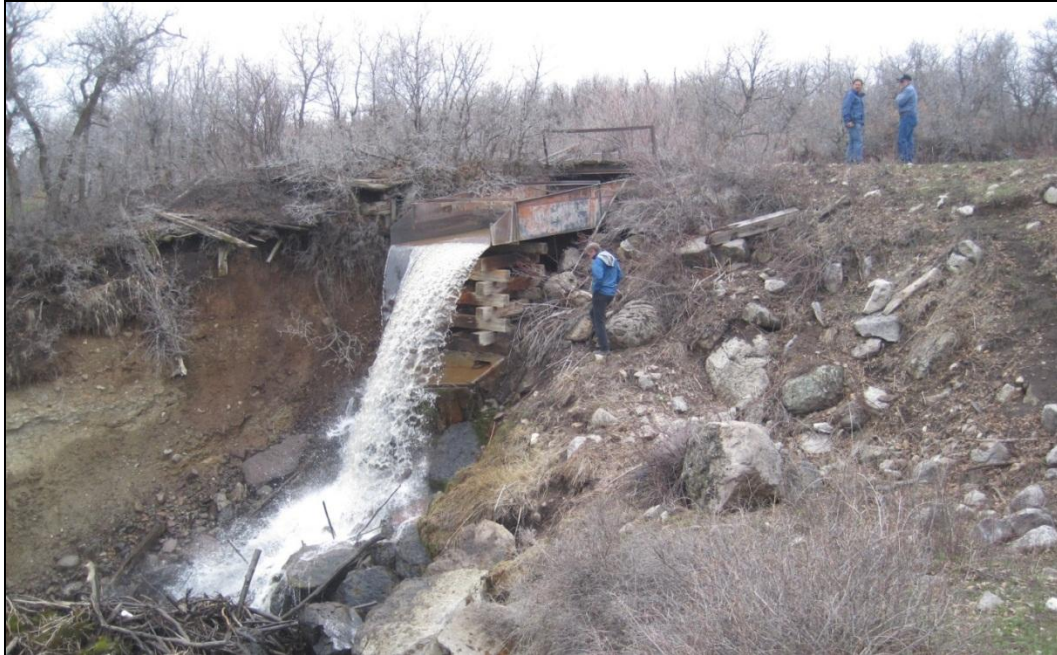
Photograph 3.—Erosion of Bostwick Park Vernal Mesa Ditch below Cimarron Ditch diversion structure.
