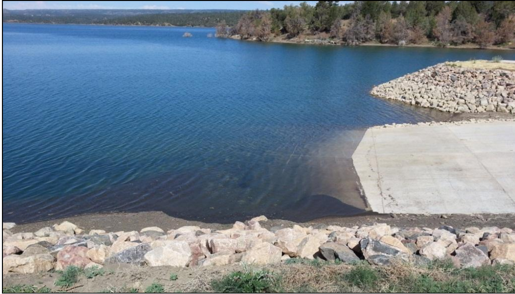
Photograph 1.—Lake Nighthorse boat ramp with eroded materials deposition (Animas-La Plata Project).
