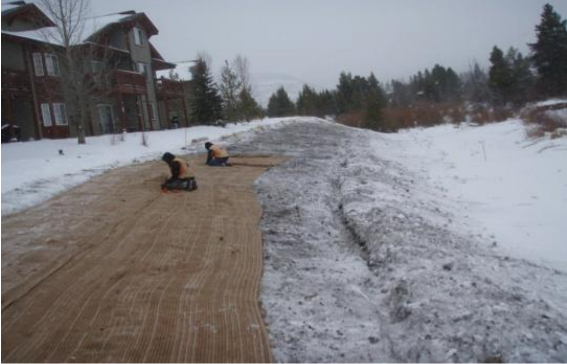
Just ahead of the winter's first major blast, Friday Dec. 14 was dedicated to seeding and the placement of erosion control fabric. The heavy equipment was moved out on Saturday Dec. 15.
