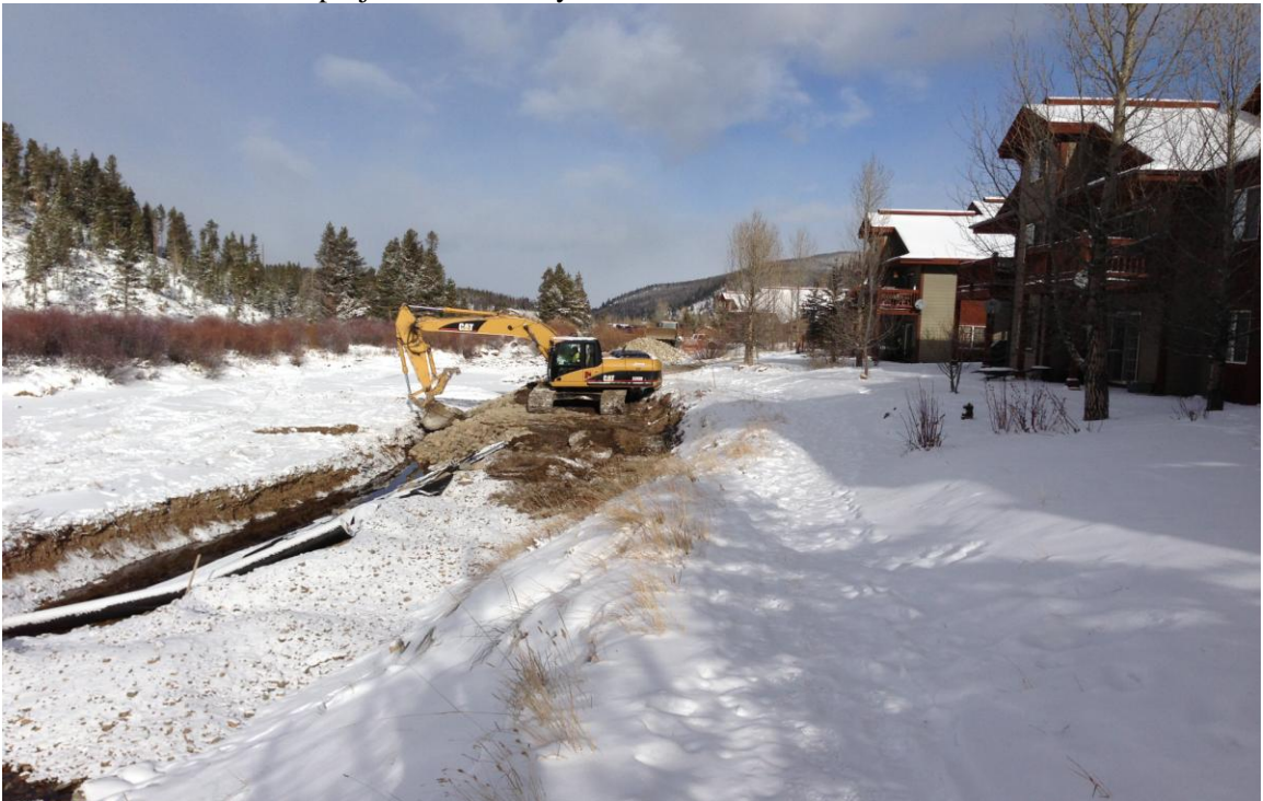
Day one sees the placement of almost 200 feet of cobble toe.
