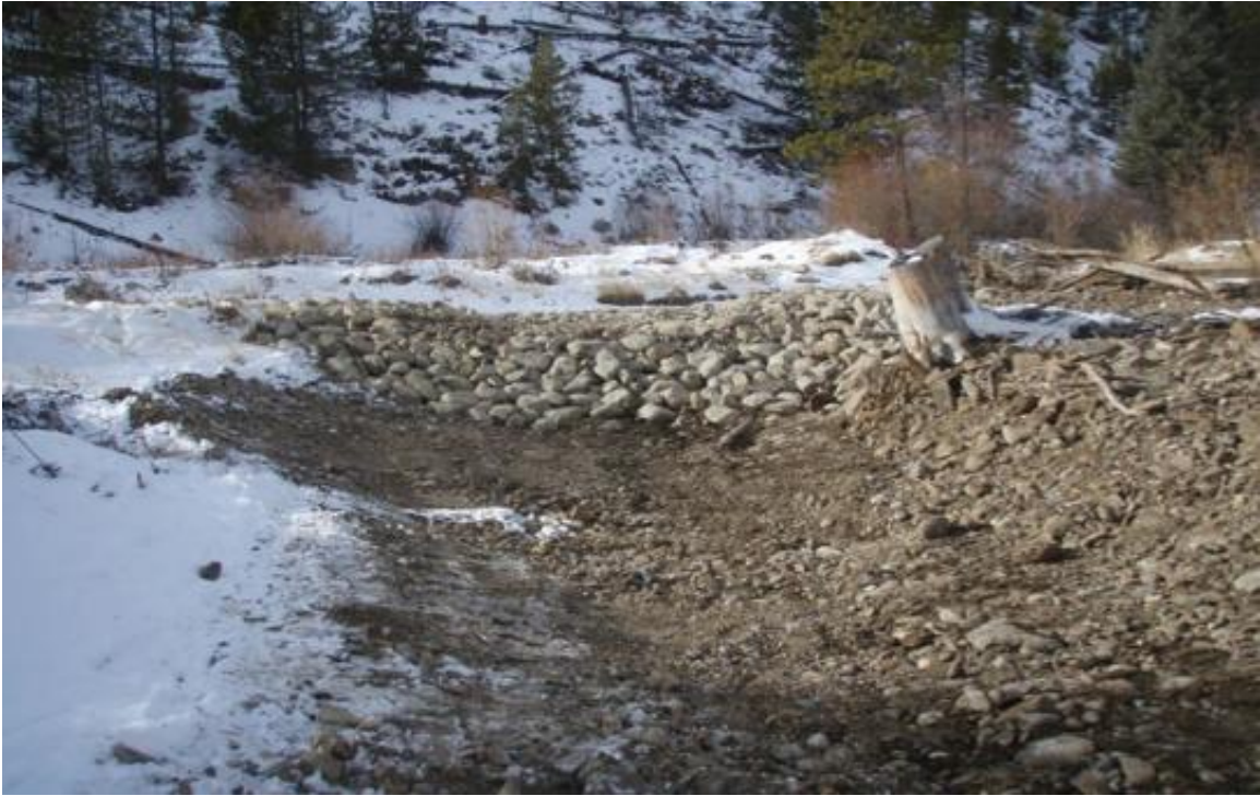
A cobble side channel split is constructed upstream.
