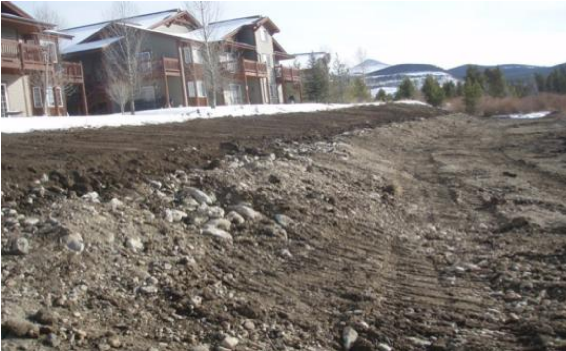
Days 2 and 3 entailed grade control and channel cutting
