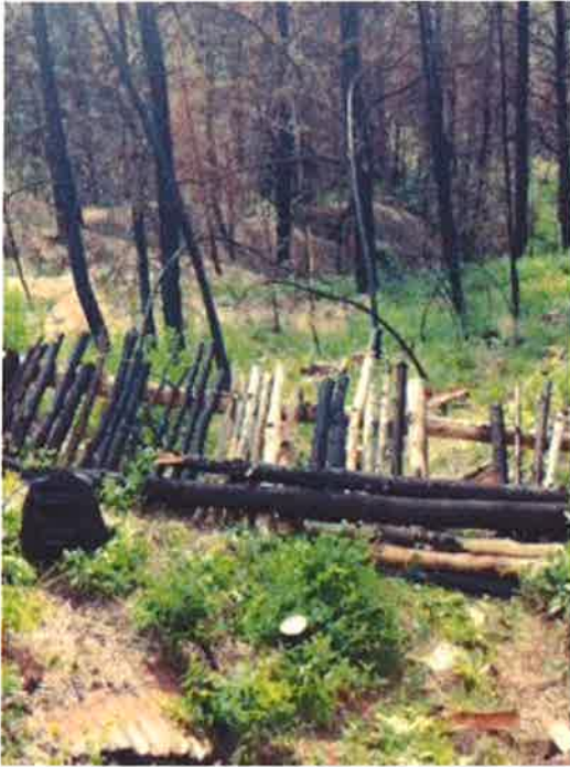
Check Structure, As Built
