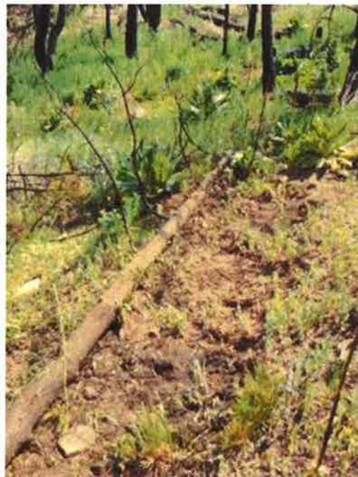
Contour Felling, As Built
