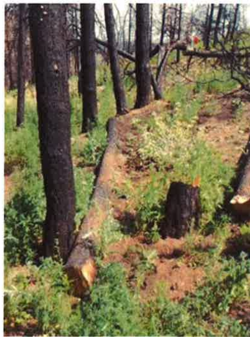
Contour Felling, As Built
