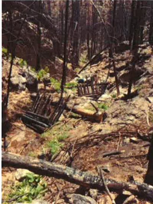
Check Structures, As Built
