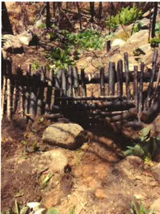
Check Structure, As Built
