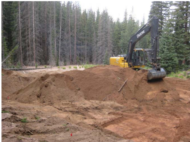
Figure 1. Heavy equipment used to remove alluvium deposition in Tin Barn Wetland during 2012 work.
