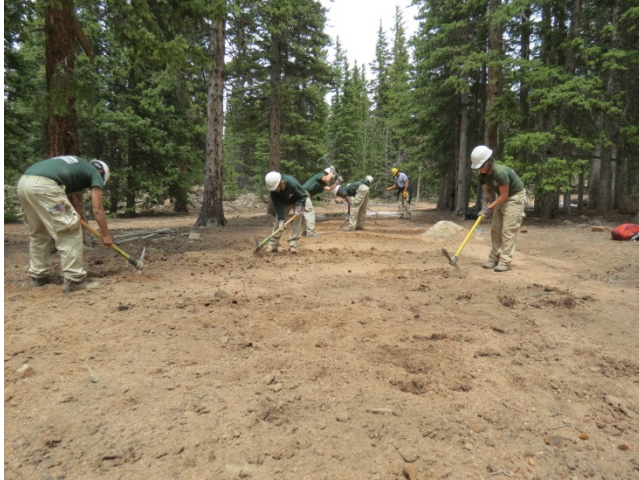
Figure 5. MHYC members hand decompacting wetland access road during 2013.
