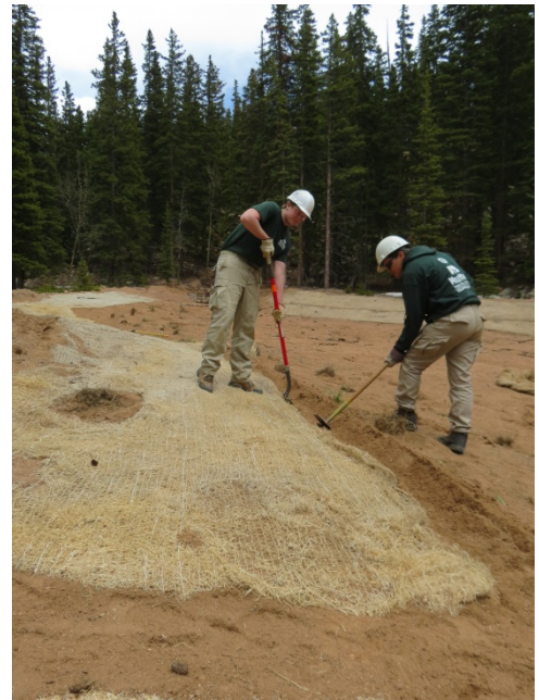
Figure 6. Installation of erosion control matting near Tin Barn Wetland during 2013.
