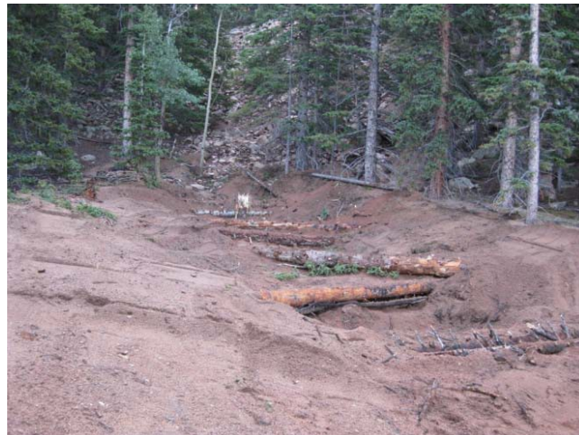
Figure 2. Log 'rock and roll' structures installed during 2012 work.
