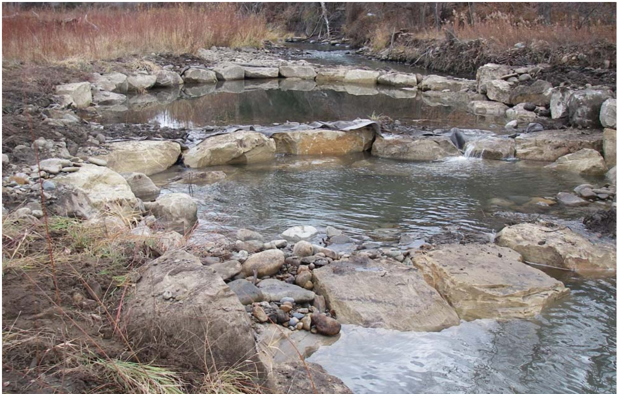
POST: Upstream view of cross vane structures.
