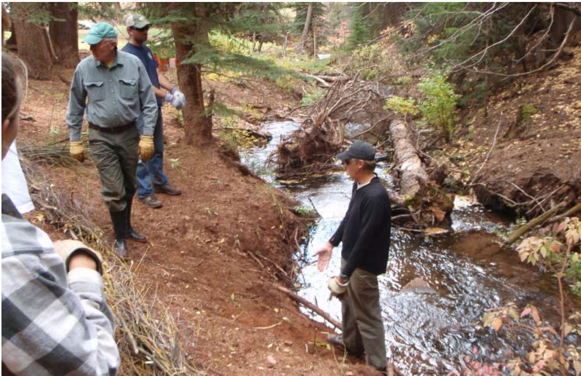
US Forest Service East Fork Red Dirt Creek streambank restoration.
