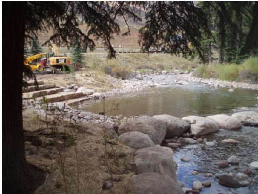
Streambank and channel restoration work completed by the Town of Vail at Stephens Park in lower Gore Creek's gold medal designated waters.
