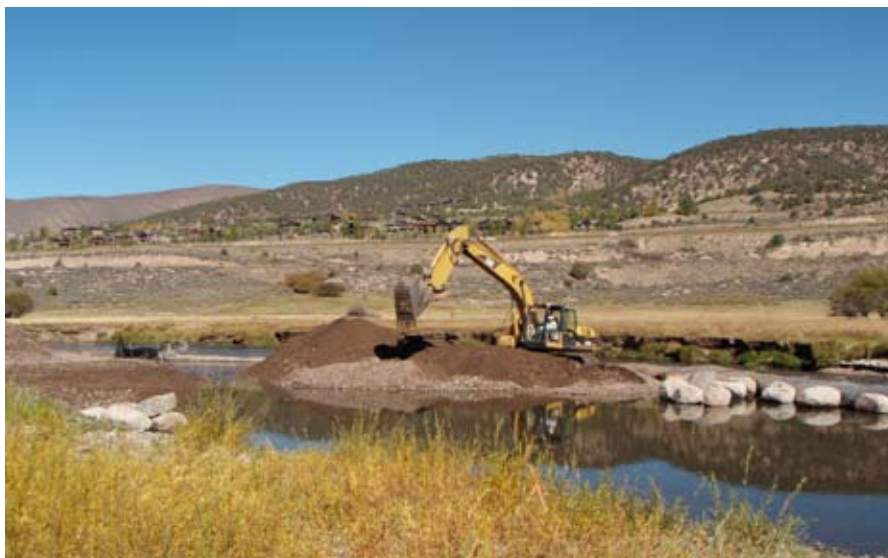
Restoration work on the Middle Eagle near Edwards.
