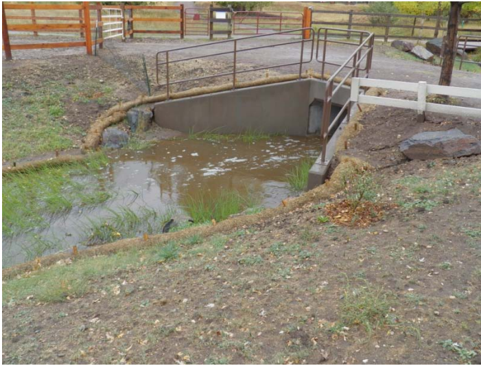
9. Post-construction photo of downstream end of box culvert.
