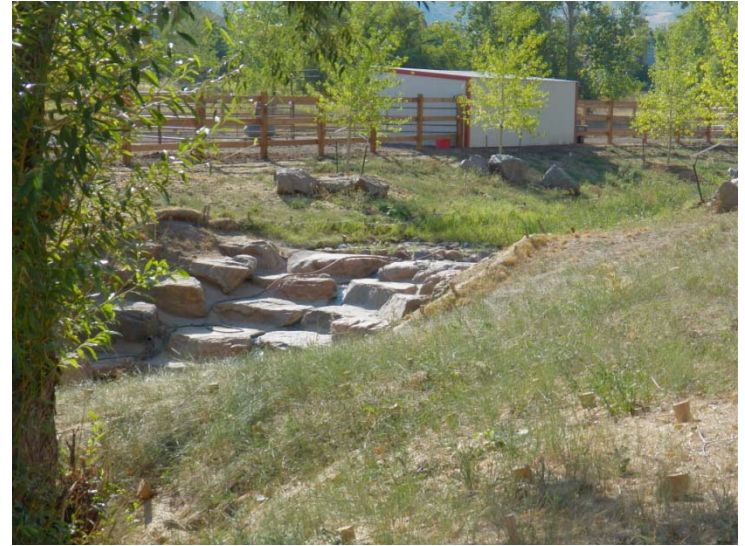
2. Post-construction photo of same location. Culvert was Replaced with open channel.
