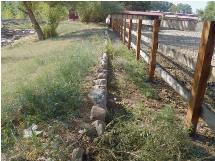
11. Post-construction photo of rock lined berm designed to prevent manure from entering drainage.
