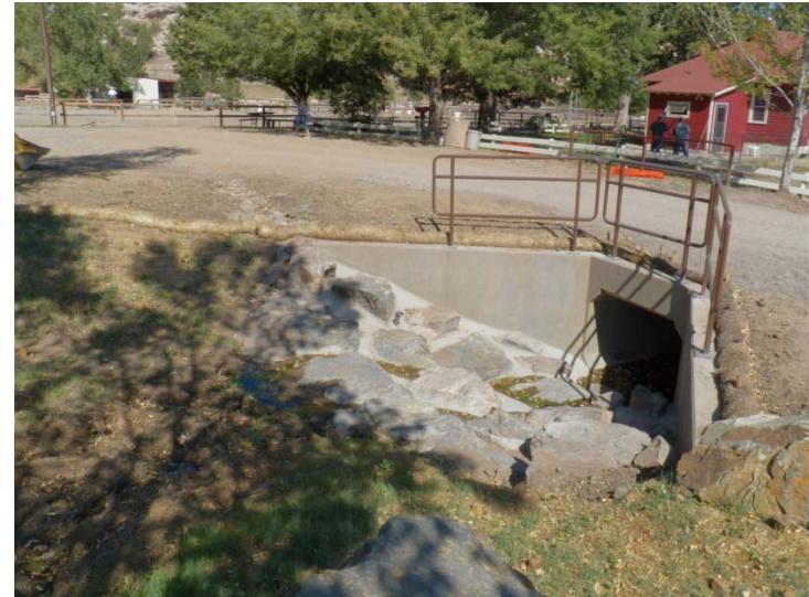
10. Post-construction photo of upstream end of box culvert.
