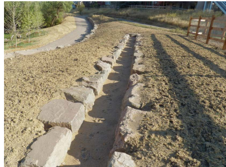
11. Post-construction photo of water quality trench. Run-off from Adjacent pasture is intercepted by the trench and treated Before entering the stream channel.
