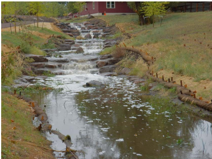
15. Post-construction photo of grouted boulder drop structures During storm event.
