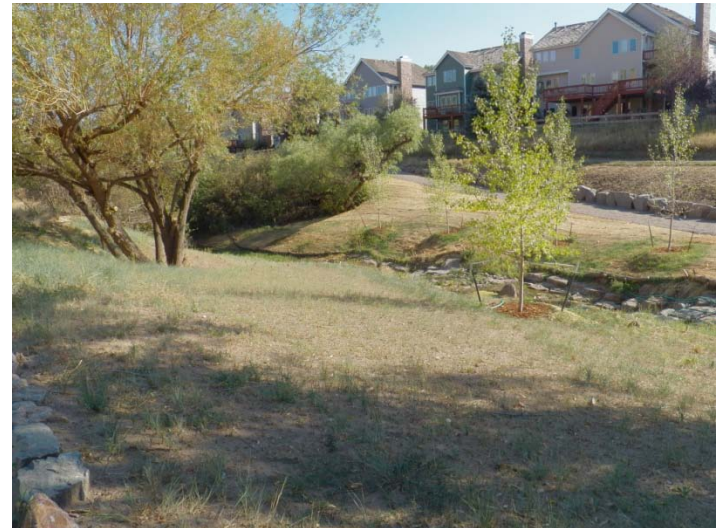
4. Post-construction photo of same general area. Tree in Upper left corner is same tree in pre-const. photo. New Stream channel is south of old channel with extensive bank grading
