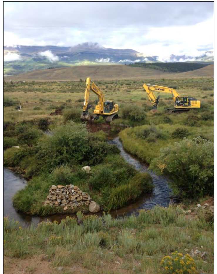
Figure 30. Two of the three excavators working in the Meander 1 Area.
