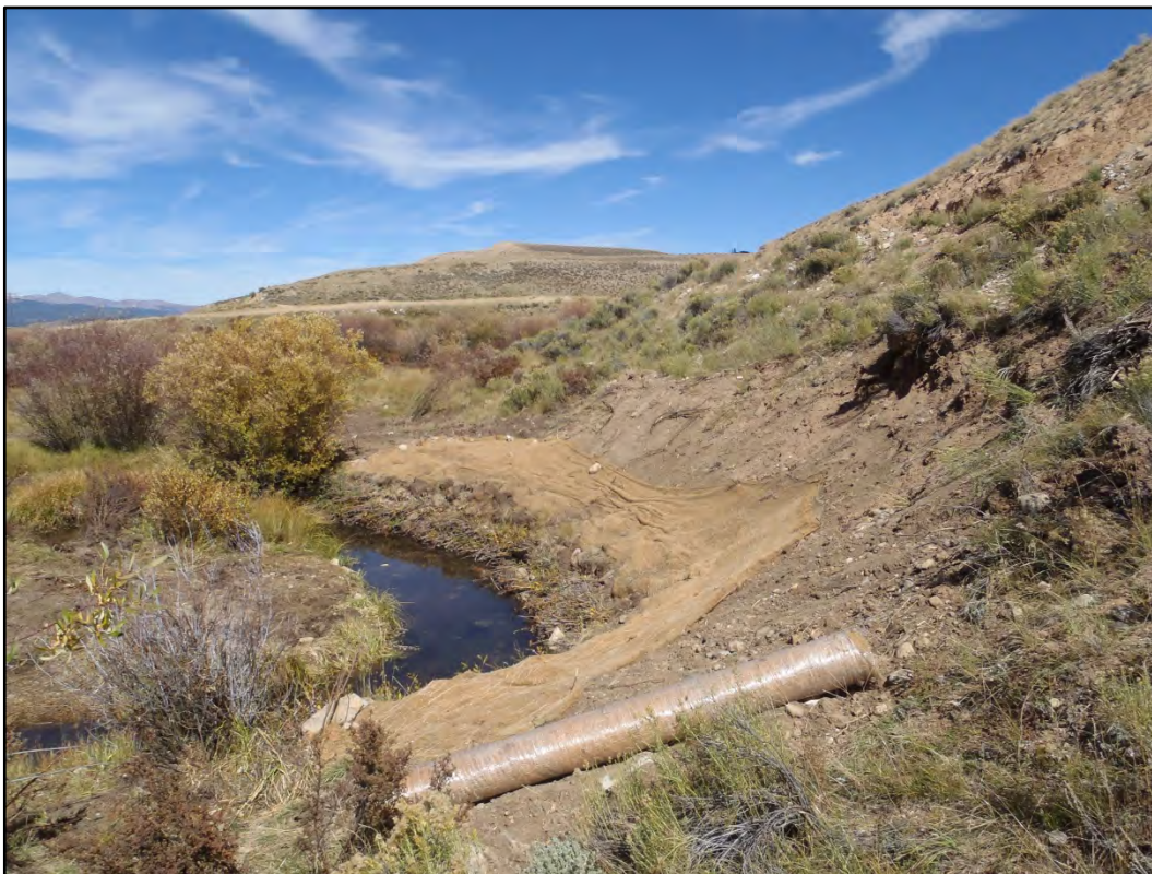
Figure 6. Post-construction of Meander 1.
