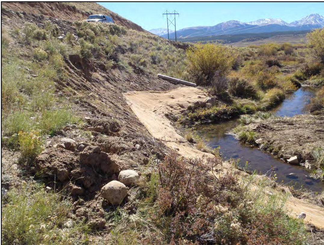
Figure 8. Post-construction photo of Meander 2.
