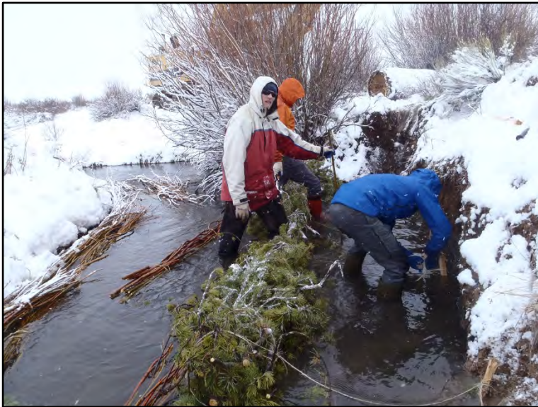
Figure 18. Staking pine bough fascines to the back of the bank.
