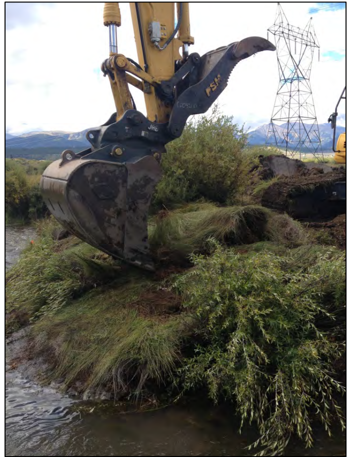
Figure 27. Laying sod mats and willow transplants near Meander 2.
