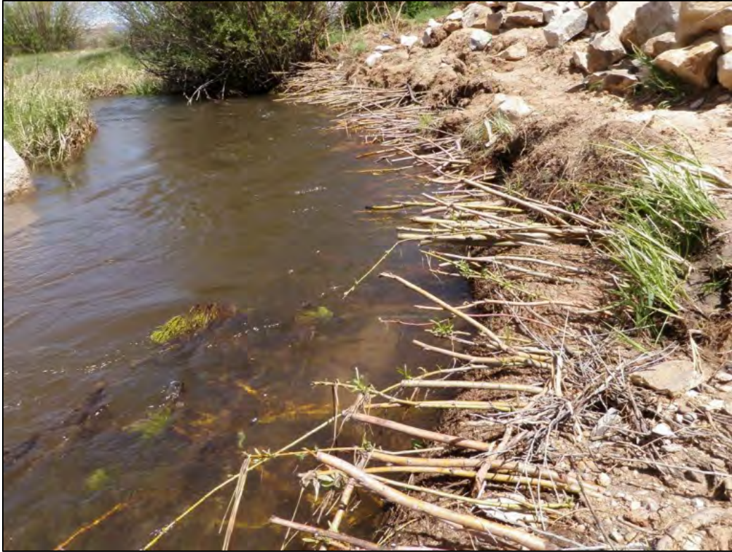
Figure 23. Willow growth in soil lift May, 2013. Note pine bow fascine below water.
