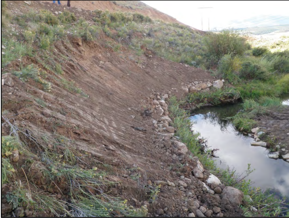
Figure 21. Completed soil lift.
