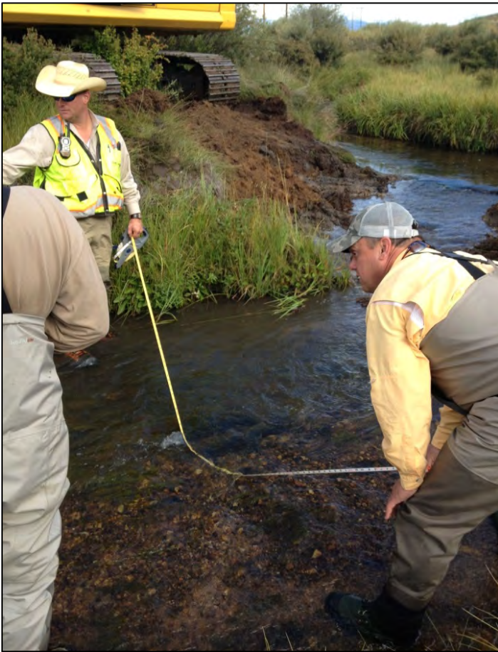
Figure 29. Lining out the new channel.
