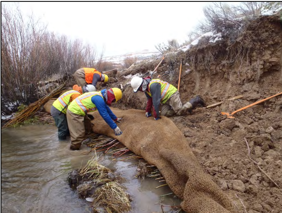
Figure 20. Folding Coir fabric over soil.
