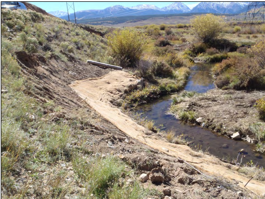
Figure 2. Photo Point 1 – Meander 1 Post-Construction
