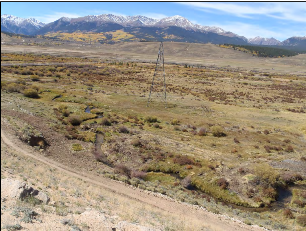
Figure 8. Photo 2b- Channel realignment post-construction.
