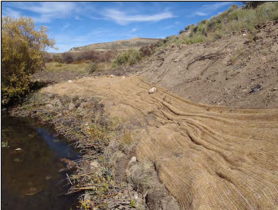
Figure 22. Soil lift with erosion mats at Meander 1.
