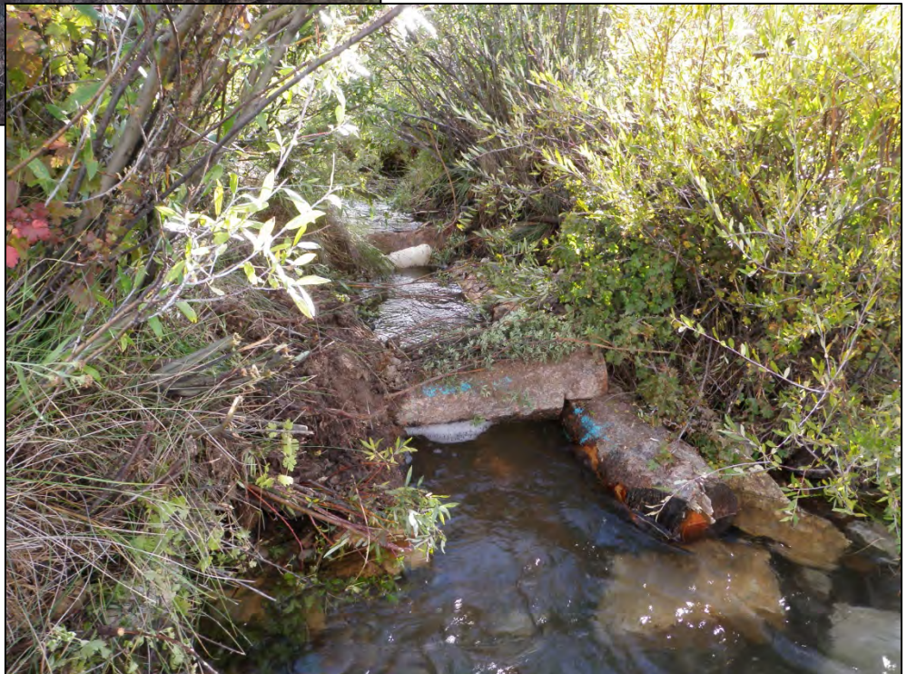
Figure 33. Log diversion structure used to divide flow into two separate channels creating better fish habitat.
