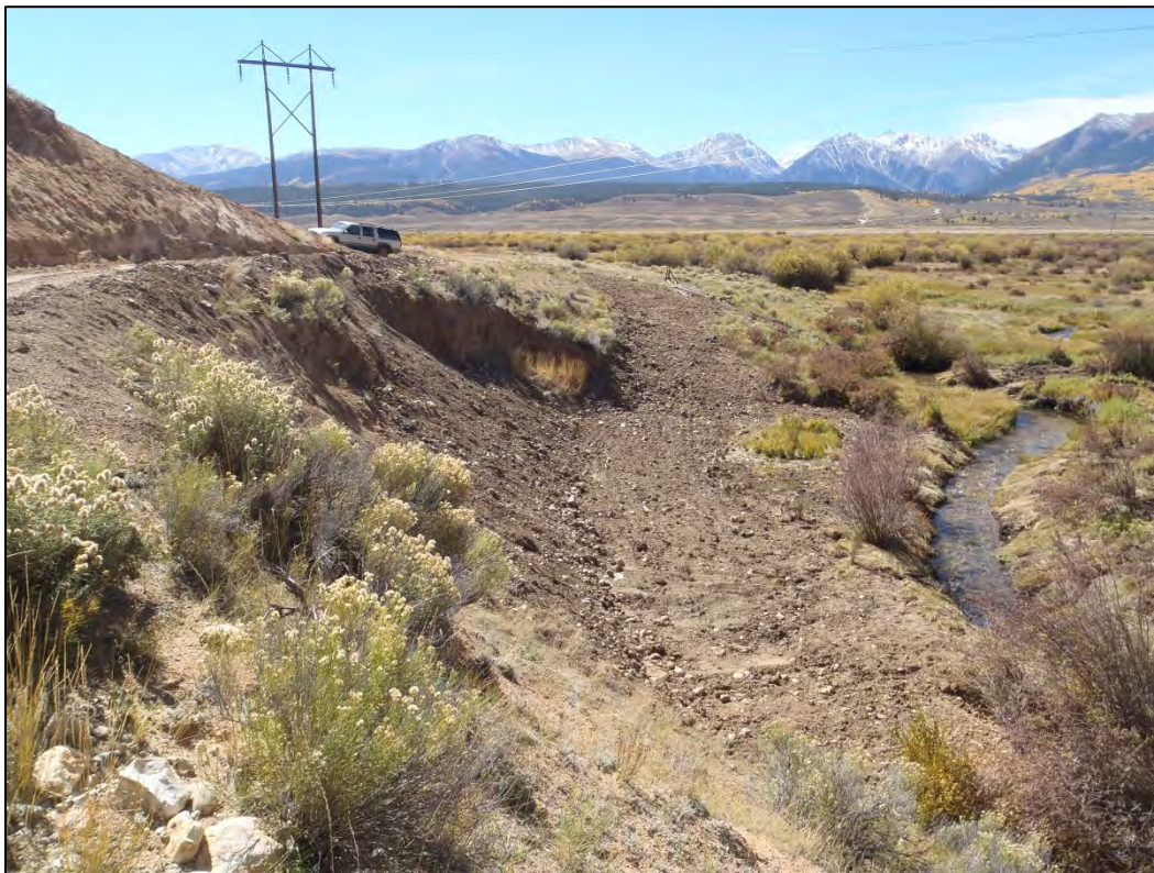
Figure 6. Photo Point 2 – Meander 2, post construction. Backfill is approximately 60% complete in this picture
