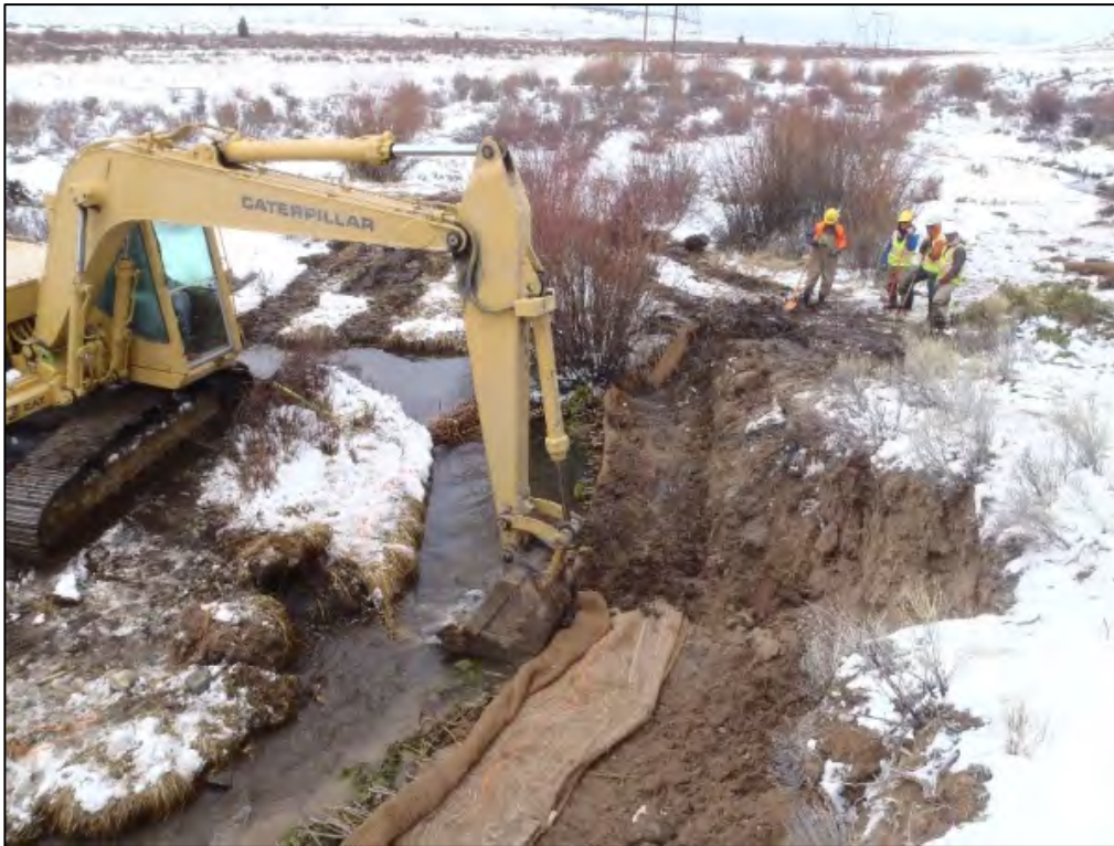
Figure 21. Soil Lift construction. April, 2013
