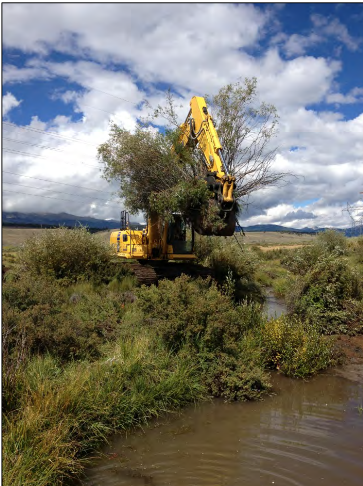
Figure 28. Relocating a willow to stabilize a new bank near Meander 2.
