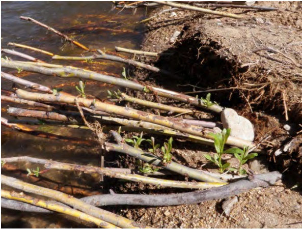
Figure 10. Soil lift willows after 8 weeks of growth.
