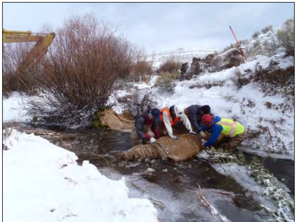
Figure 22. Soil Lift construction. April, 2013
