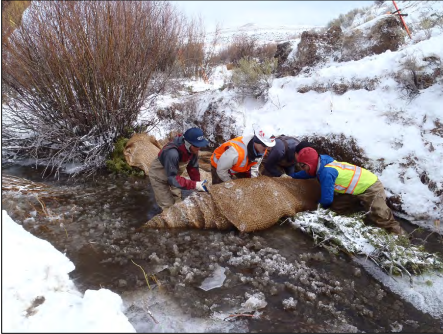
Figure 19. Rolling out Coir fabric on top of fascine.
