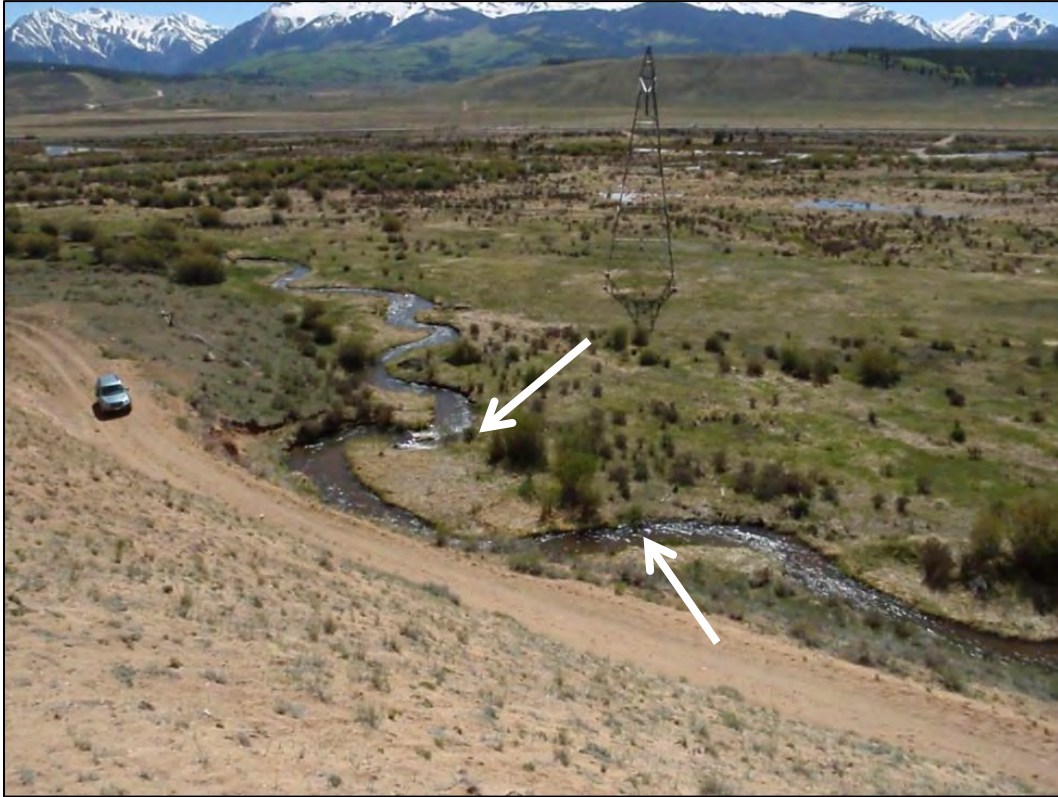
Figure 7. Location of channel realignment point of exit and re-entry. Pre-construction
