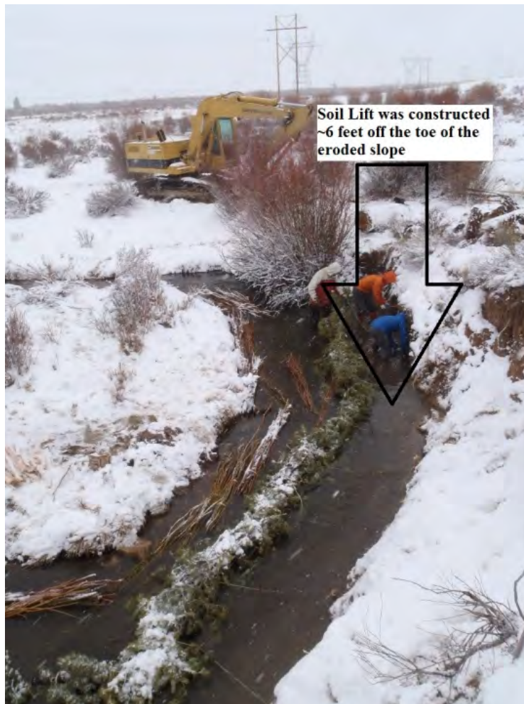
Figure 20. Soil Lift construction. April, 2013
