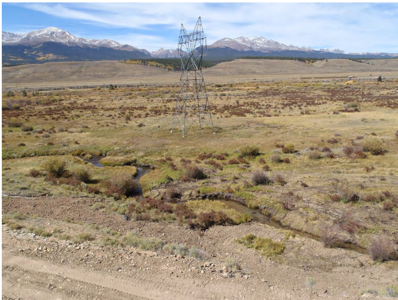
Figure 23. Completed channel realignment at Meander 2.
