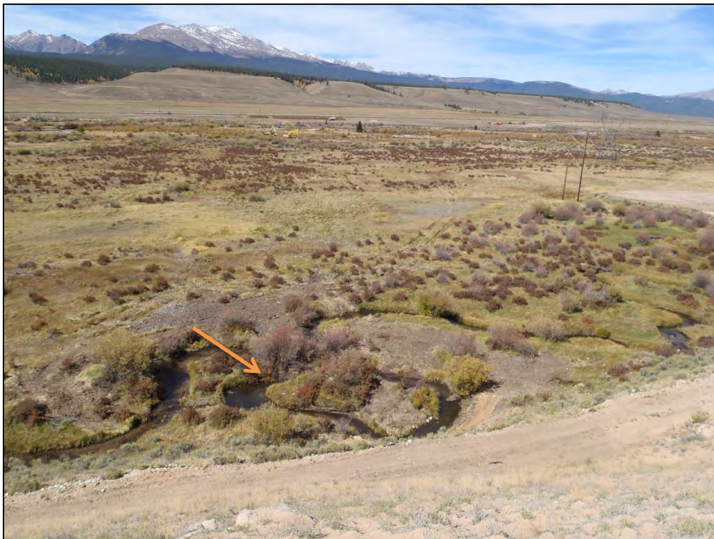
Figure 4. Photo Point 1a – Meander 1, Post Construction. Note closer of oxbow at orange arrow, new elevation control ripple is behind large transplant willow.
