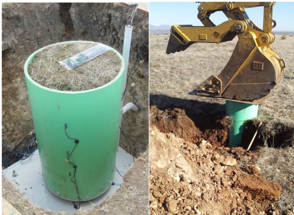
Figure 11 – Sterling Ranch Lysimeter and Soil Core
