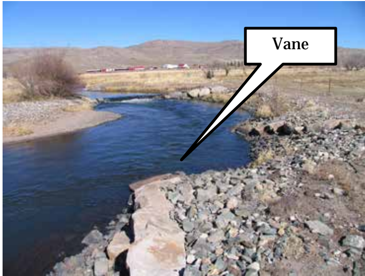
Figure 12. Examples of Vanes, Cross Vanes, Sills and Boulder Terrace.
