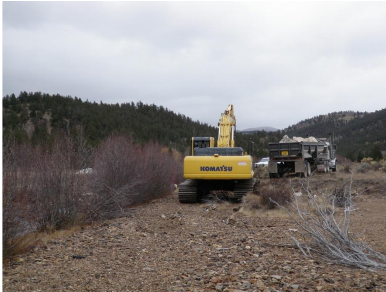
Figure 4.1: Excavator and truck containing limestone in-stream rock along Kerber Creek at KC 20
