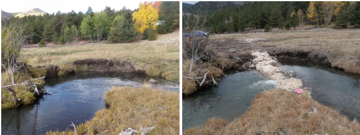
Figure 5.7: KC 20 Kerber Creek meander bend before restoration (left) and after installation of J-hook (right)
