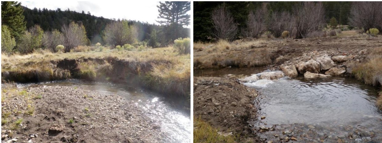
Figure 5.6: KC 20 Kerber Creek cutbank before restoration (left) and after J-hook installation and reshaping (right)
