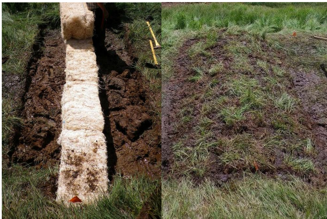
Figure B-4: installation of a Ditch 3 Excelsior bale dam (July 20, 2012)
