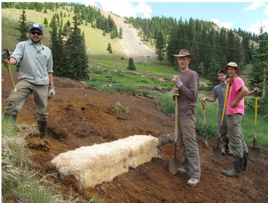
Figure B-22: installing Excelsior bale erosion controls with MSI staff, interns and a visually impaired student volunteer from University of Colorado (July 11, 2012)
