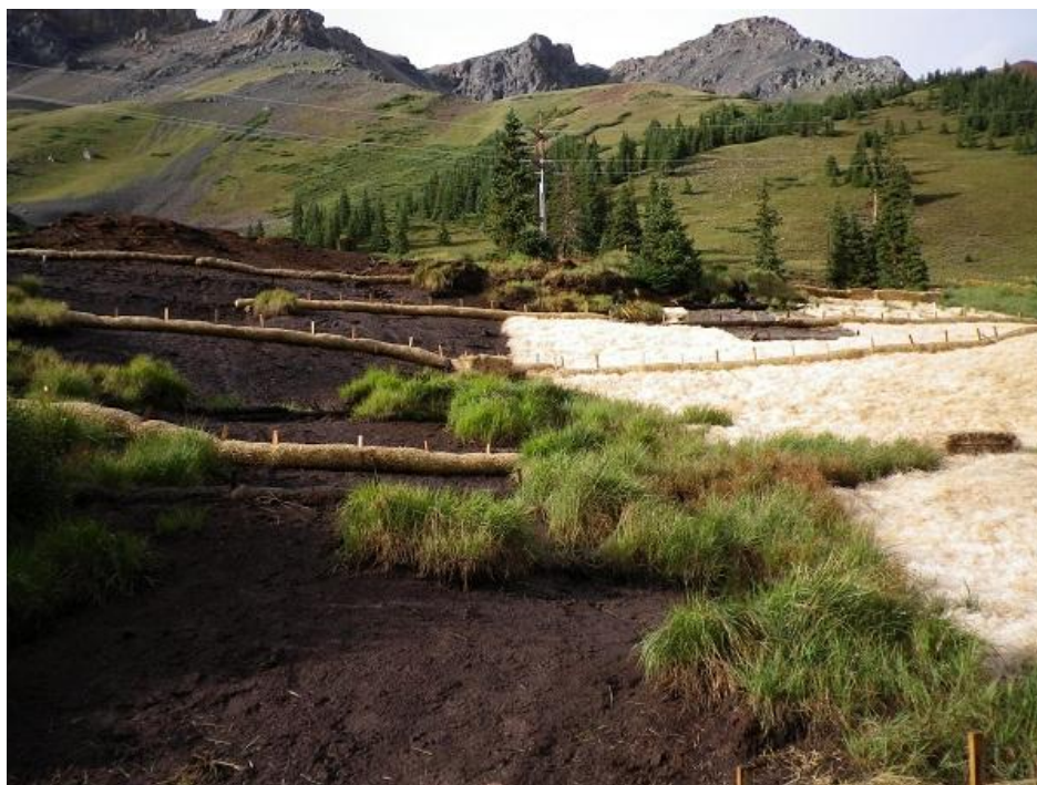
Figure B-12: looking north and upslope at the steep bare area after grading occurred and wattles and partial mulch were laid (August 9, 2012)
