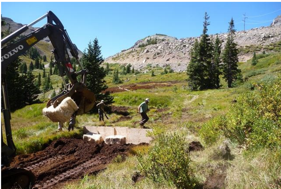
Figure B-20: AJ Construction installing a plywood dam and excelsior bales in Ditch 6 (September 5, 2012)
