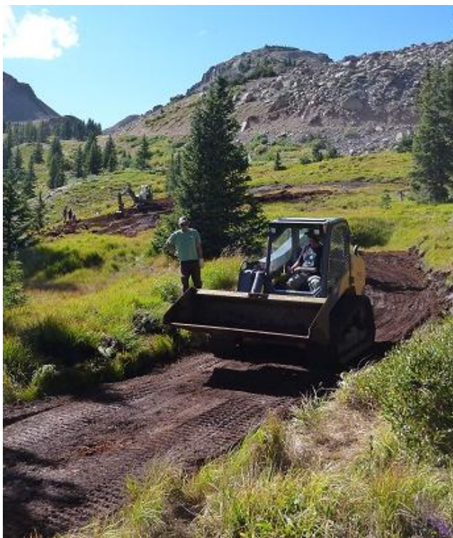
Figure B-19: AJ Construction filling Ditch 6 with material from the large bare area (September 4, 2012)
