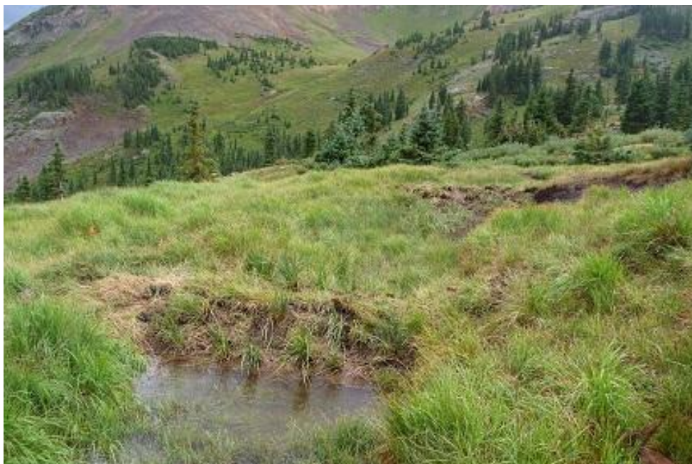
Figure B-9: Ditch 3 Excelsior bale hams holding water (August 2012)
