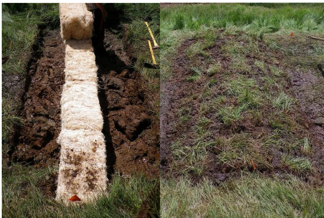
Figure B-8: installation of a Ditch 3 Excelsior bale dam (July 20, 2012)
