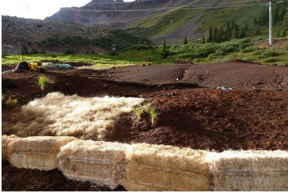
Figure B-14: looking north and upslope at the western mineralized mound on the large bare area (background). The bales in foreground are the erosion control installed to catch sediment from heavy equipment construction (August 1, 2012)
