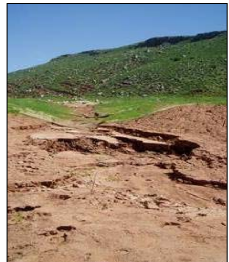
Storm damaged inlet
