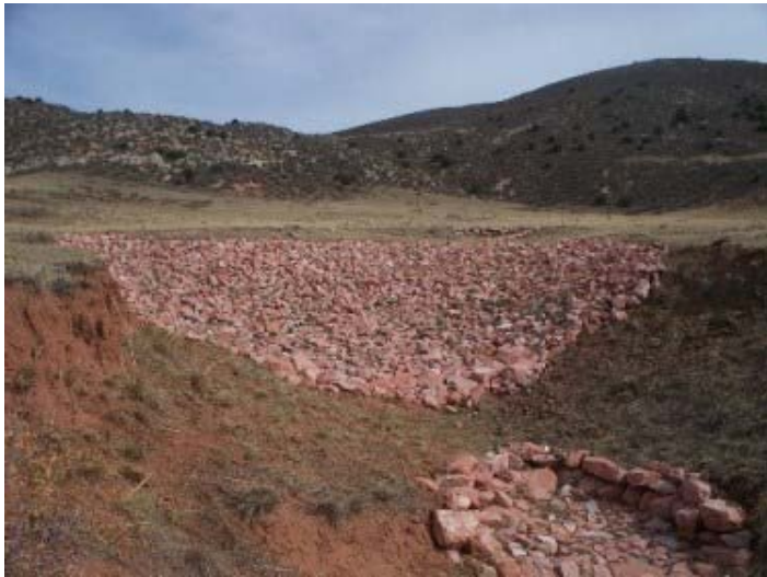
Regraded and rock ramped headcut. This experimental treatment was done with all hand labor. Future treatments be regraded using an excavator.
