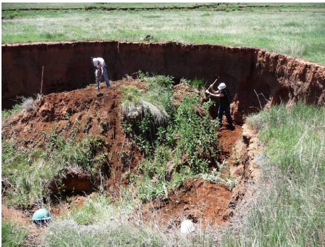
Regrading soil pillars by hand to reduce snow-based saturation points near headcuts and the base of valley walls. Additional grading was completed by excavator.
