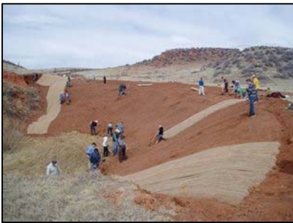
Volunteers installing erosion mat on fill slope from dam material
