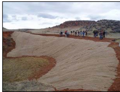
Volunteers installing erosion mat on fill slope from dam material
