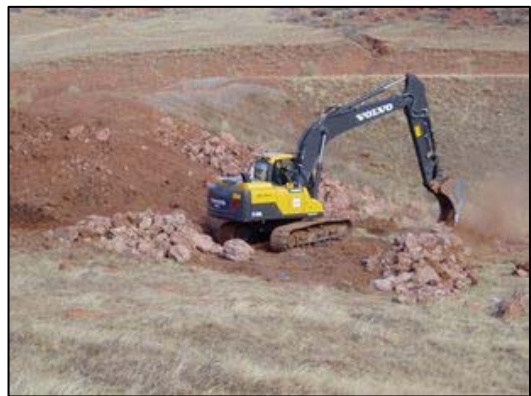
Installation of grade control structures
