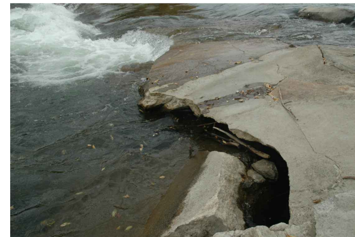
BOULDERS SEPARATED FROM STRUCTURE & UNDERCUTTING - RIVER LEFT SHOULDER
