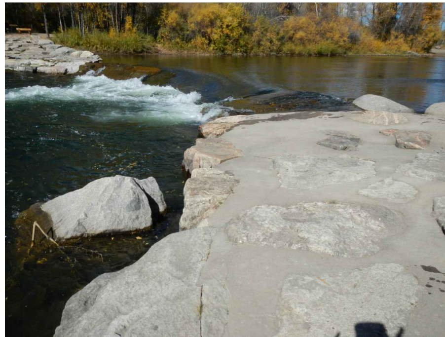
BOULDERS SEPARATED FROM STRUCTURE - RIVER LEFT SHOULDER PHOTO F2-3 NO SCALE
