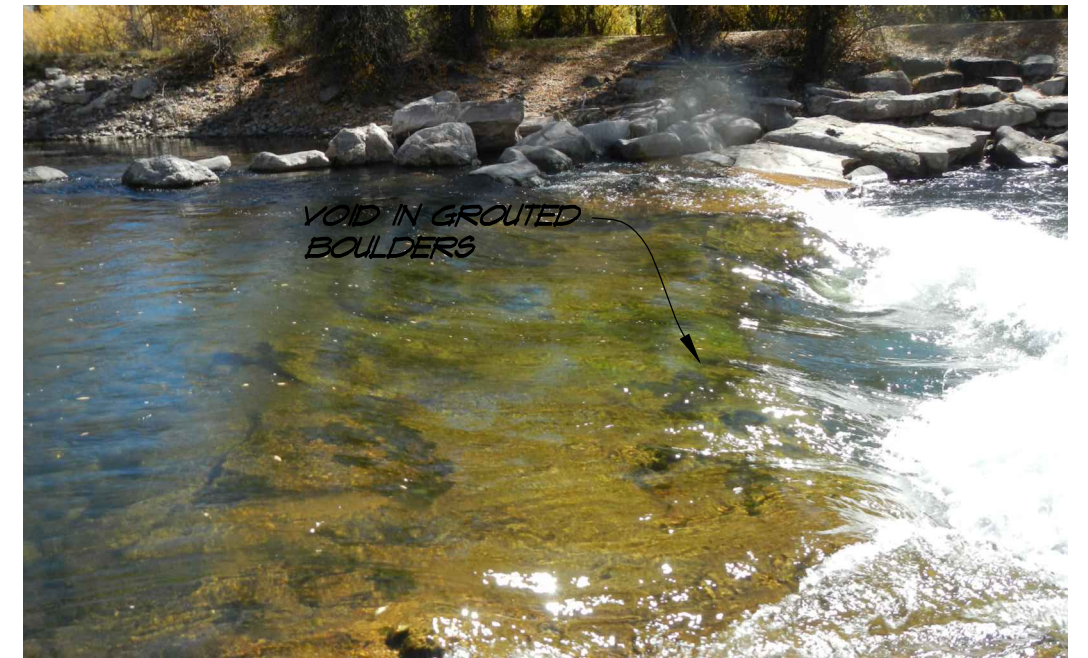
VOID IN GROUTED BOULDERS - BOAT CHUTE
