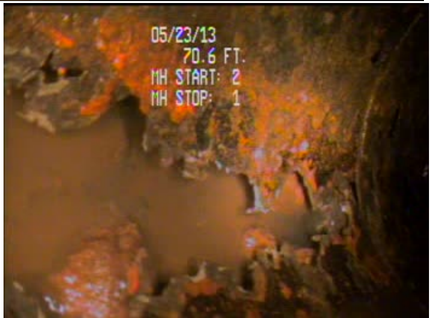
Figure 5 – Overall view of missing invert at 70.6 ft. (note that view is rotated 90 degrees).
