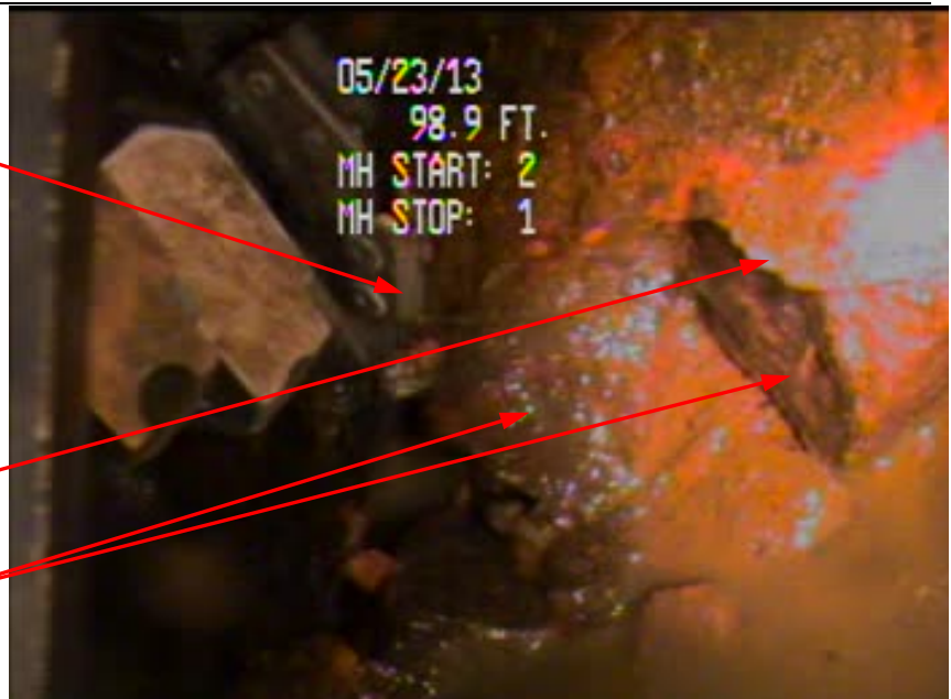
Figure 11 – Close-up of left (looking upstream) ROV track near downstream end of missing invert section.
