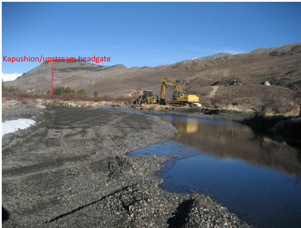
Post work gravel bar blended into west bank
