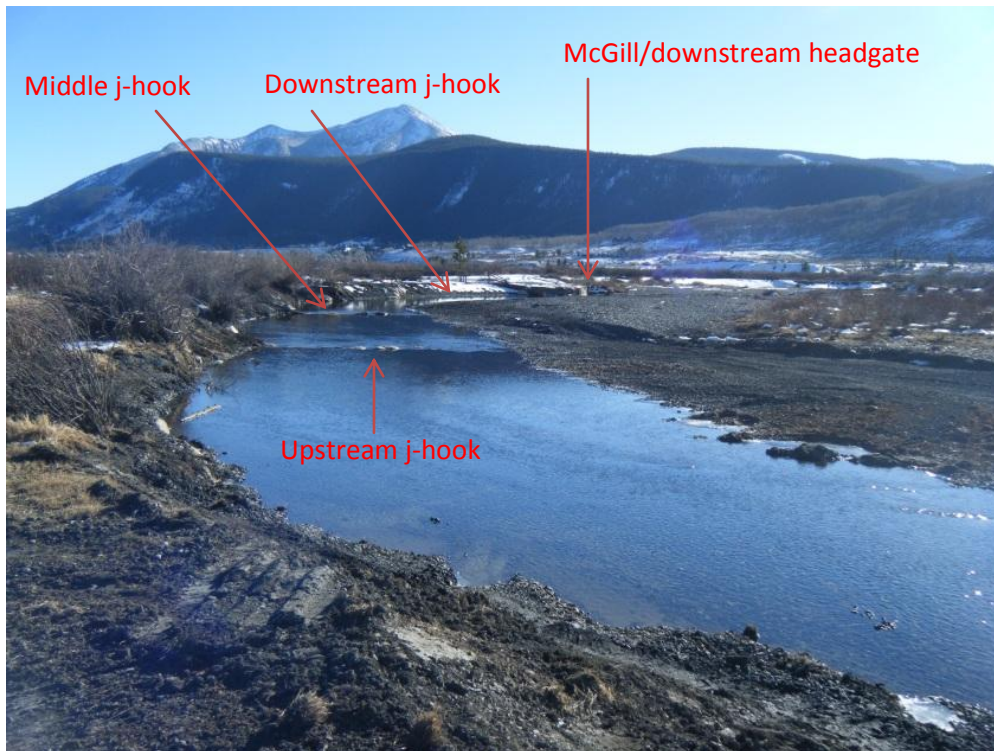
Post work view of restored bend and j-hooks
