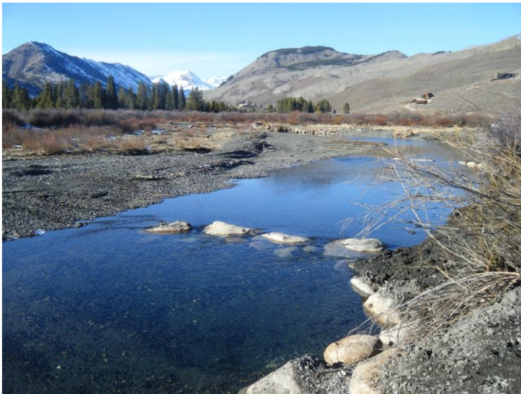
Post work view of middle and upstream j-hooks
