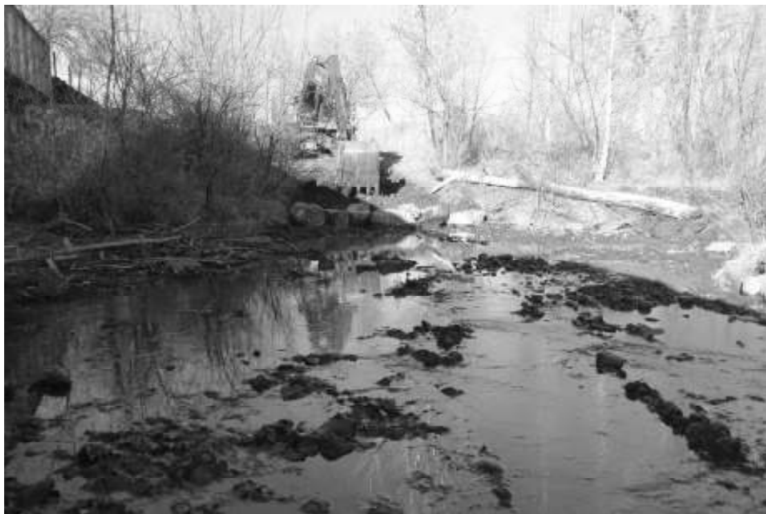
Photo 5: Closing and Rehabilitating a Motorized Access Route to the River.
