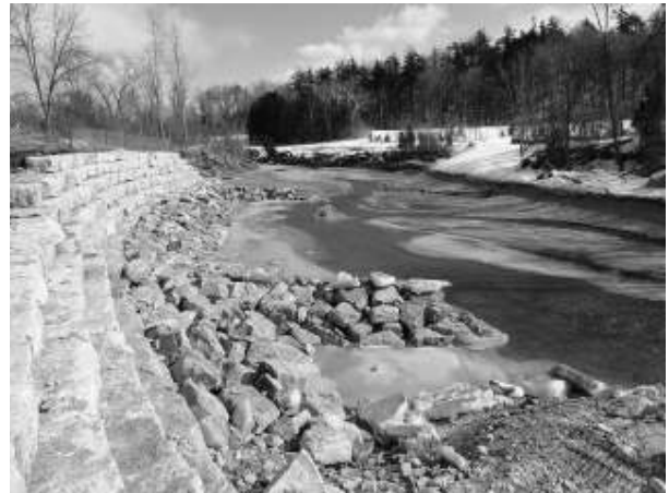
Photo 2: Example of Bendway Weirs & River Bank Revetment
