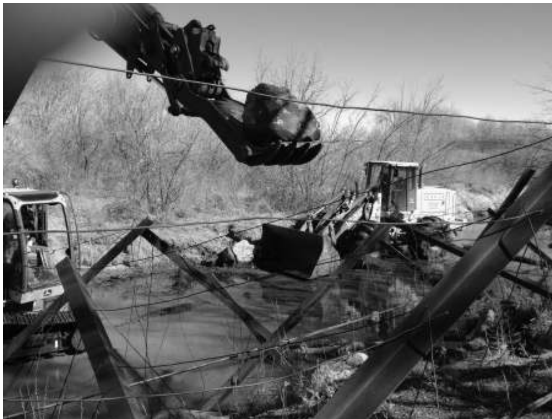
Photo 3: Utilizing innovative techniques to install vanes around the existing Jetty Jacks.
