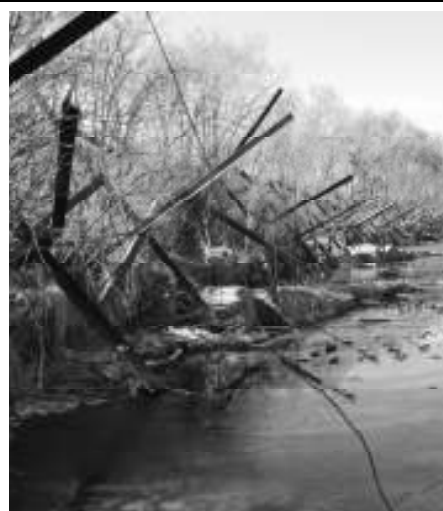
Photo 4: Completed J-Hook & Boulder Vanes adjacent to the Jetty-Jacks.
