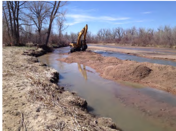
Photos 3 & 4. Cofferdam Excavation 4/9/14
