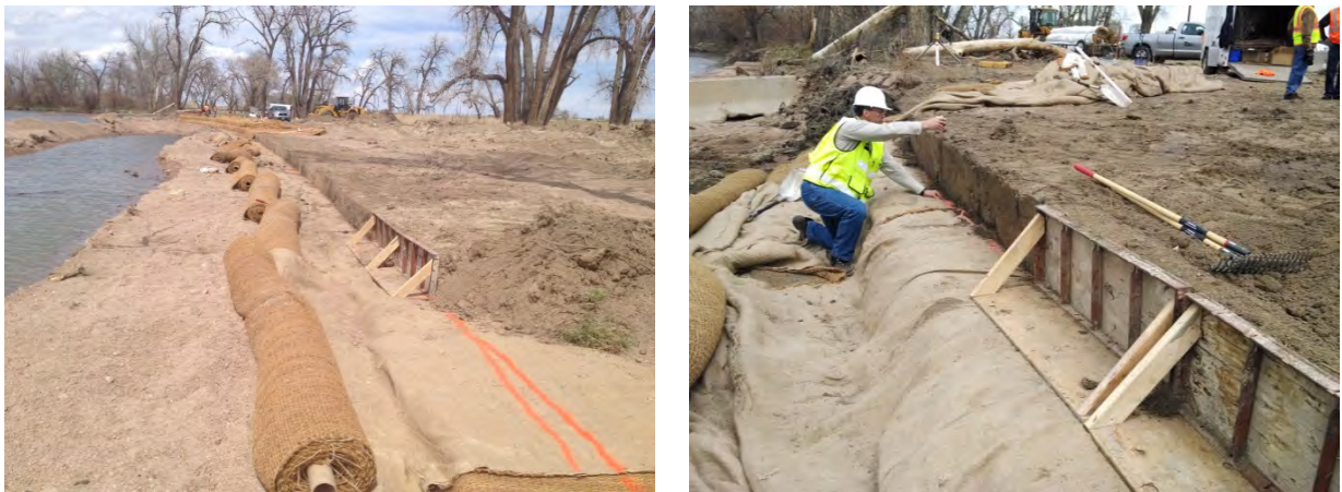
Photo 21. Batter Board and Final Installation of KoirWrap Blanket 5/2/14
