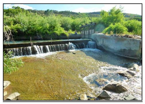
The Highland Ditch Company has diverted irrigation water from the White River since the 1880's. The headgate design allows fish to become entrained in the Ditch and the diversion structure prevents fish migration during irrigation season. This proposal is to redesign the diversion structure and headgate to include a fish screen that ensures the ditch can divert their full 250cfs water right without negatively impacting water operations or fish.
