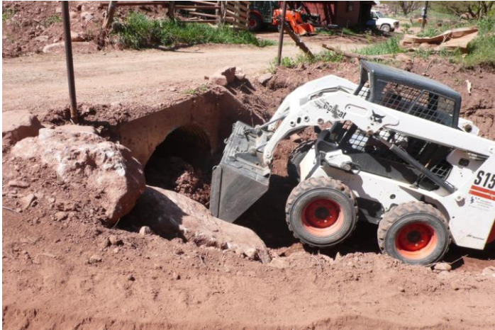
Bobcat and “handdiggers” cleaning out culverts.
