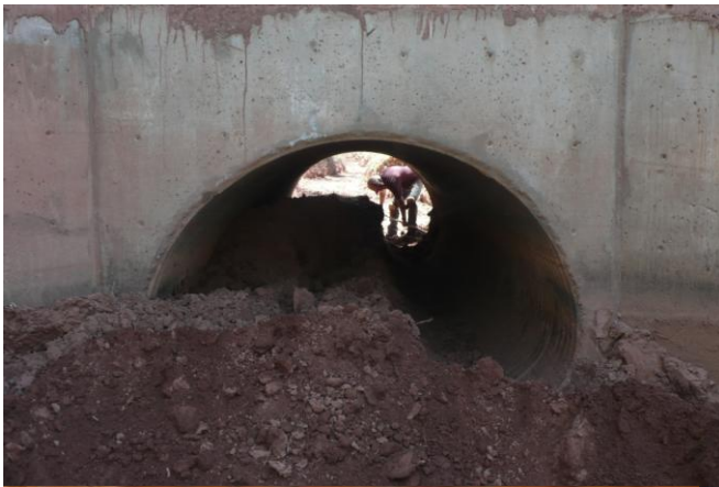
Bobcat and “handdiggers” cleaning out culverts.
