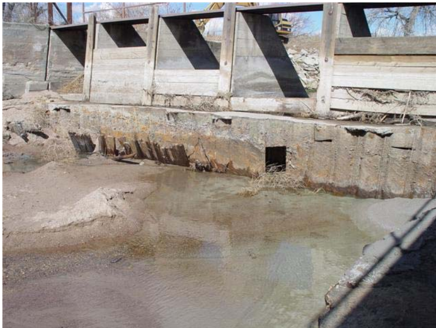
PHOTO 4 – CANAL HEADGATE BLOWOUT AREA
