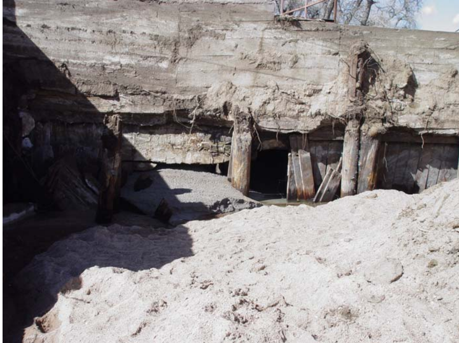
PHOTO 3 - LEFT (NORTH) ABUTMENT BLOWOUT
