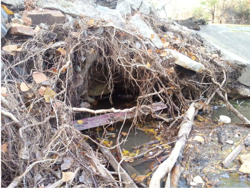
Photo 5 Scour hole to the south side of the Diversion Dam
