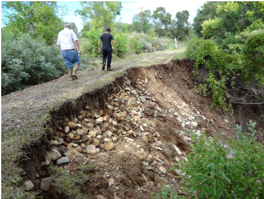
Photo 4 September 16, 2013 Outer Ditch Embankment Slide
