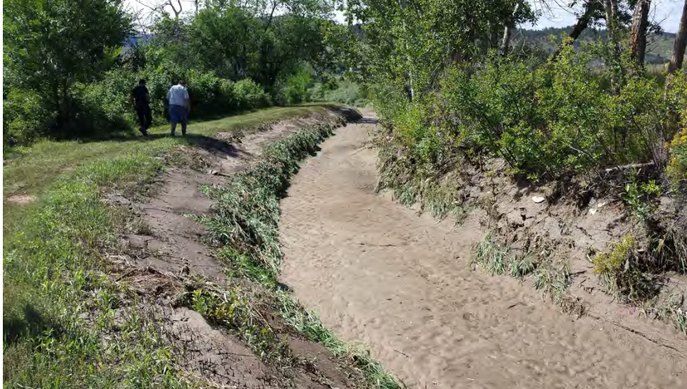
Photo 5 September 16, 2013 Typical Sediment Build Up
