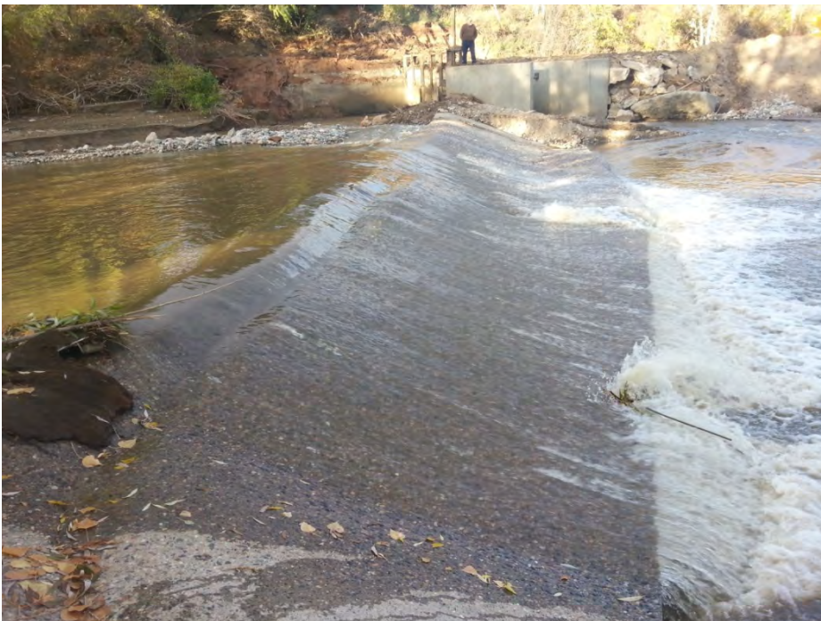
Photo 4 Diversion Dam Damage and Undercut Toe
