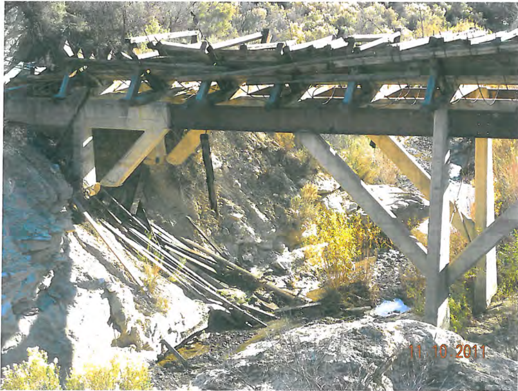
Supports at southern end of McElmo Creek Flume where bank has eroded away (Photo by Linda Towle)
