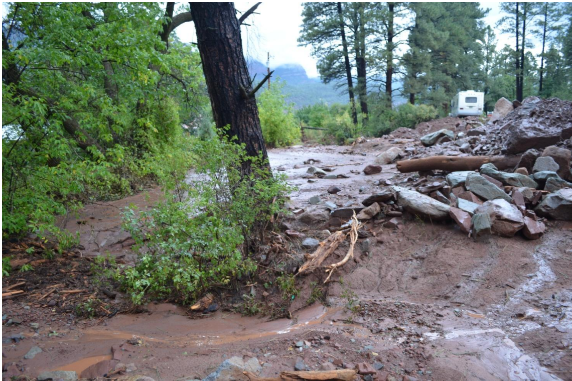
Debris filled in and overflowed ditch
