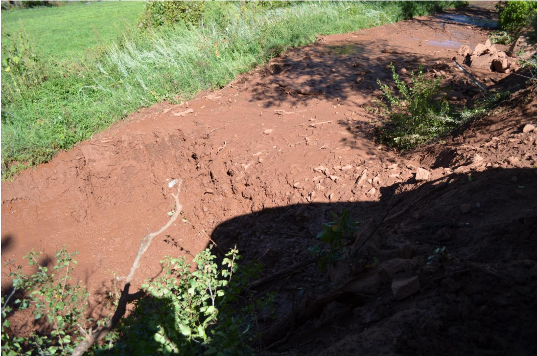
4 feet of mud and rock in ditch; ditch protected private property in this case
