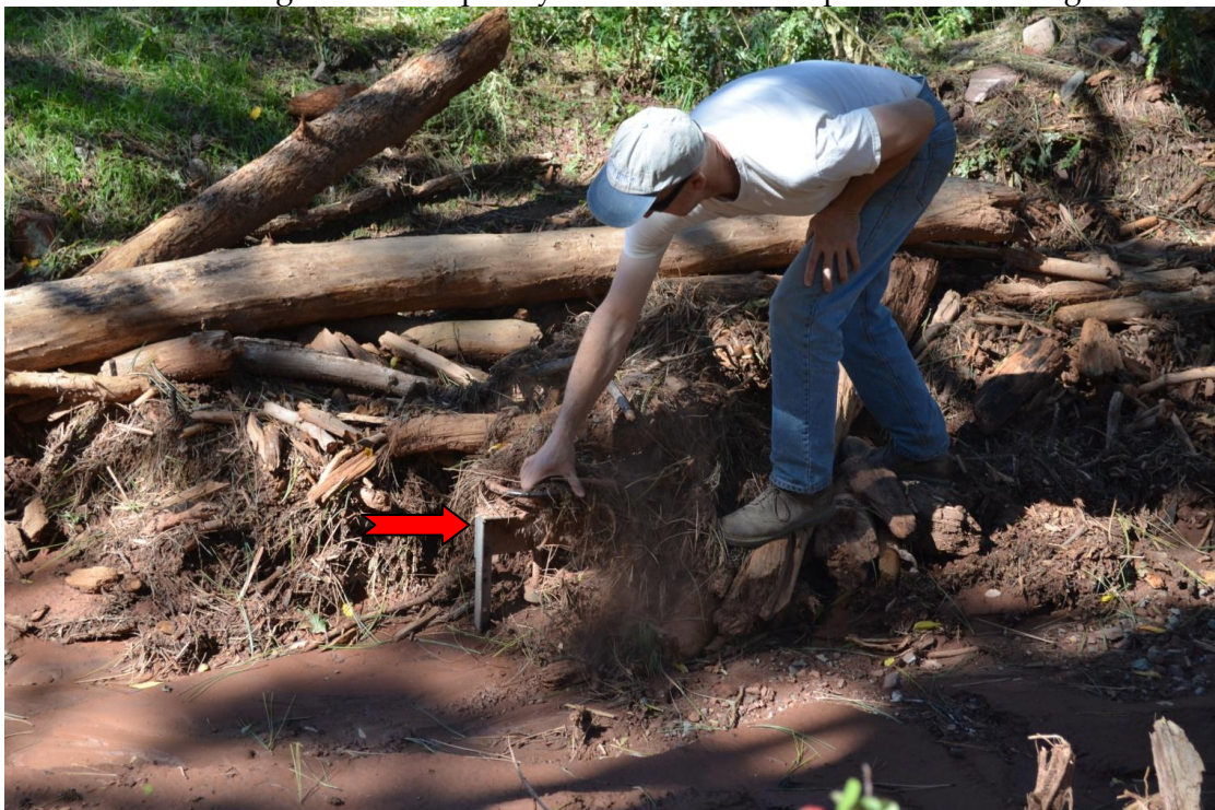
Private headgate totally buried in debris
