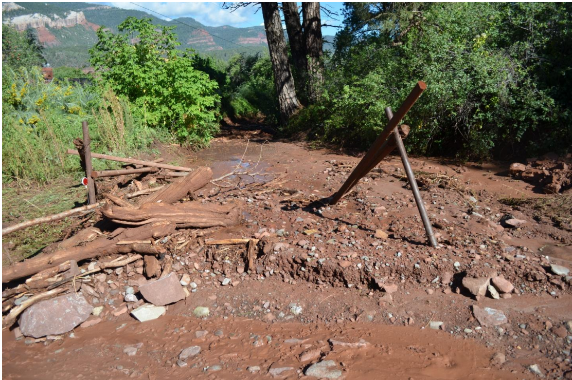
Buried ditch crossing – ditch completely filled and took out private ditch bridge
