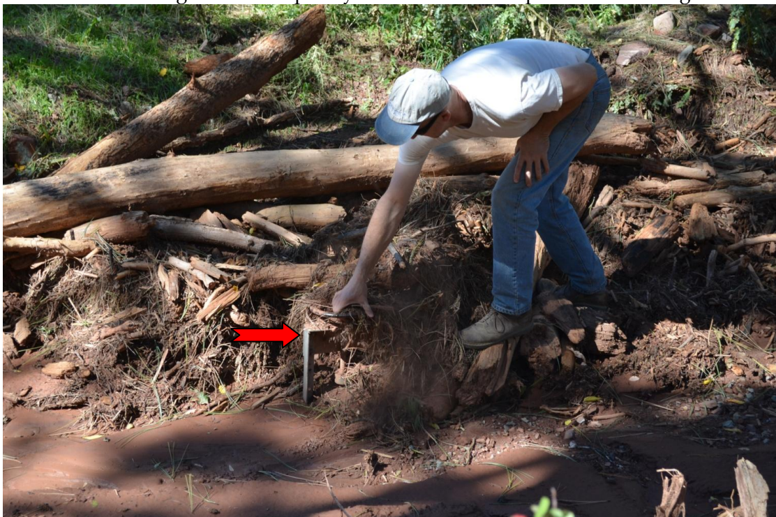
Private headgate totally buried in debris
