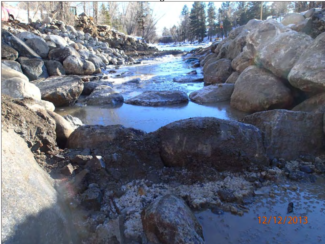
Fish Passage Weirs 1-3
