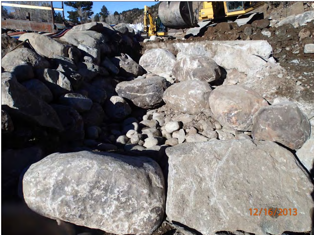
Fish Passage Weirs 6-8
