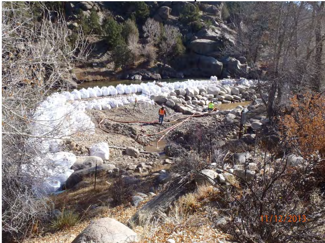
Coffer Dam and Drop #1
