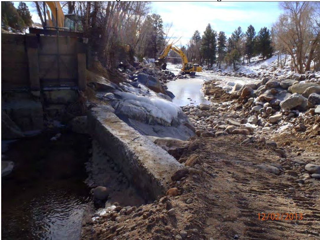
Existing Diversion Weir and Headgate
