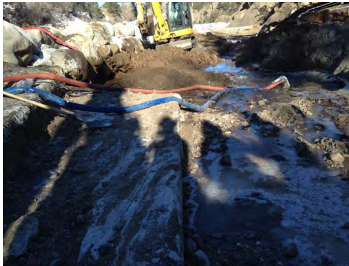
Existing Concrete Weir Wall & Upstream Slab
