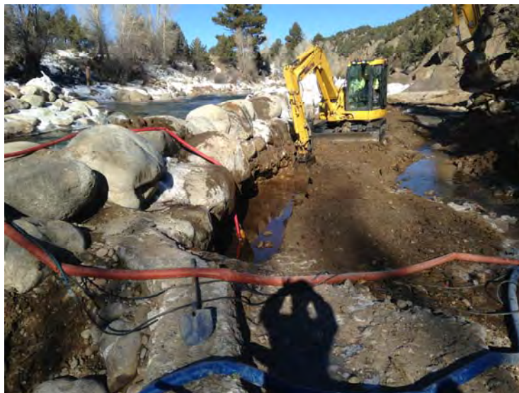
Existing Concrete Weir Wall & Upstream slab, grout curtain trench
