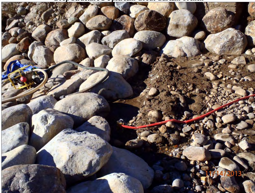
Drop Structure 2 Upstream Grout Curtain Trench
