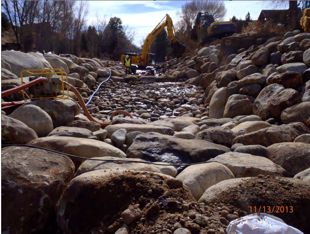
Drop Structure 1, Pool 1, and Drop Structure 2 Looking Downstream
