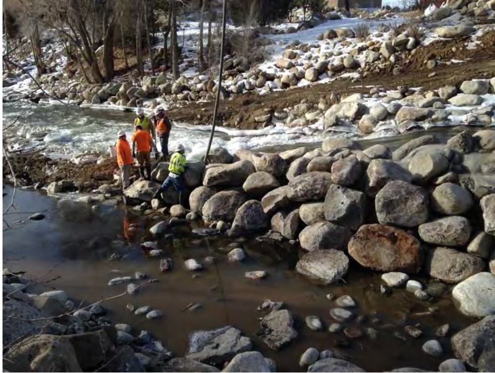
Grout Placement Divider wall Downstream Weir Wall
