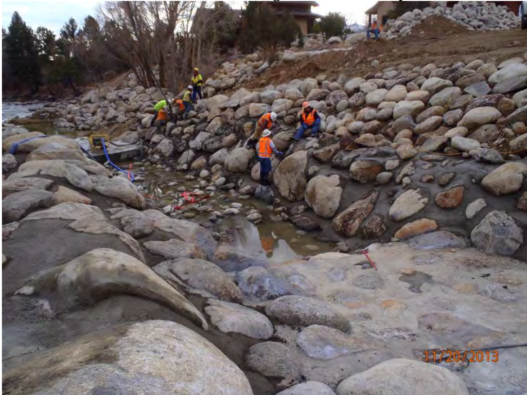
Grout Placement River Right Bank Above Drop 3
