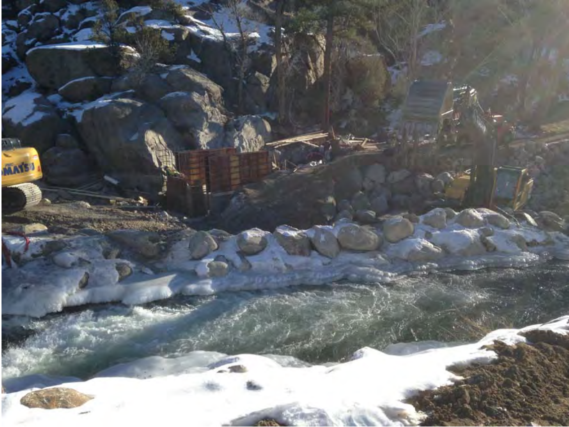
Concrete Forming Headwall & Walls Phase 1
