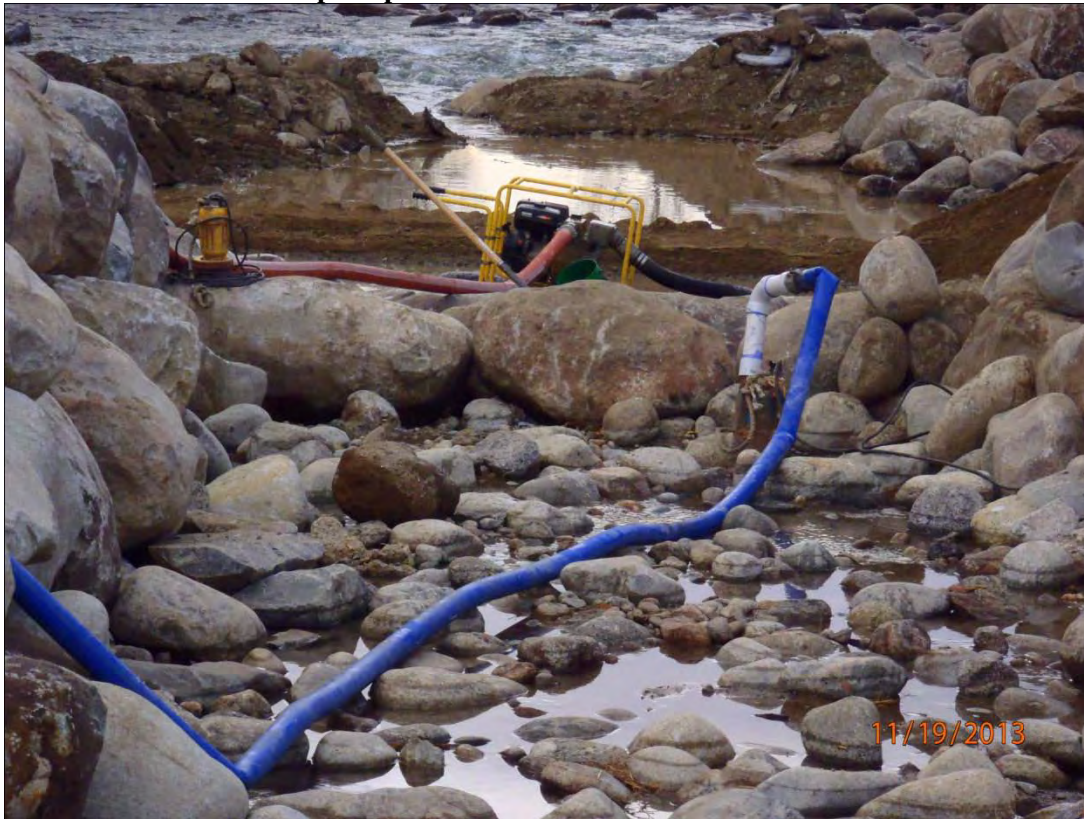
Drop 3 Upstream Prior To Grout Placement
