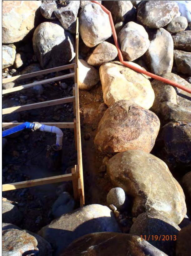
Drop 3 Upstream Grout Curtain Form
