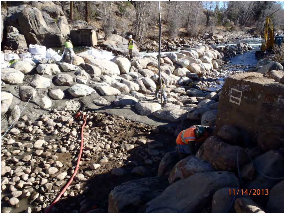
Placing Grout Drop 2
