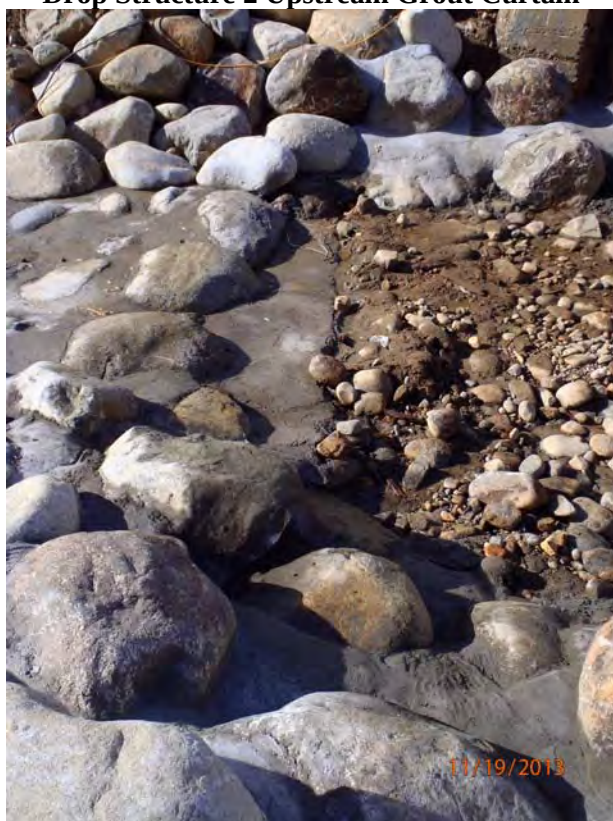
Drop Structure 2 Upstream Grout Curtain
