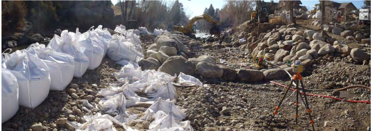
Drop #1 Looking Downstream
