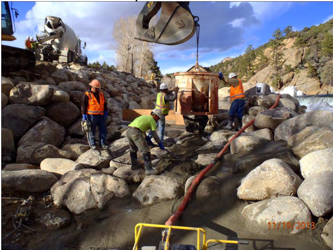
Drop 3 Grout Placement
