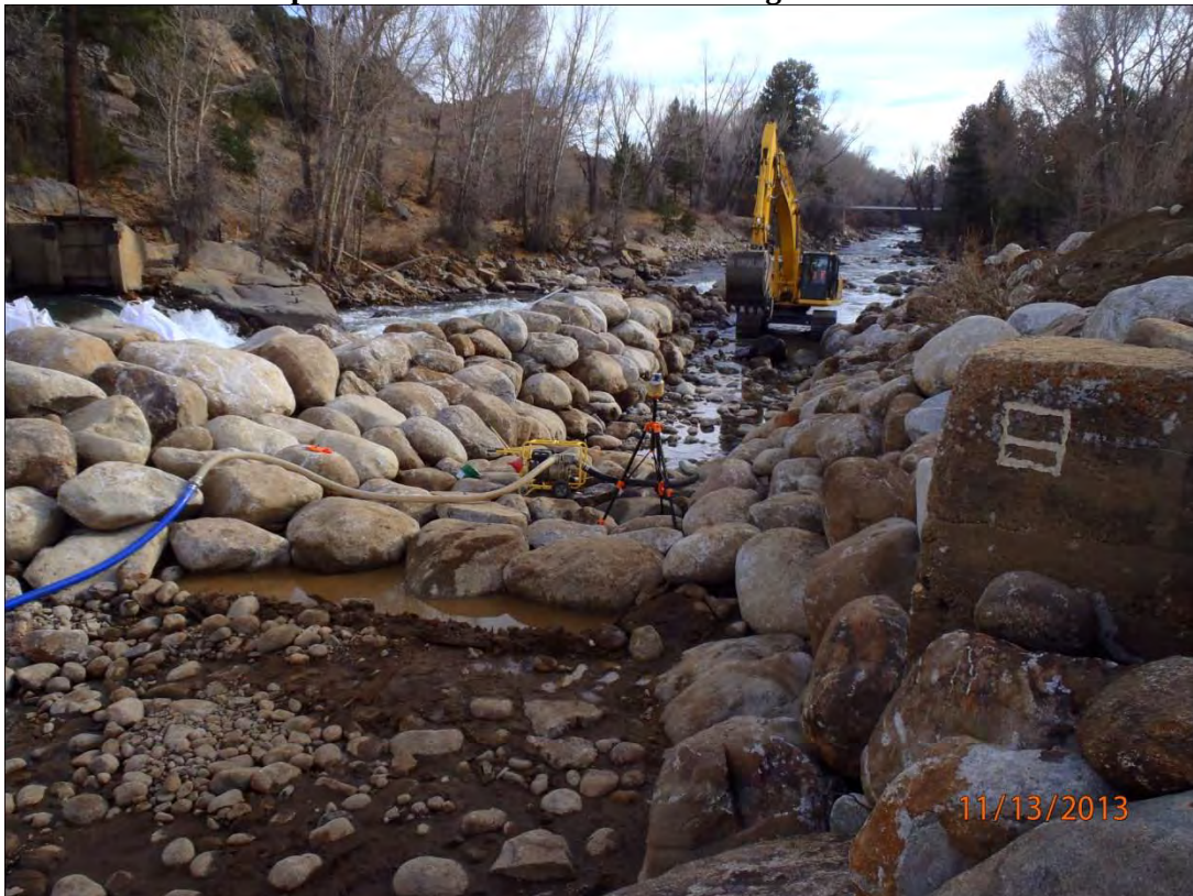
Drop Structure 2 and Channel Looking Downstream
