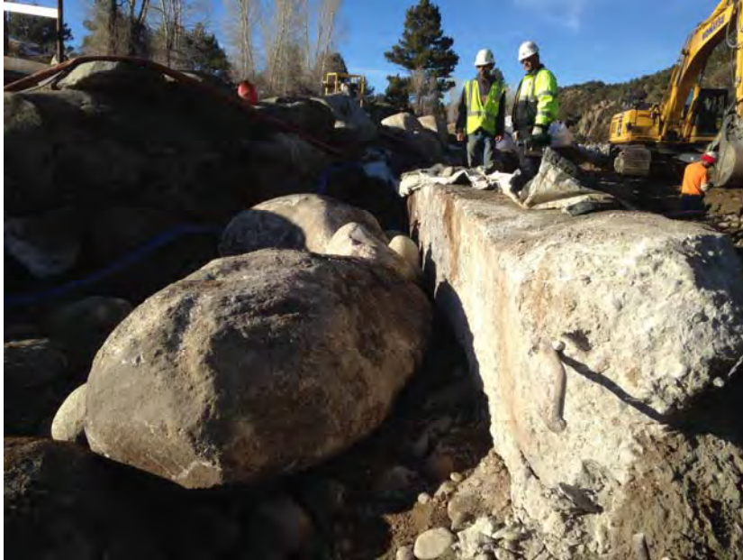
Existing Concrete Weir Wall
