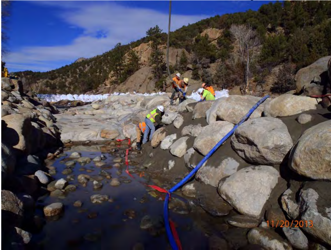
Grout Placement On Divider Island Below Drop 2
