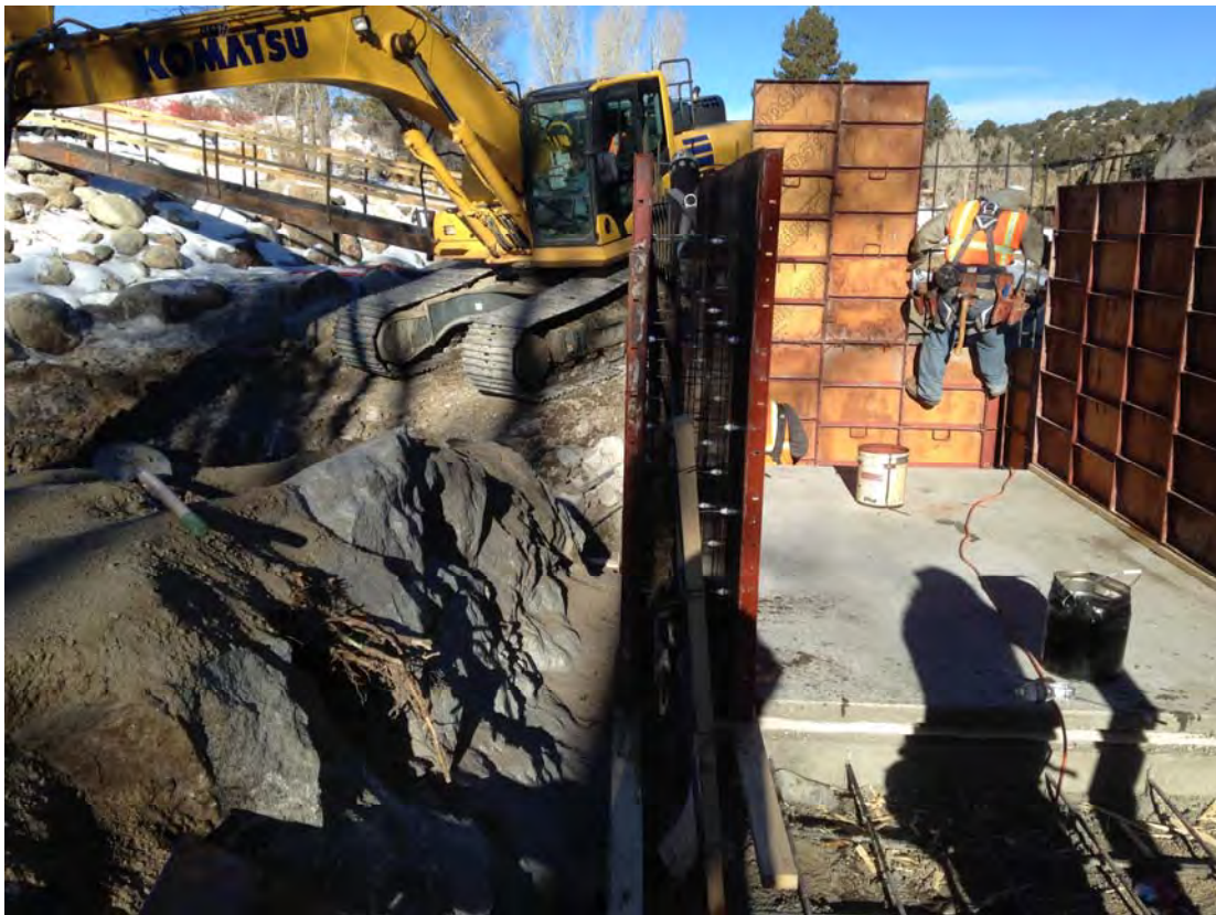
Phase 1 Walls Forming
