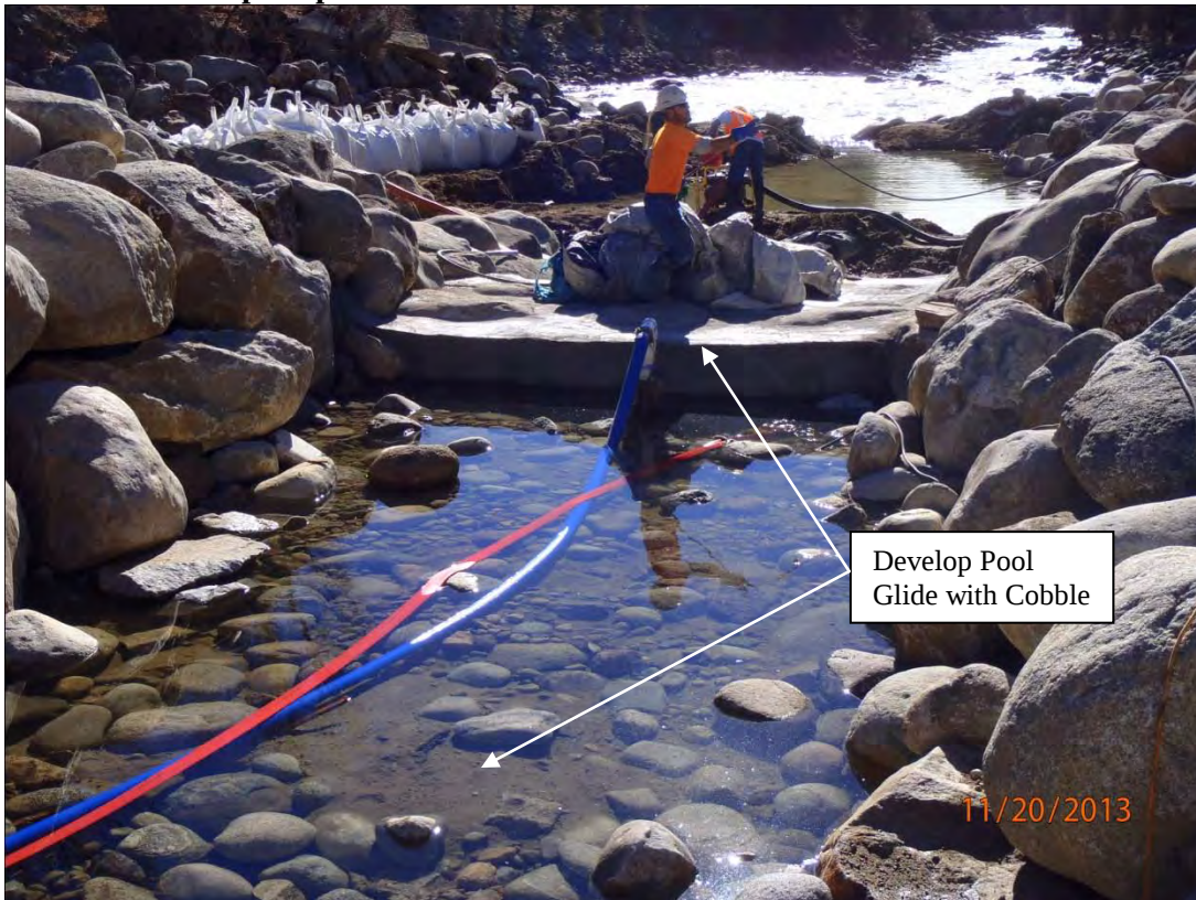
Drop 3 Upstream Post Grout Placement and Form Removal
