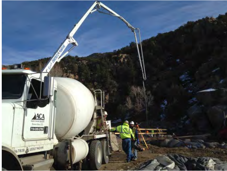
Grout Delivery and Pumper
