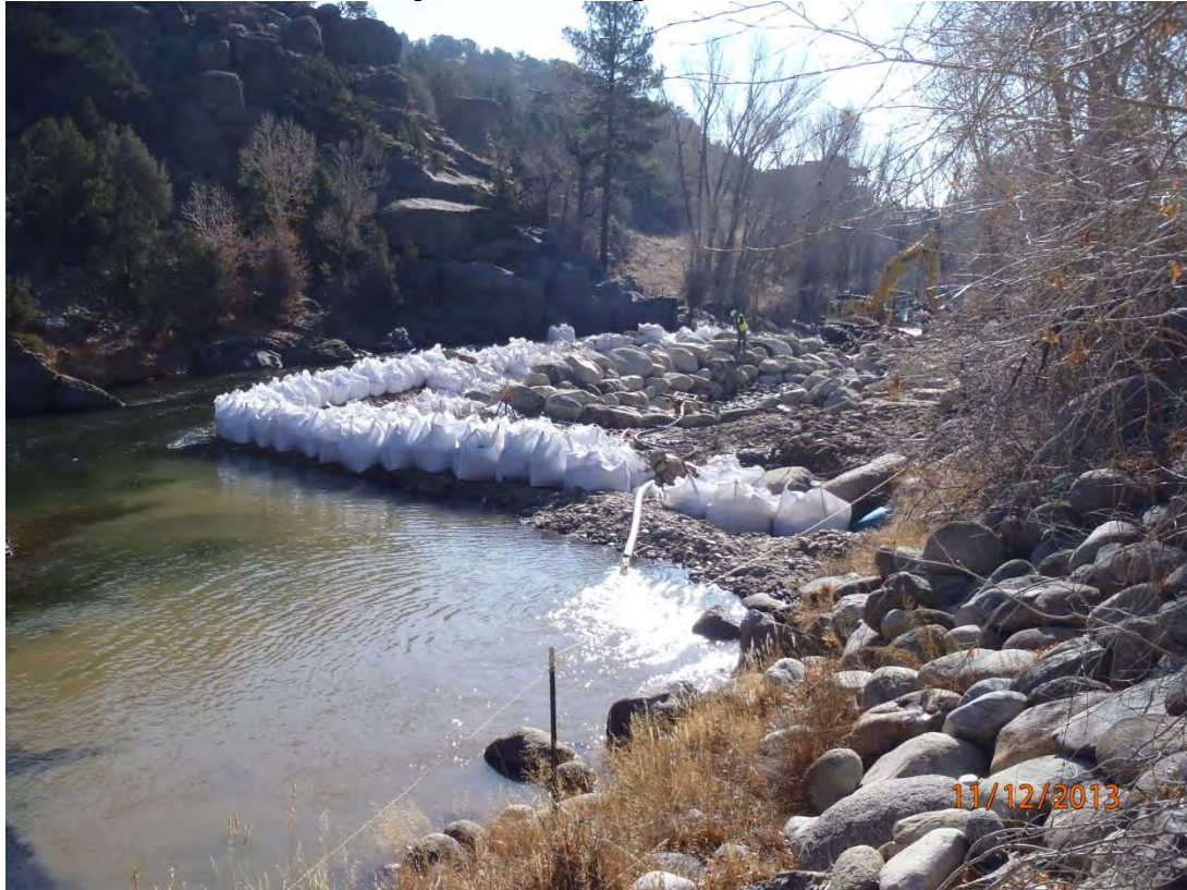
Project Site Looking Downstream
