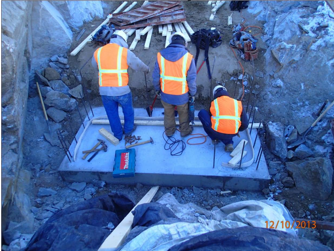
Floor of Headgate
