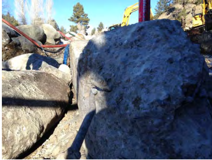
Existing Concrete Weir Wall
