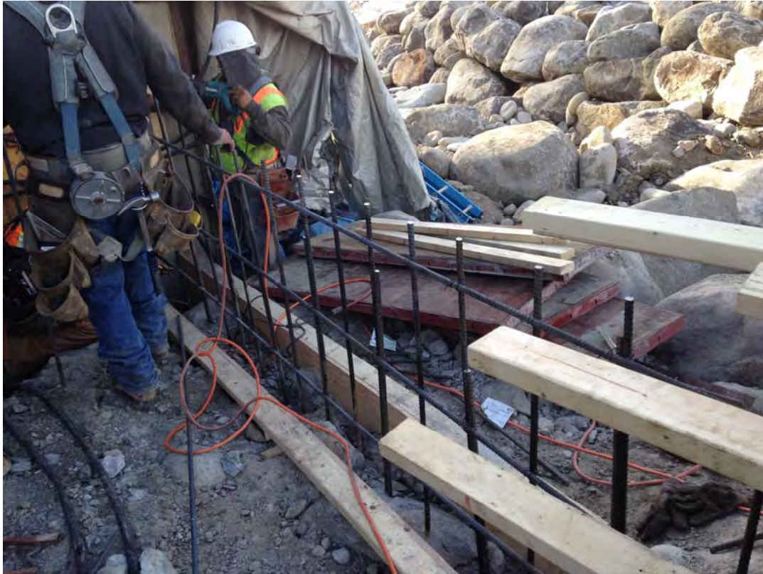
Weir Wall Phase 1
