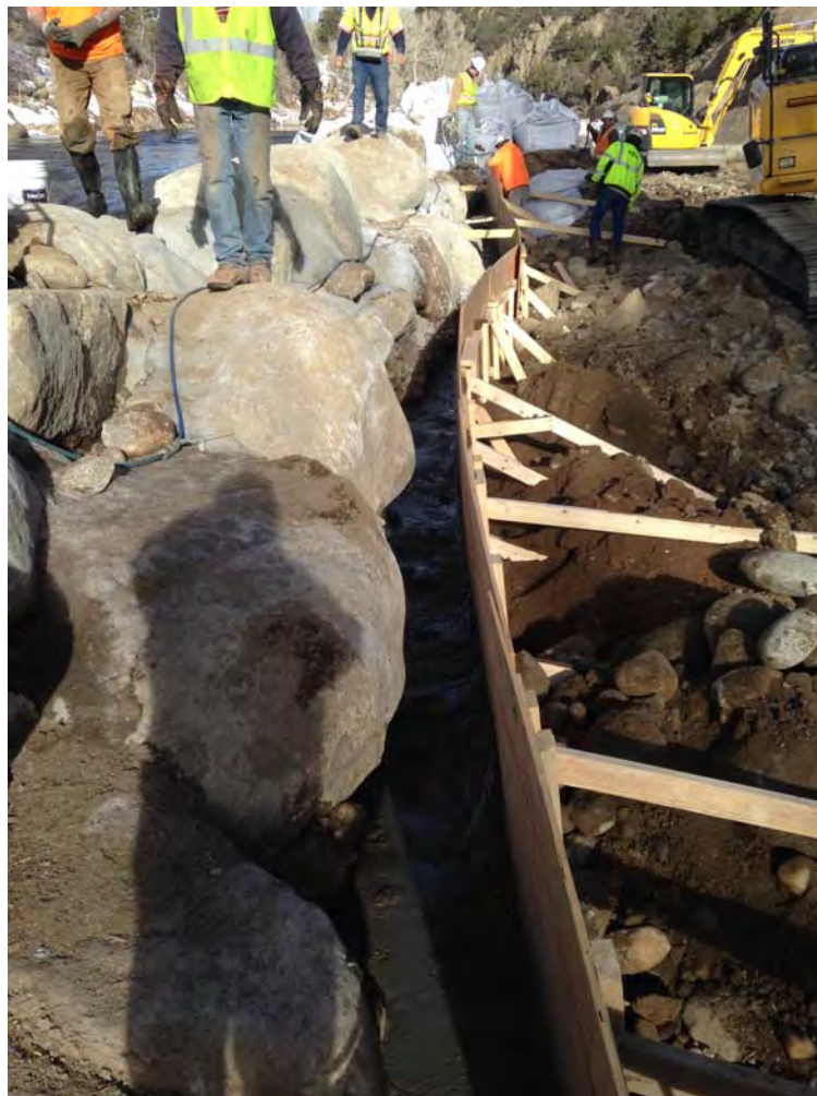
Grout Curtain along Divider wall Upstream Weir Wall
