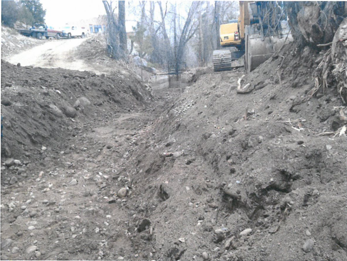
Excavating Ditch between Phase II and Downstream Bypass Structure
