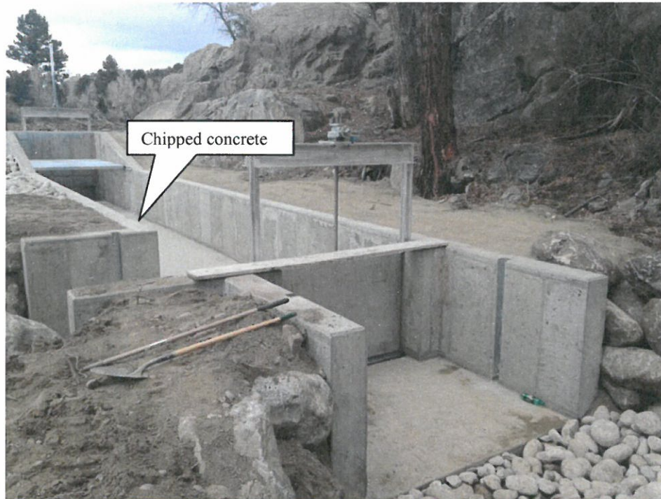
Phase II Concrete Channel & Gate
