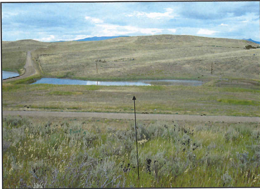
Photograph 3. Photograph Point 5 – Looking north at M3 (9/10/2008).
