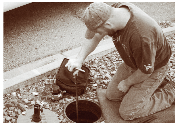
St Charles employee installing a new radio read water meter
