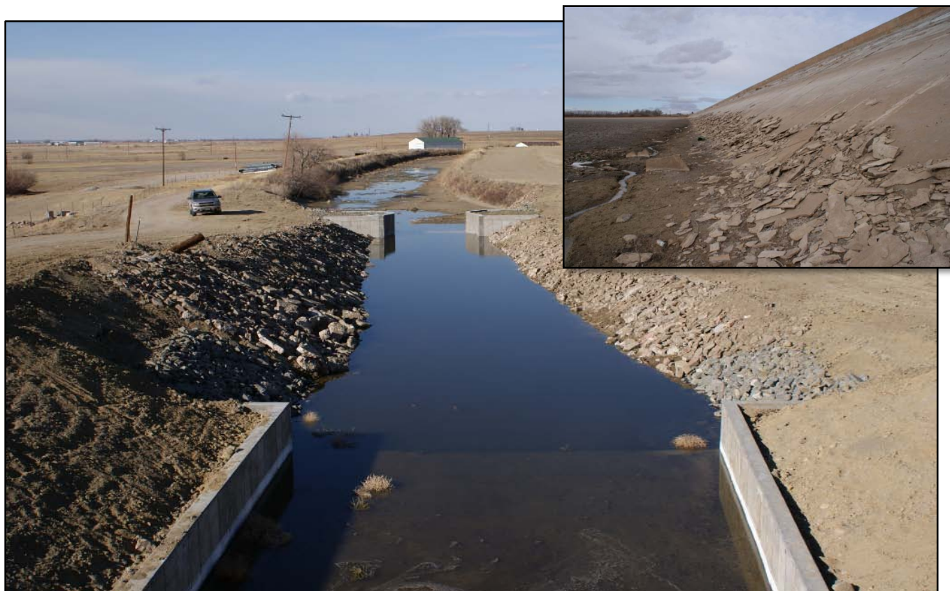
Prospect Reservoir Dam pre-project debris (inset) and the rehabilitated Horse Creek Reservoir outlet flume
