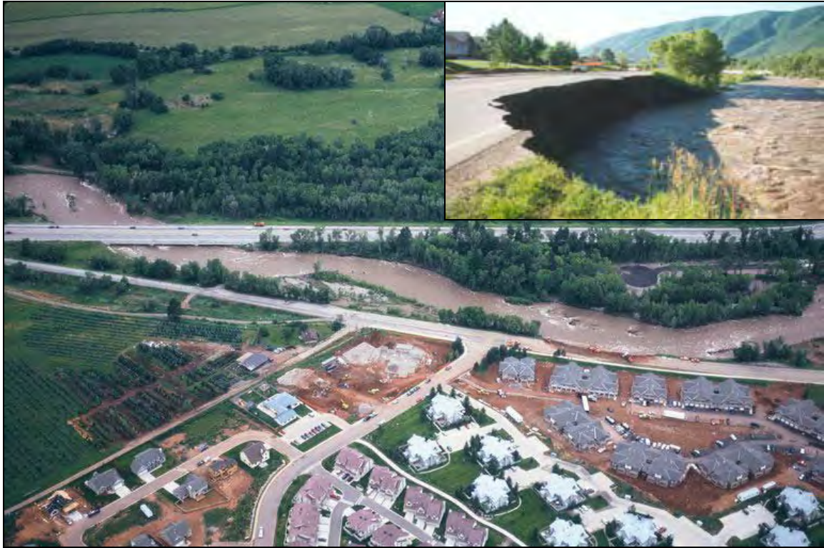
The photograph above is an aerial view of the flooding that occurred in 1995. The inset photograph is a close-up of the eroding bank and collapsed Two Rivers Road.
