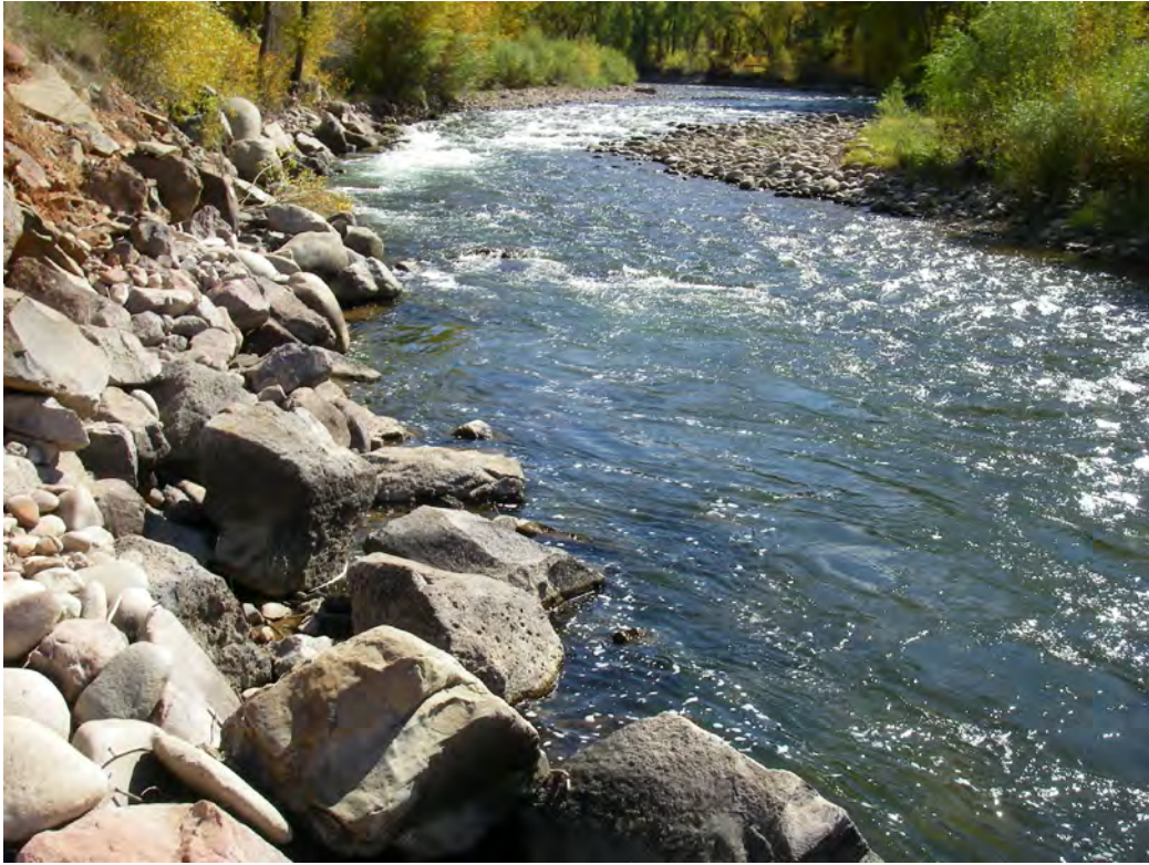
Photo No.3 Looking upstream towards location of upstream structure.
