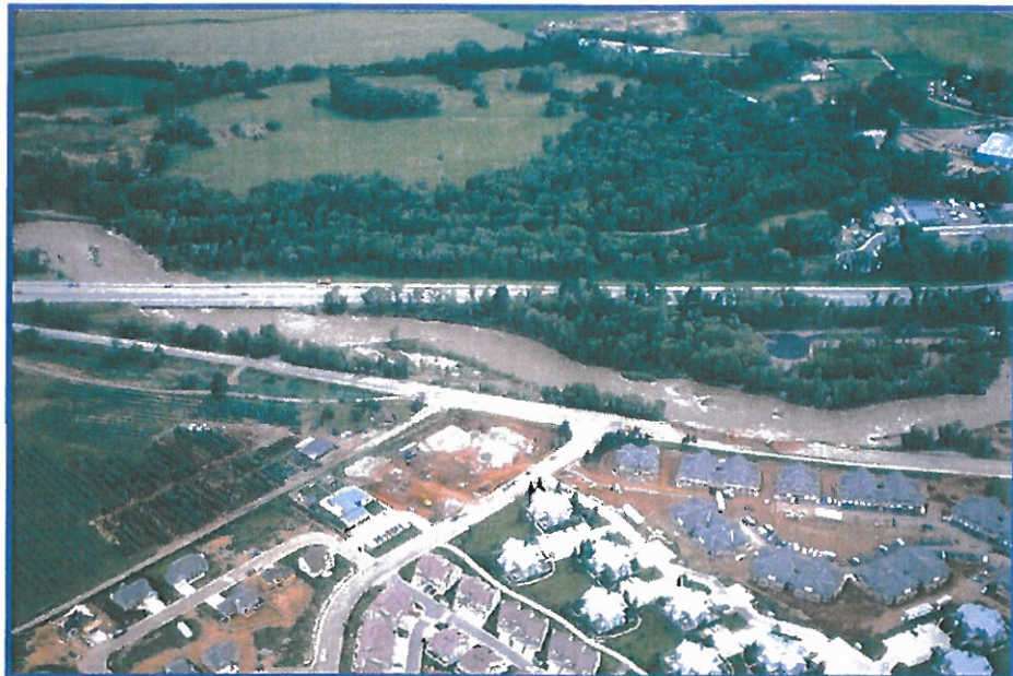
Photo 1: Aerial View of River Park Area during 1995 Flood
