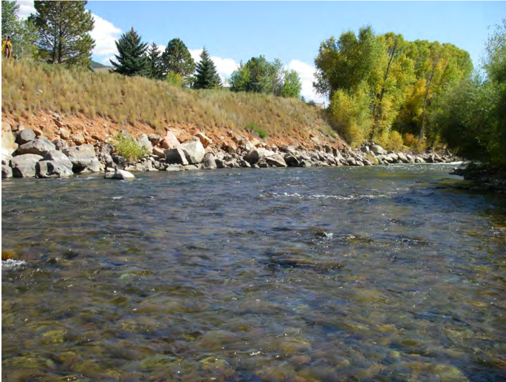
Photo No 1. Existing Denuded Bank
