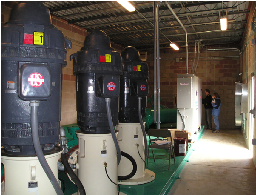
Figure 18. Example pump station that transfers water from an equalizer reservoir
