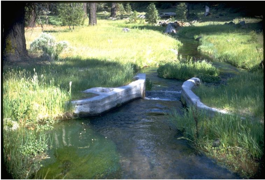
Figure 6. Concrete Parshall flume constructed in field
