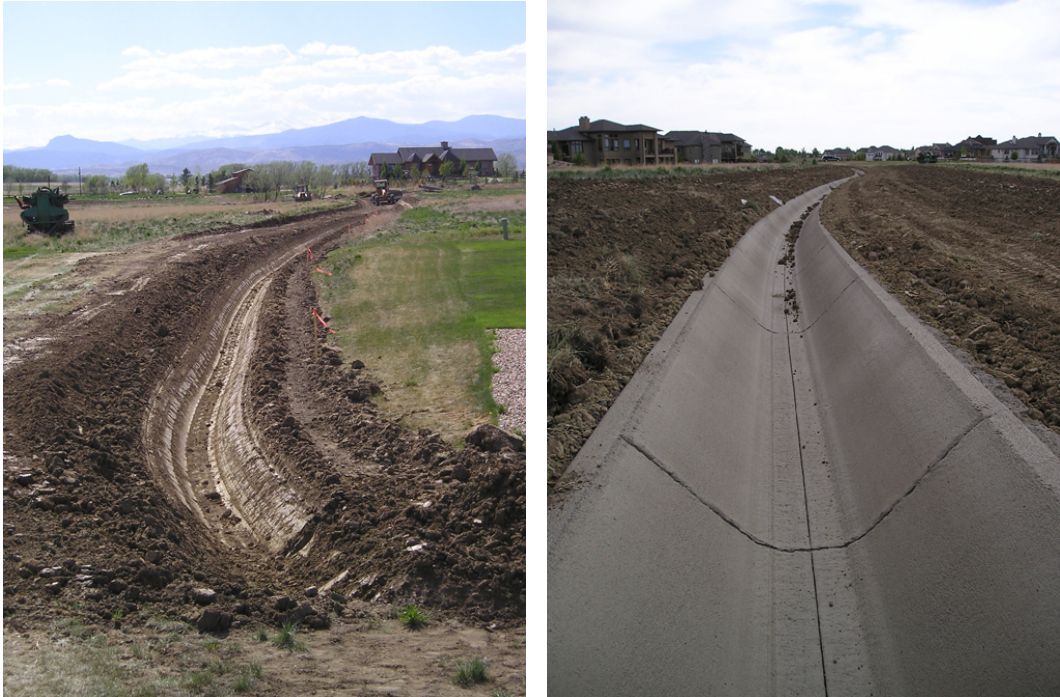
Figure 16. Preparation of site and completed concrete ditch
