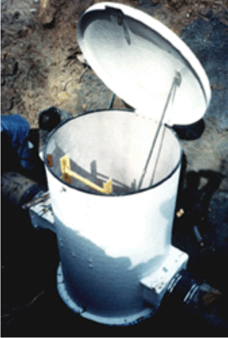
Figure 12. TRACOM Packaged Metering Manhole with a Palmer-Bowlus flume
