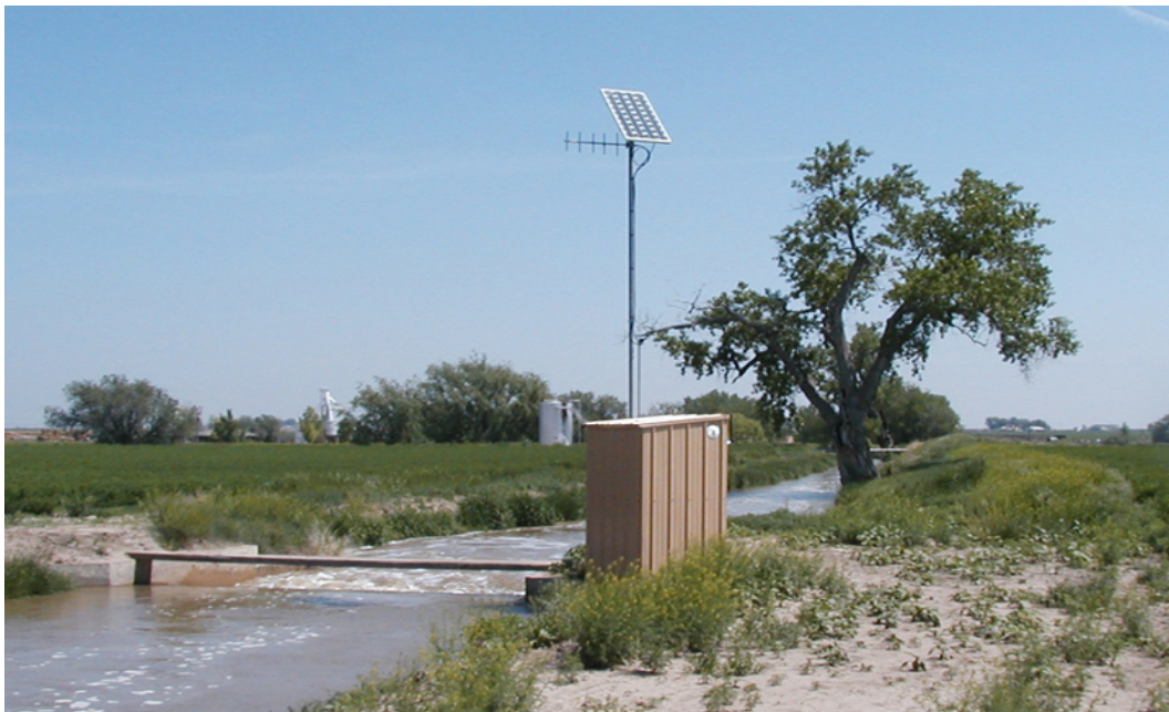
Figure 19. Example of a remotely monitored rated section using a SCADA system. Equipment is 12-volt DC powered from a solar panel that maintains a charge on a battery. Communication with the site is via radio.
