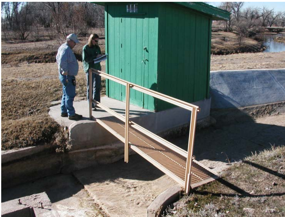
Figure 14. Rated section measurement structure for the Evans Ditch
