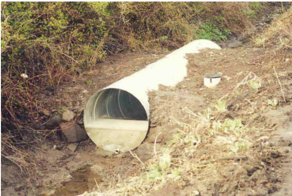
Figure 10. Long-throated flume installed in a pipe section, with stilling well included for measurement capabilities
