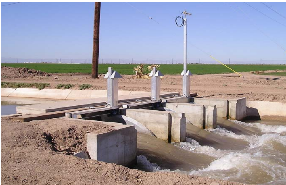
Figure 3. Rubicon gate installation with SCADA
