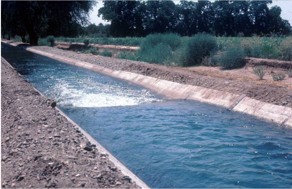
Figure 9. Long-throated flume in operation
