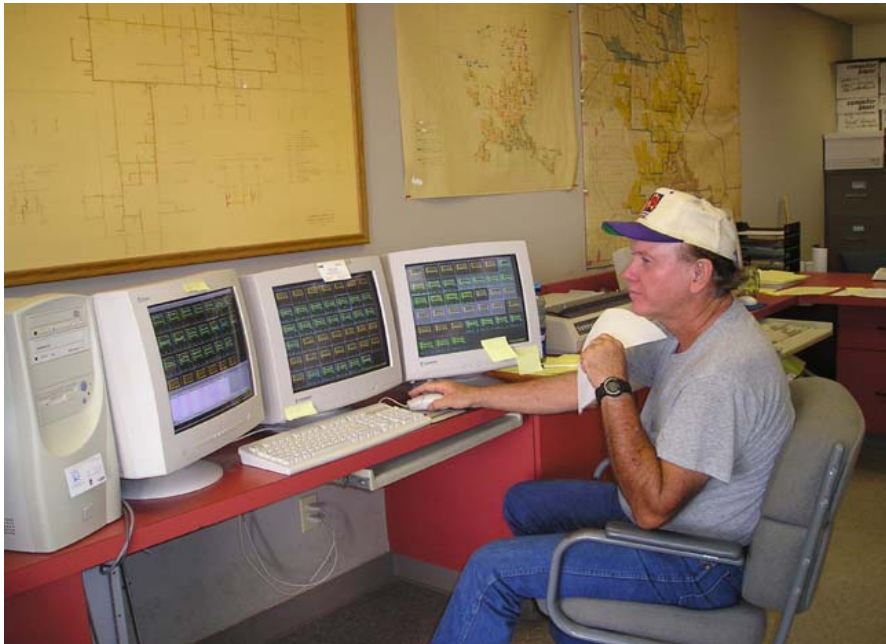
Figure 20. An operator at the Central Arizona Irrigation and Drainage District near Phoenix monitors primary flows and water surface elevations in the 60 mile canal. This SCADA system was implemented at very low cost using affordable RTU equipment and spread spectrum radios for communication.
