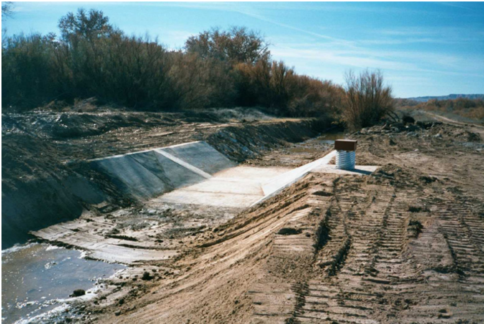
Figure 8. Long-throated flume under construction
