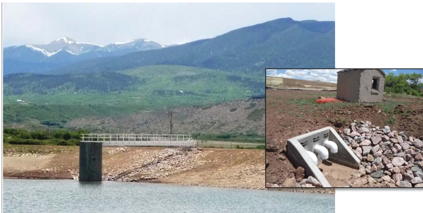
Finished project photos of the North Lake Dam outlet works and toe drain system.
