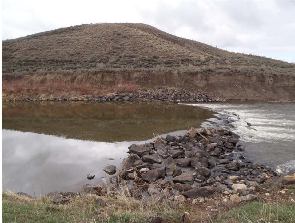
Figure 8 Check structure below McElroy No. 2 Ditch. Structure creates hydraulic hazard for boaters and swimmers. Also exacerbates erosion on banks because it is curved incorrectly. Center of structure should be upstream of wings to relieve stress on banks, provide boat and fish passage, and eliminate dangerous hydraulics.
