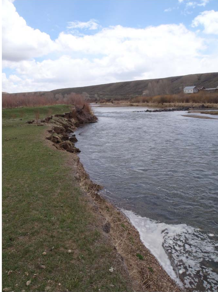
Figure 12 Bank instability at Orr Pump No. 1. Improperly constructed drop structure directs stresses towards bank. May also cause formation of gravel bar on right of the photo which may place additional stresses on the bank.
